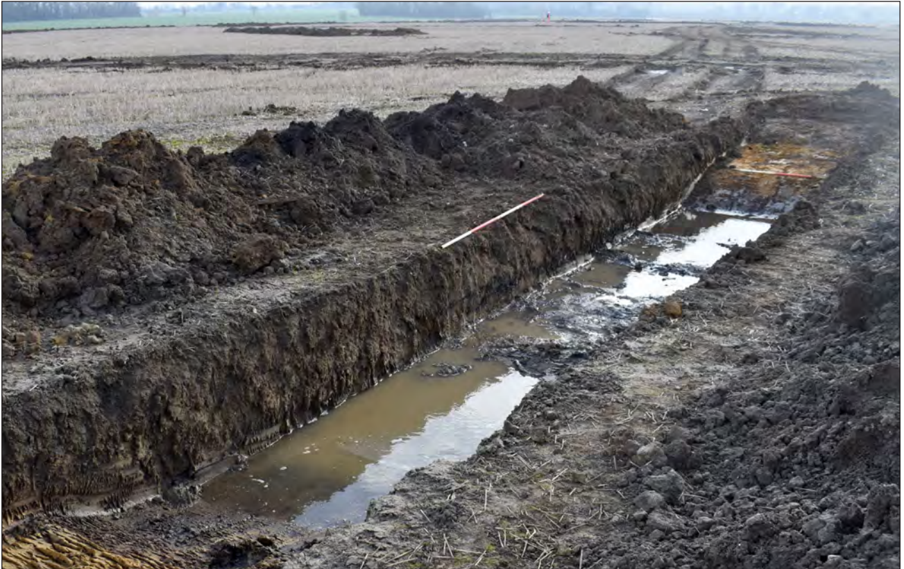
Plate 1: Trench 12 pond 227 looking east
