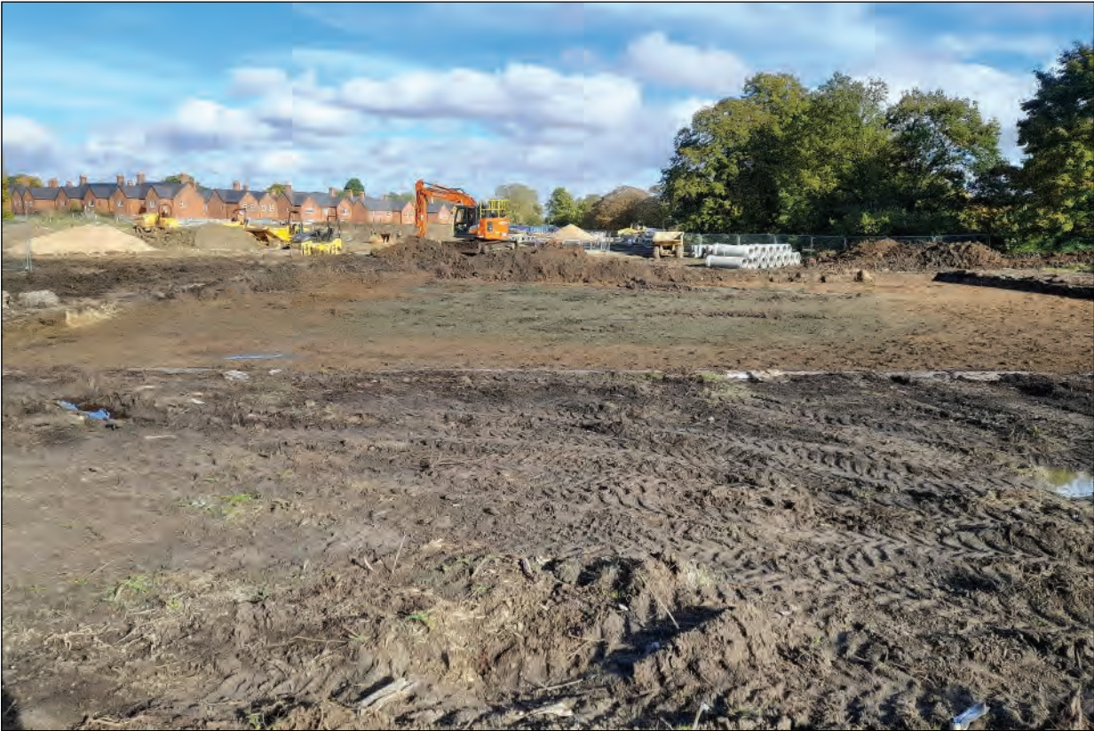
Plate 1: Overview of the tennis court area
