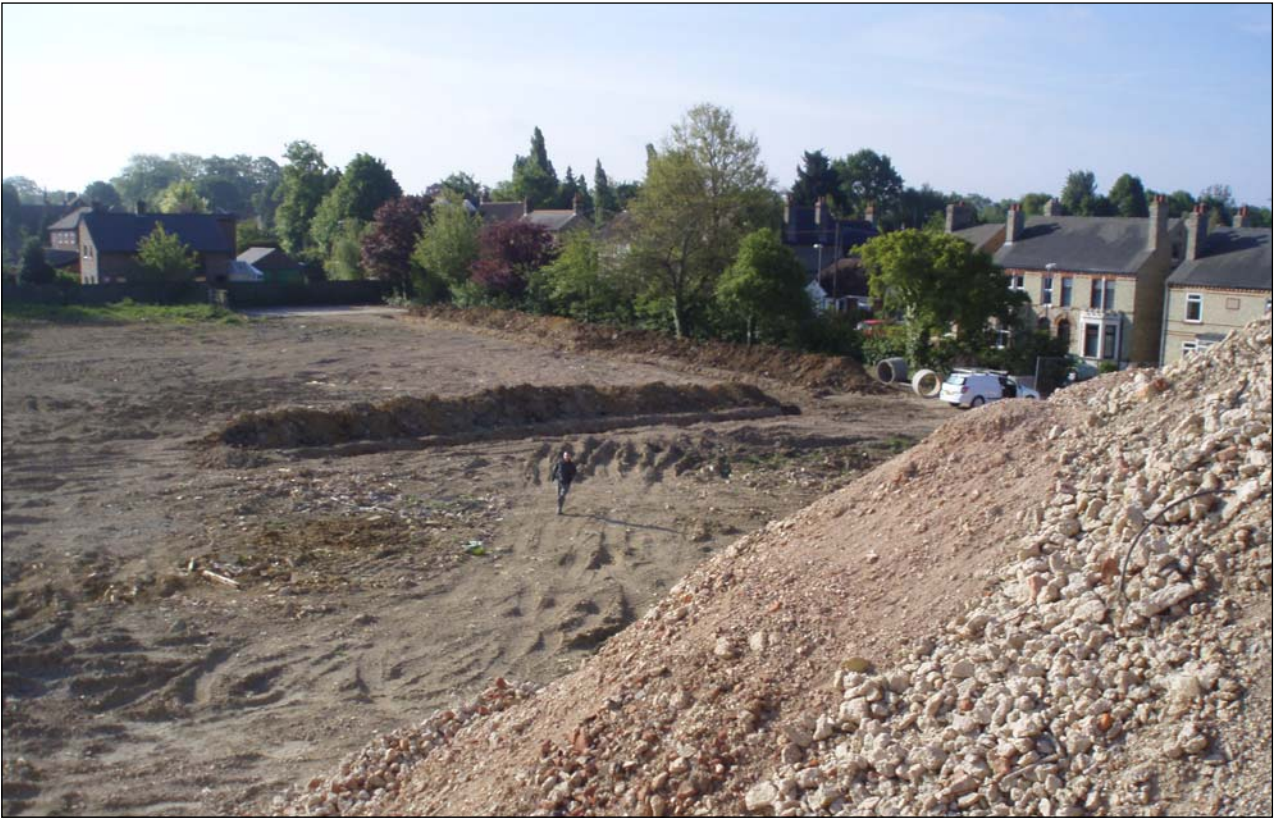
Plate 3: Trenches 5 and 6 from northwest, taken from spoil heap
