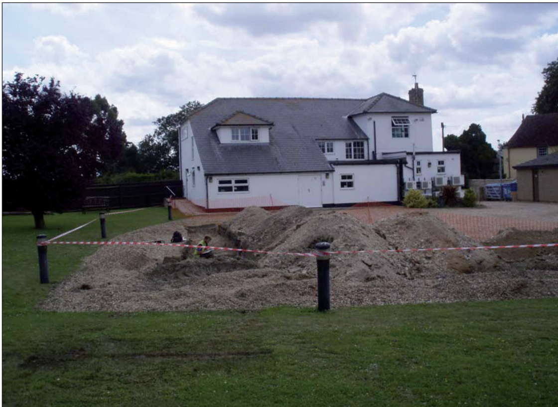
Plate 2: Existing structure and trench 1
