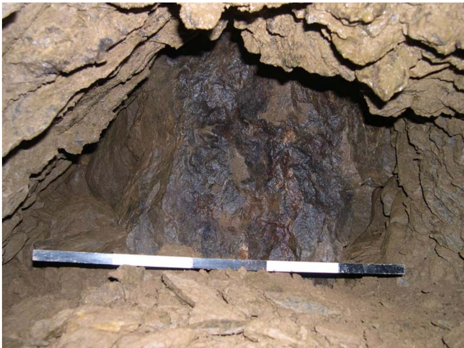
Figure 21: stone blocking (20 th century?) at the eastern end of the 'creep' passage (approximately 4m from the open hole)
