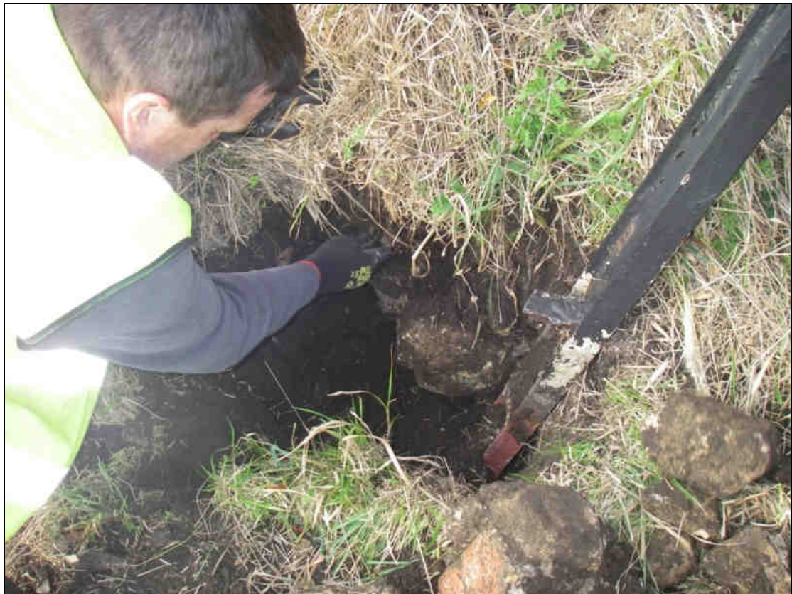
Plate 4. Stones from a collapsed section of the curtain wall, looking north
