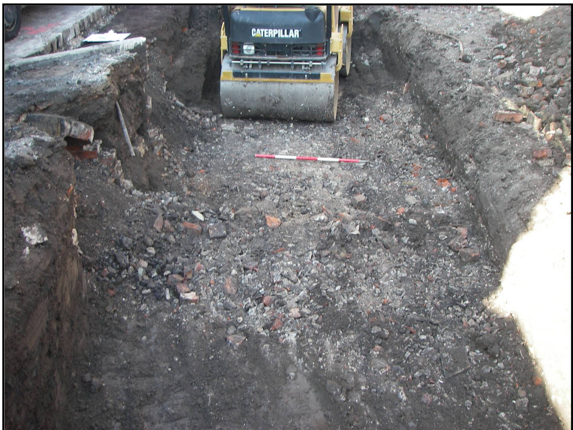
Plate 2: Backfill 1007 of westernmost cellar prior to rolling, view west
