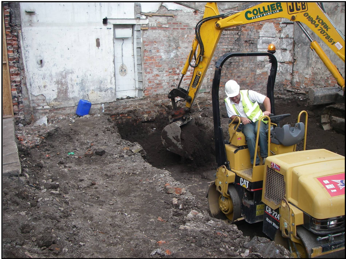
Plate 1: The groundworks, view north-west
