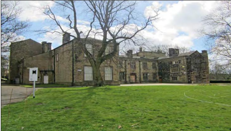
Plate 1. View of survey area and Bolling Hall, looking south
