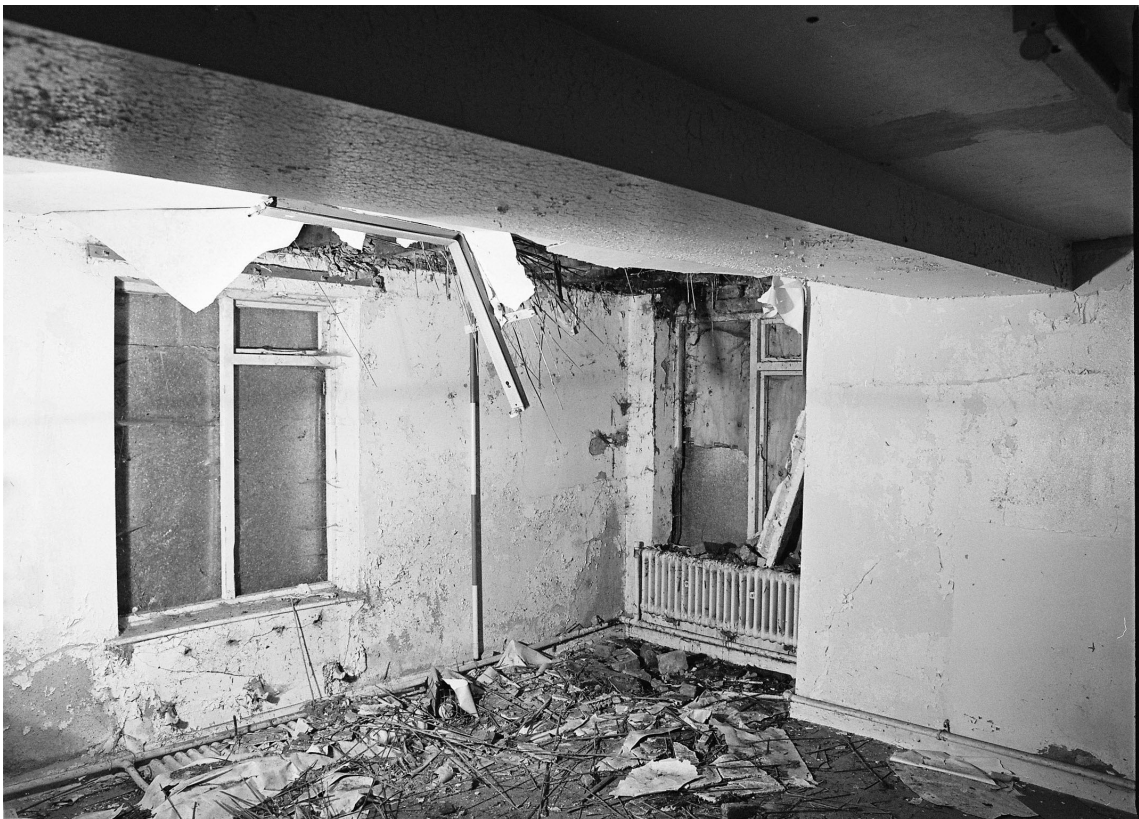
Photograph 44 Film 3_008 Direction SW
