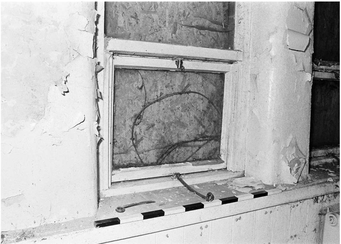
Photograph 32 Film 1_007 Direction SW
