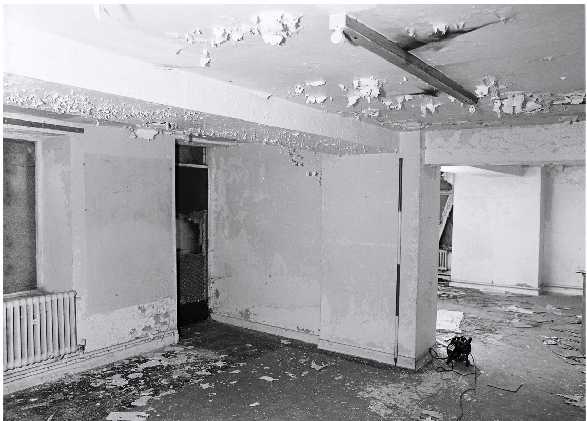
Photograph 42 Film 3_006 Direction SW
