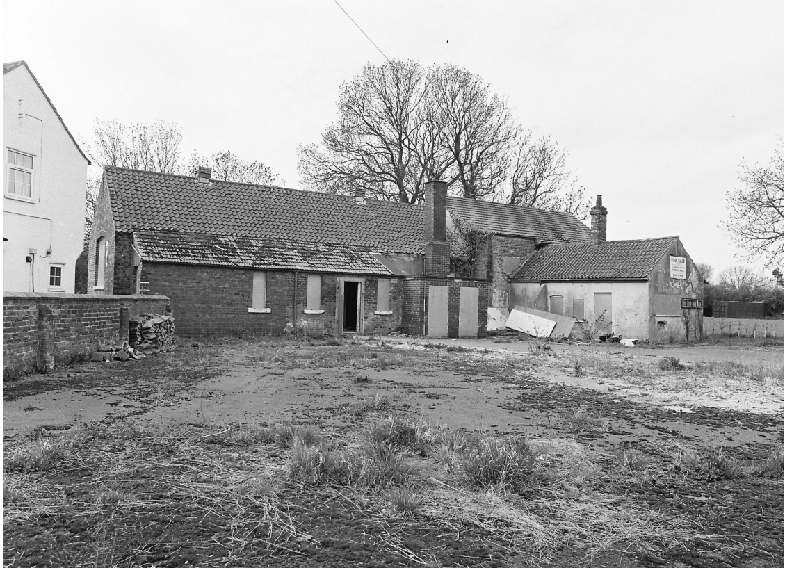
Photograph 1 Film 4_002 Direction SW
