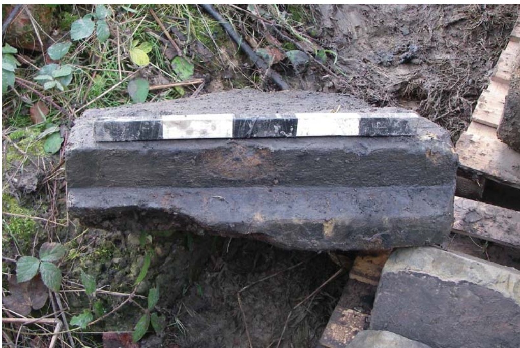
Plate 11. Cornice with dressed and chamfered faces (Cat. No. 8)
