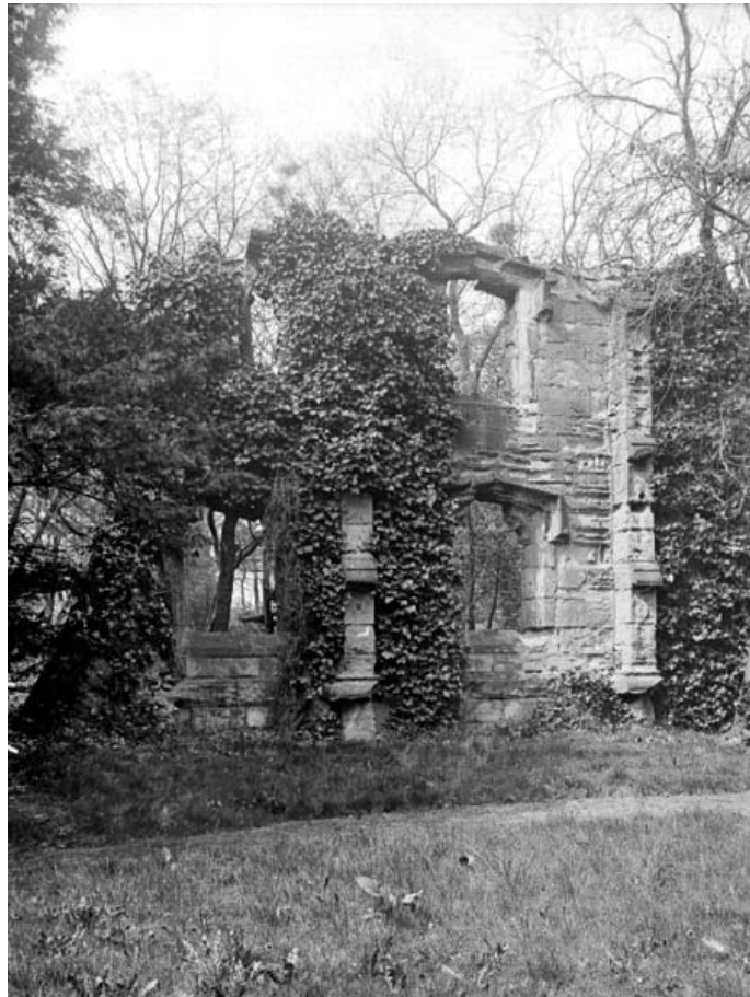
Plate 16. Stone-built phase of the Hall, with moulded window tracery, hood mould and reveals. The moulded stonework could be a match to some of the recorded stone work (see Cat. Nos 2, 3 and 11)
