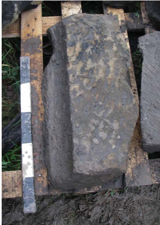
Plate 6. Hood mould with hollow chamfer (Cat. No. 3)
