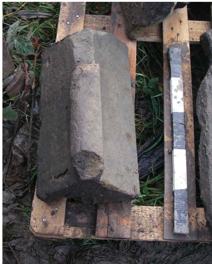
Plate 4. Coping stone with roll apex (Cat. No. 1)
