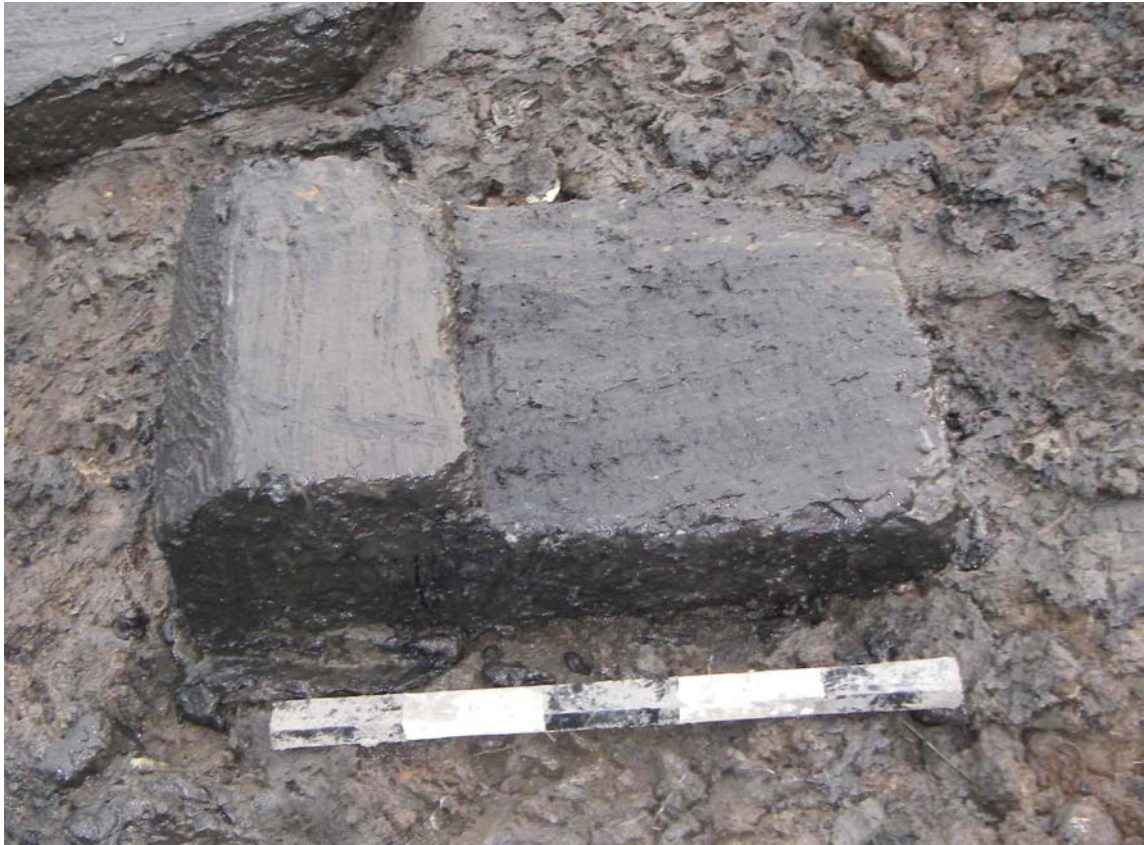
Plate 15. Chamfered and splayed door jamb (Cat. No. 12)
