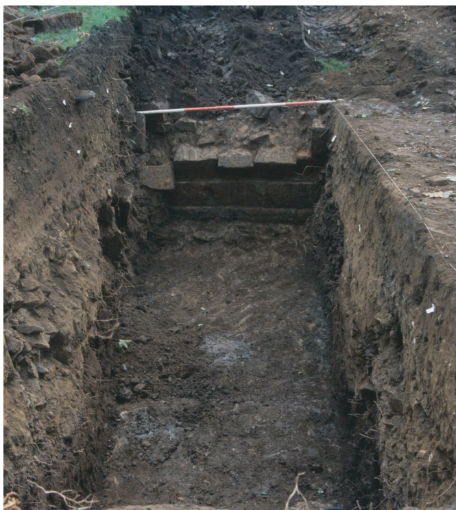
Plate 1. Trench 3, view of moat retaining wall (1116) in machine excavated sondage, looking south-east
