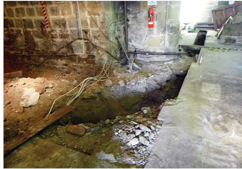
Plate 2. Completed drainage trench across the nave, looking north
