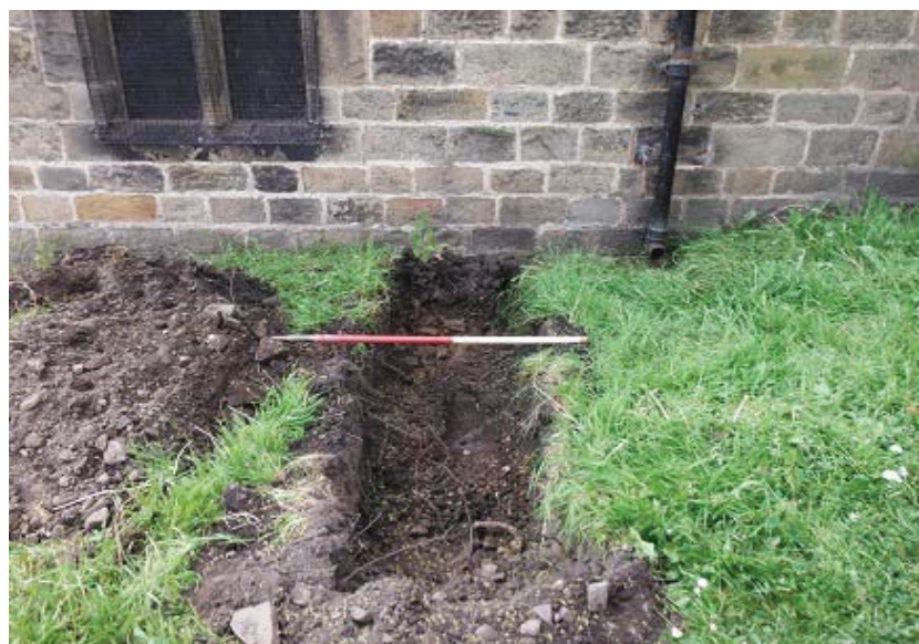
Plate 4. Excavation of topsoil from external drain trench, looking south
