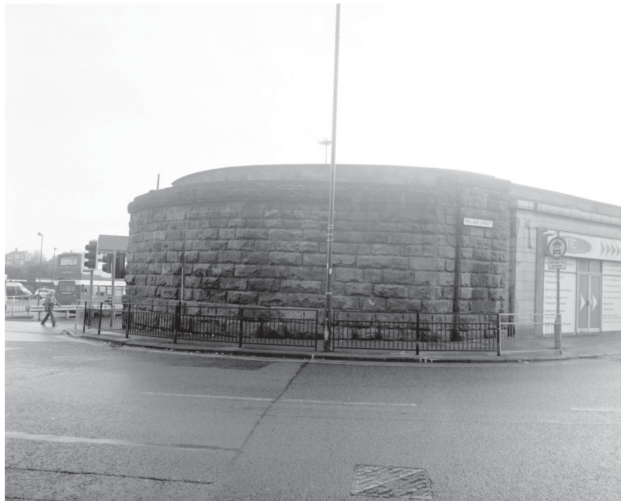
4 9716/7 SE Curved north elevation of additional end wall
