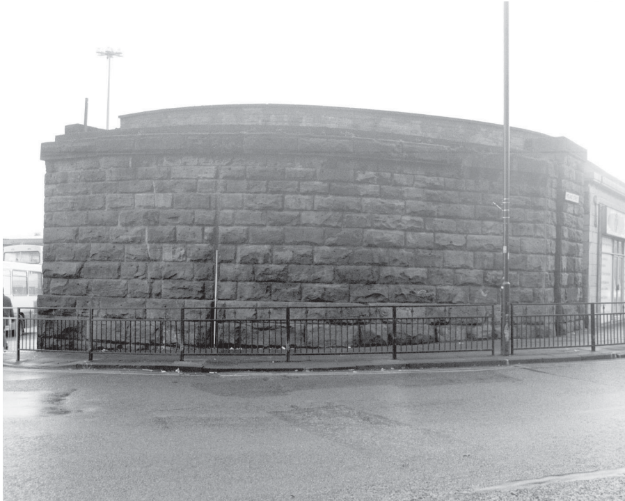
5 9716/10 SE Detail of north curved elevation of additional wall
