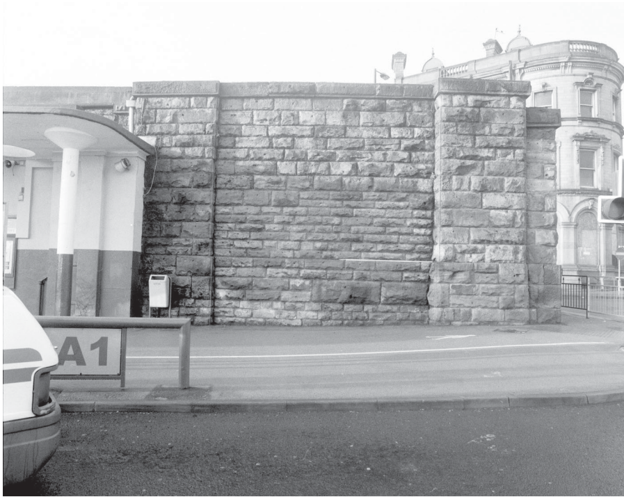
1 9716/4 SW North-west facing elevation with buttresses
