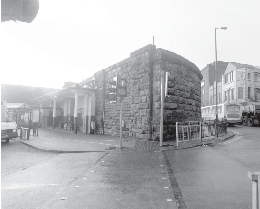
3 9716/6 S North end of viaduct with rock faced re-built addition
