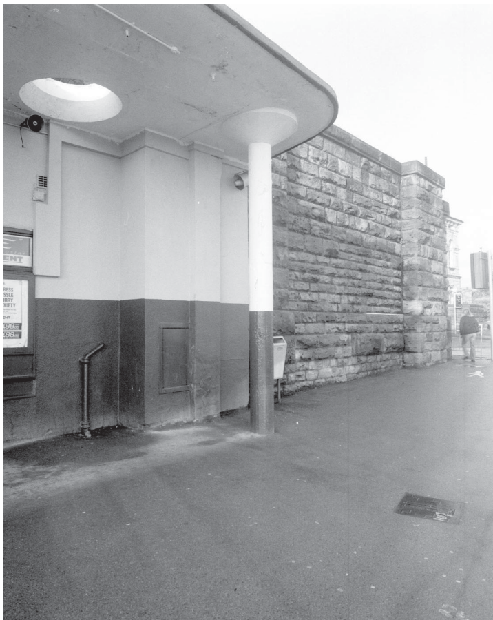
2 9716/5 NW North-west facing elevation with modern concrete shelter obscuring detail
