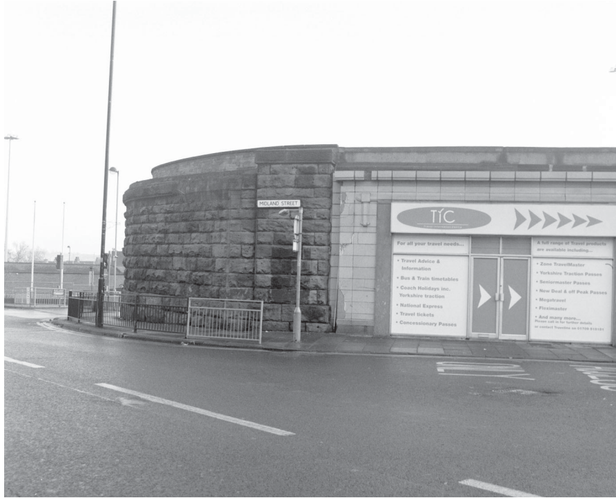
7 9716/12 E North end of viaduct showing buttress
