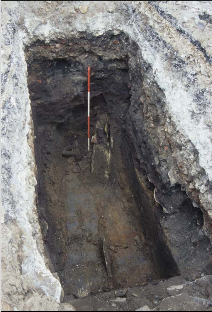
Pl. 11. Stone culvert 254 in Trench 18 from the west
