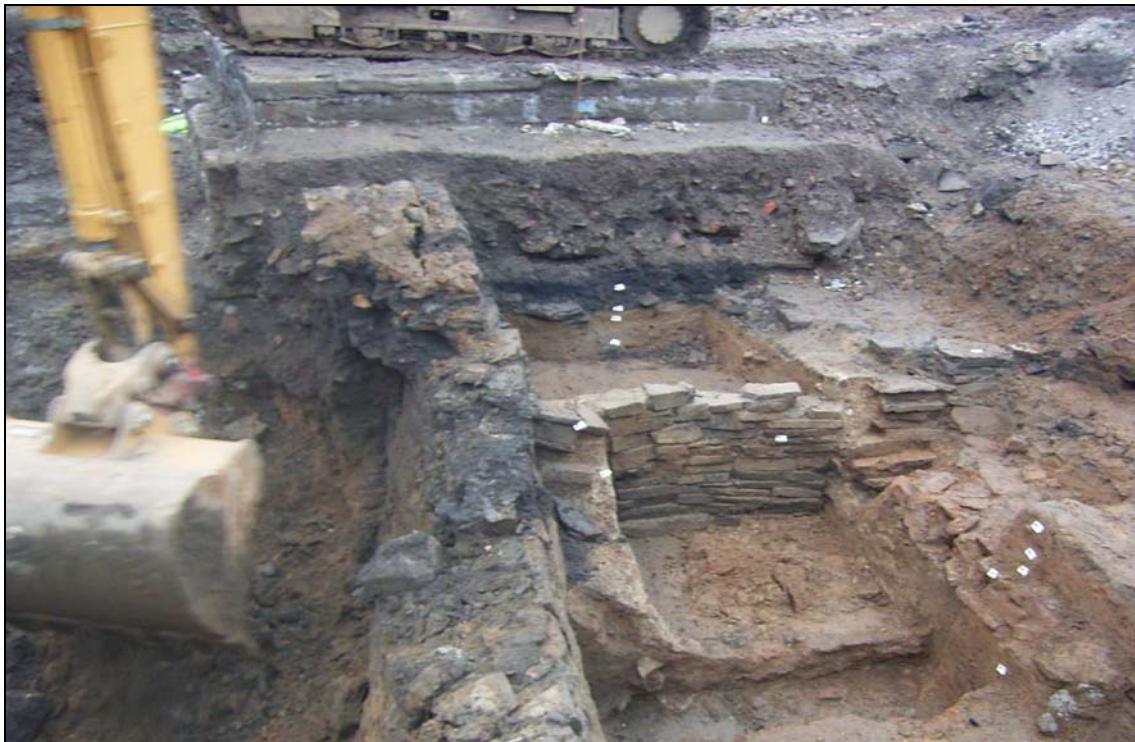
Pl. 42. Working shot from west showing Phase I wall 1321 exposed beneath wall 1040
