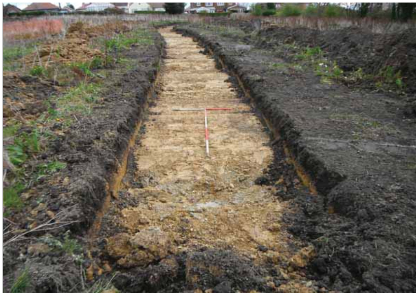
Plate 3. General view of Trench 5, looking west
