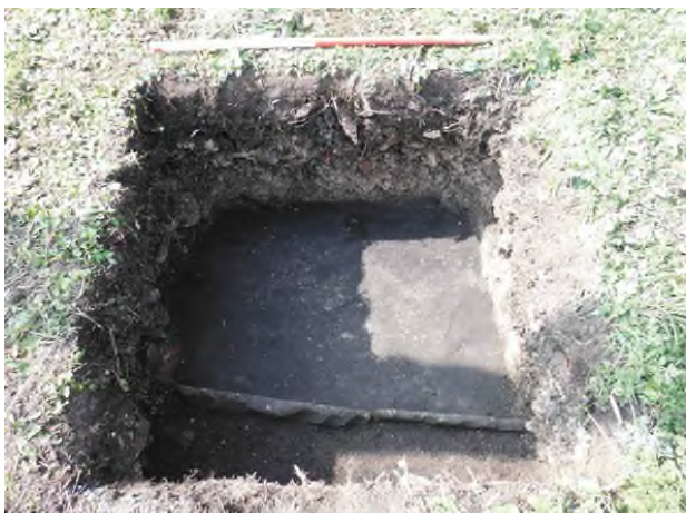
Plate 18. TP4, looking west with path 402 and kerb stones 403
