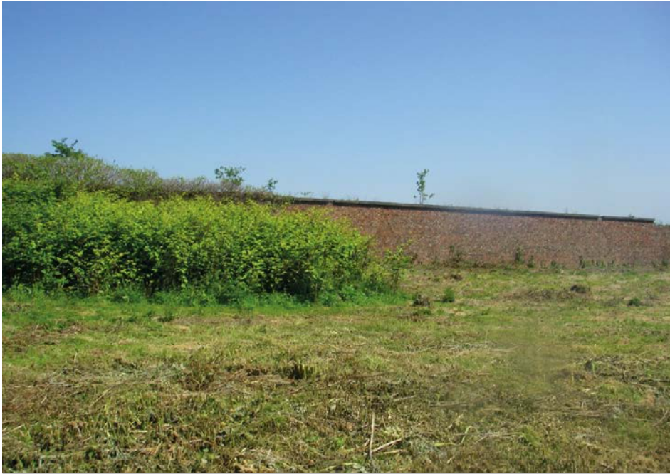
Plate 1. General view of site, looking north
