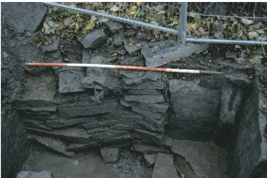
Plate 14. Detail of south-east wall (206, 205) of waterhole 209, with dry stone and inverted slab construction, looking south-east
