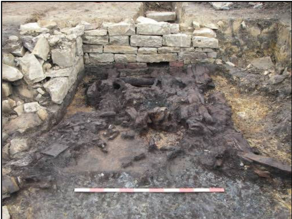
Plate 2: Area A/D. Northern wall of stone tank (009), mouth of culvert (010) and waterlogged timbers (2134)
