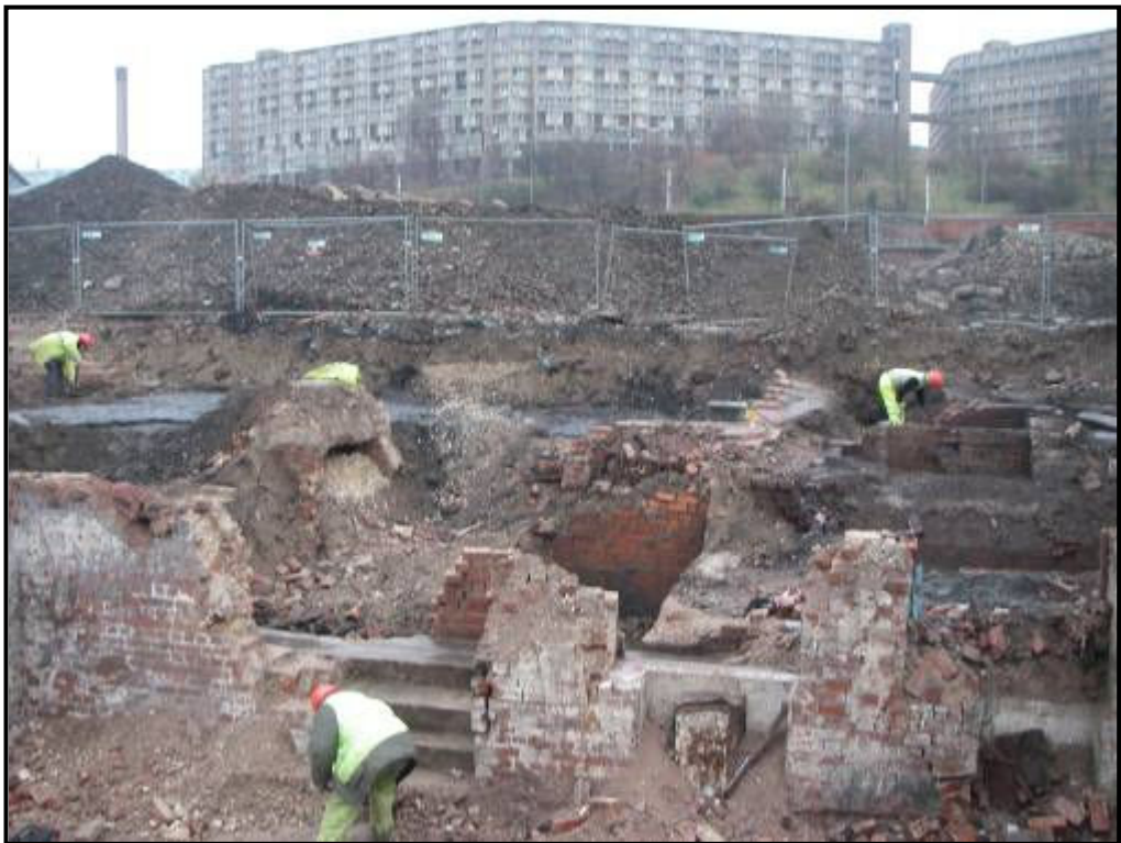
Plate 16. Area E. Excavation of the Sheaf Island Works basements
