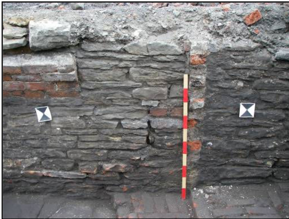
Plate 10: Area A/D. West facing wall of cellar 14, showing the bottom four courses of a brick vaulted ceiling to the left and the scar of the dividing wall between cellars 14 and 15 by the scale
