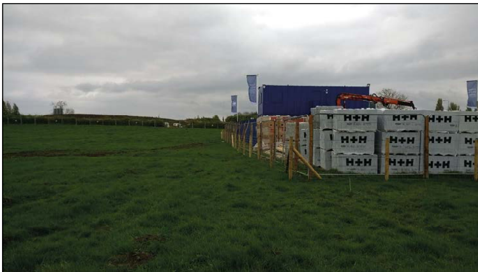
Plate 3. General view of site, looking south
