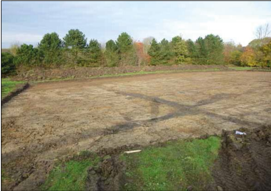
Plate 1. Shot of excavation area after topsoil strip; facing northwest
