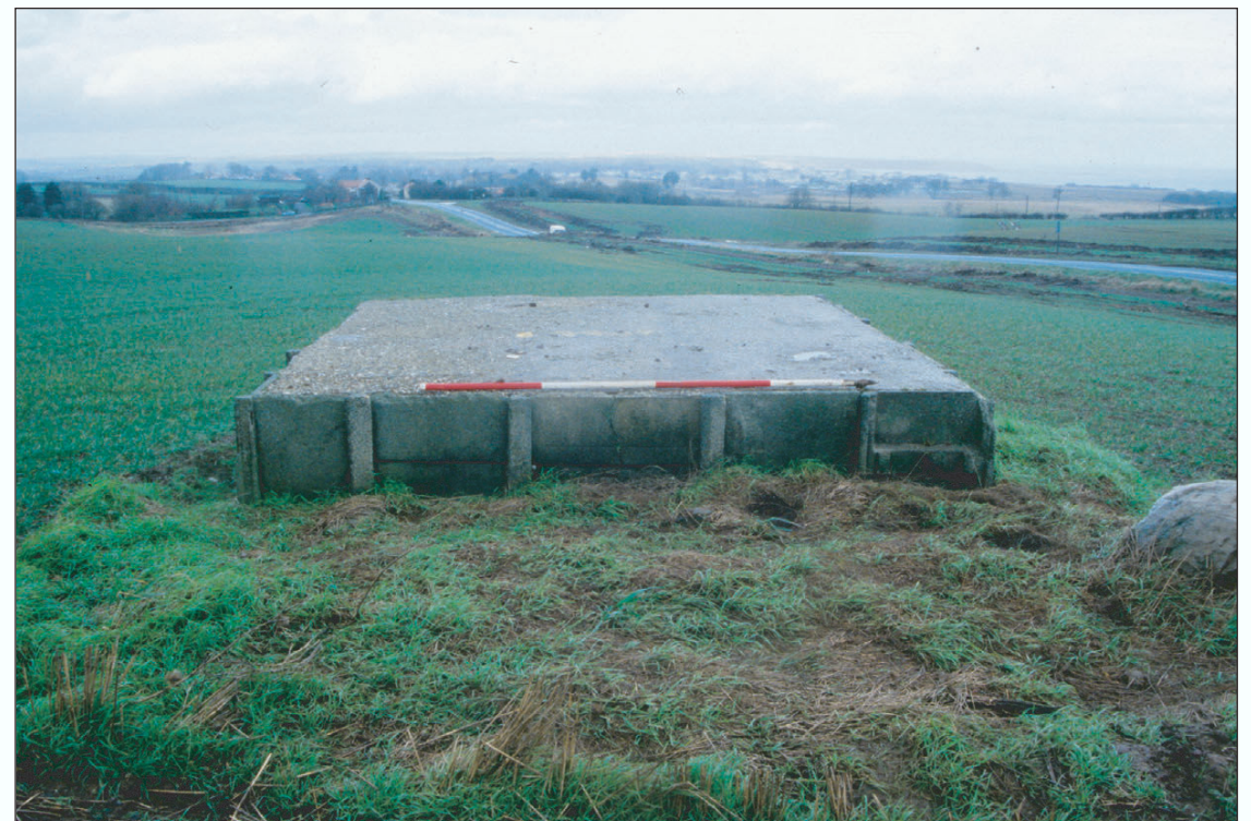
Plate 16. Pill box 2, looking north northwest (Area E)
