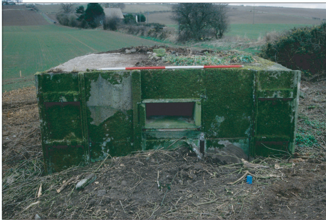
Plate 13. Pill box 1, looking south southwest (Area E)
