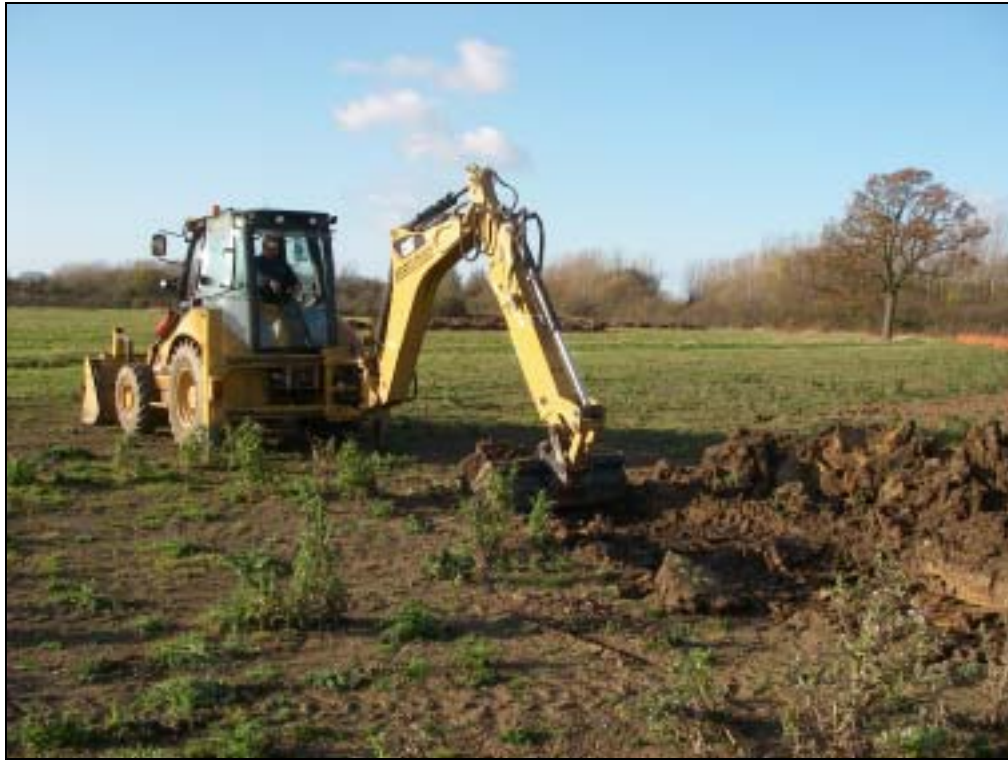
Plate 1. Excavation of Trench J, looking northwest
