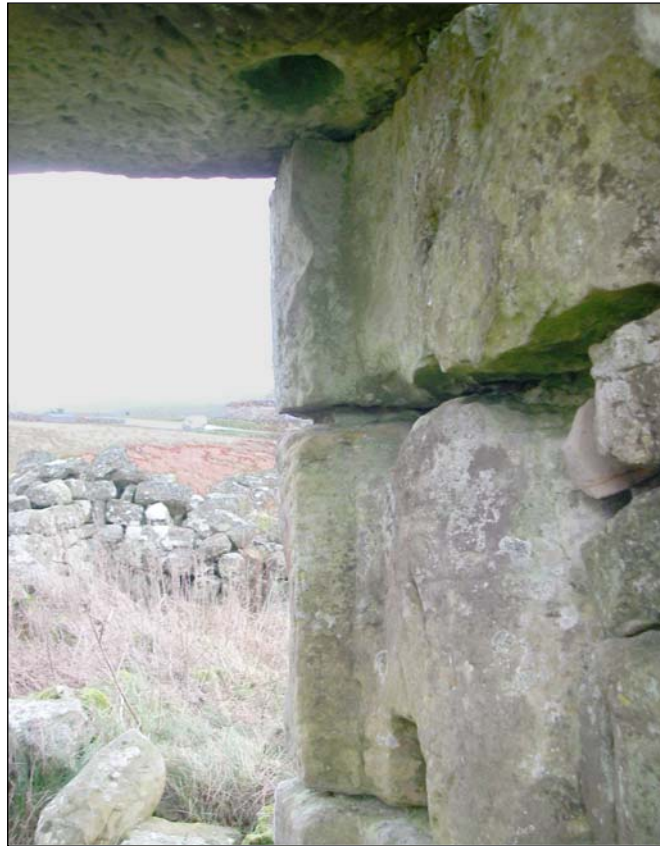
Plate 9. The interior of the southern wall of the bastle doorway with the circular depression of the harr-socket on the lintel, and the hole for the drawbar to the bottom right
