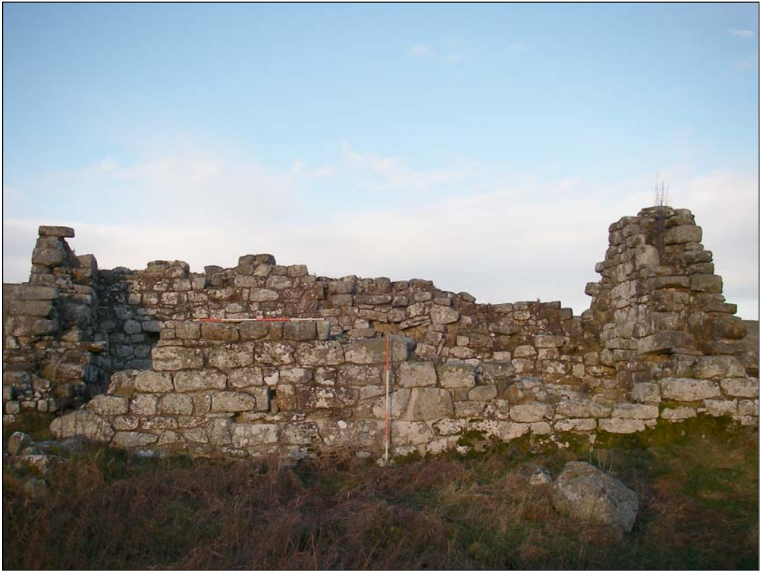
Plate 7. The southern wall of Ironhouse Bastle, looking north
