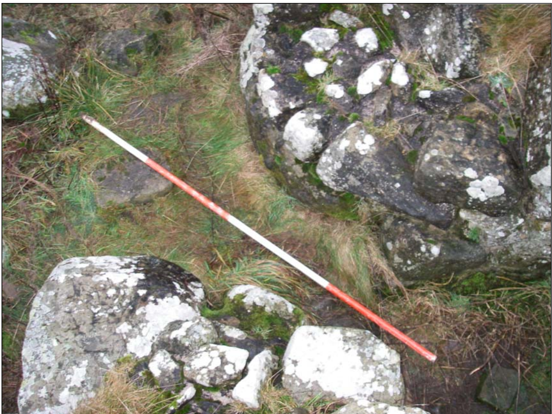
Plate 14. The break in the south-western corner of the bastle wall
