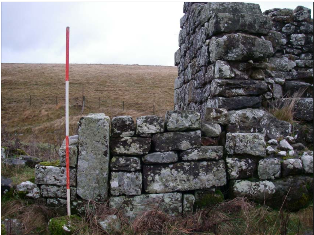
Plate 18. The blocked doorway in the southern wall of House 1, looking north
