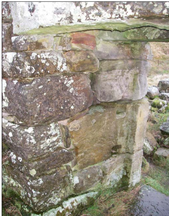
Plate 10. The interior of the northern wall of the bastle doorway, showing the tunnel for the drawbar, and below, the hole for the opposing drawbar, together with latch indentations
