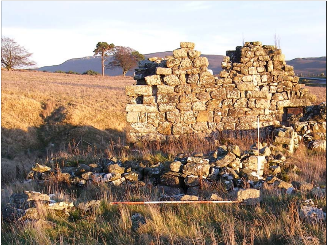
Plate 17. The remains of House 1, adjacent to the western end of Ironhouse Bastle, looking east
