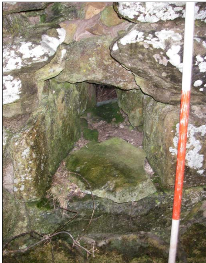
Plate 12. The interior of the slit-vent in the western gable-end wall of the bastle
