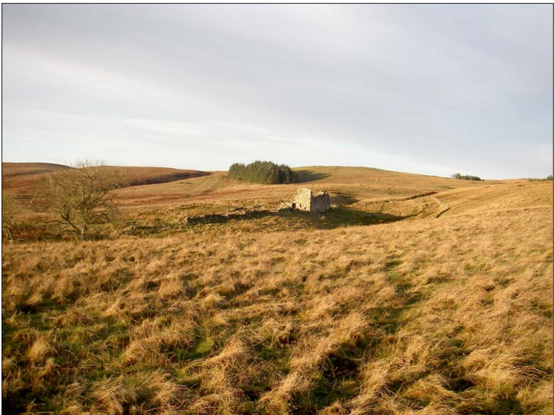
Plate 2. Ironhouse Bastle with the eastern range of buildings to the left, looking south-west
