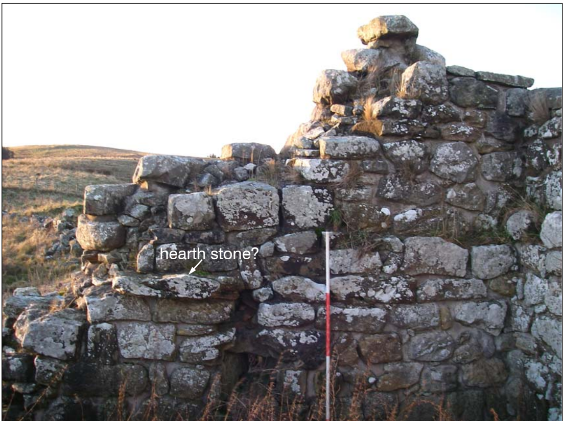
Plate 16. The interior of the western gable-end of the bastle. A projecting stone to the left may have supported a hearth, and a recess to the top right may be the remains of a cupboard space. There is a slit-vent at the centre of the base of the wall
