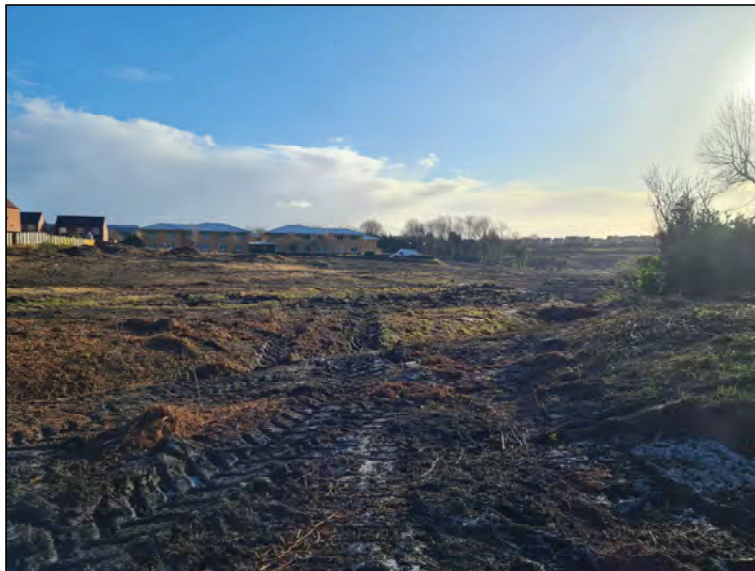
Plate 3. General view of Phase 2b, looking southeast
