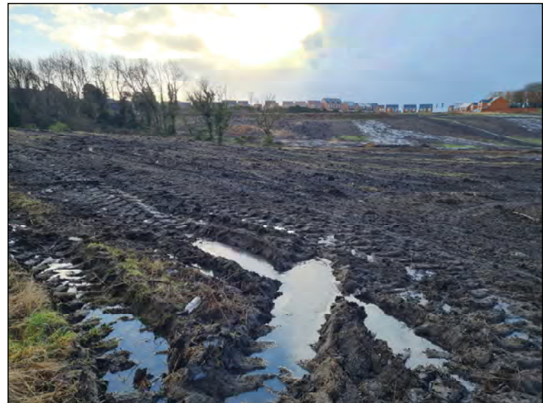
Plate 4. General view of Phase 2b, looking south
