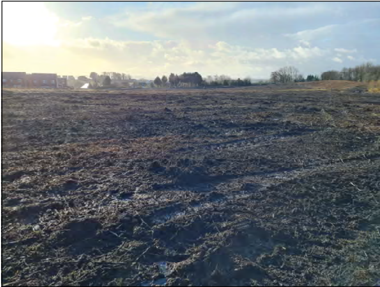
Plate 1. General view of Phase 3, looking south
