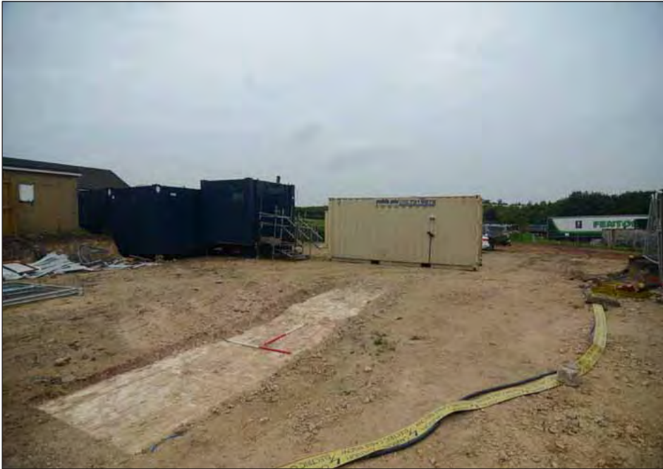
Plate 1. General view of Trench 1A, looking north
