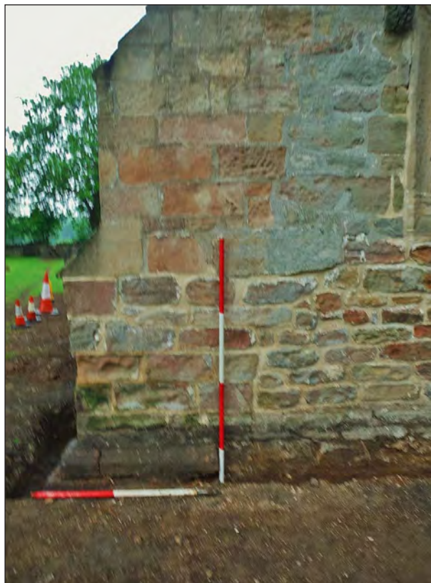
Plate 10. Context 105 and buttress, facing east
