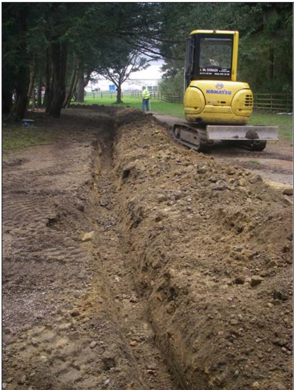
Plate 1. Excavated service trench, looking south-west
