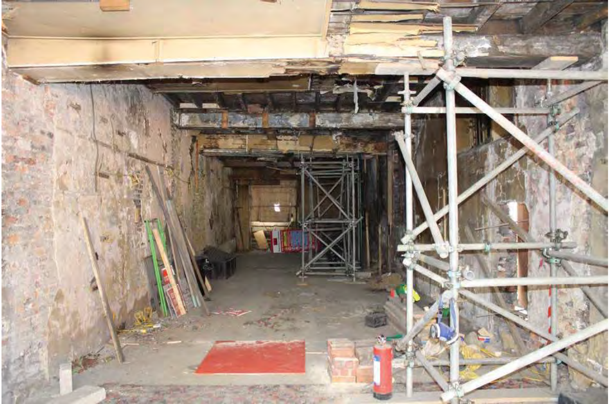
Plate 35 East range, ground floor
