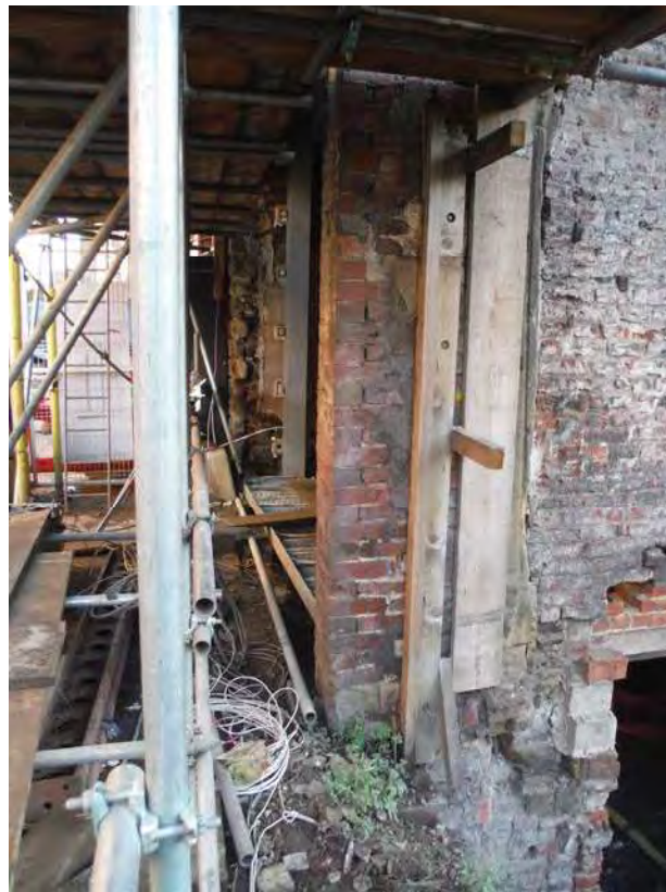
Plate 50 Ground floor level of the north elevation of the east range
