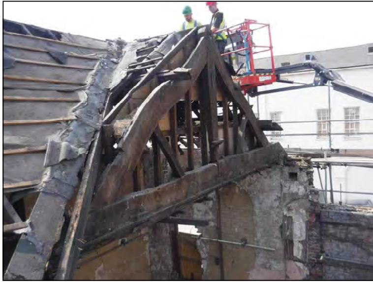
Plate 1. Truss 1, general view, looking south-east
