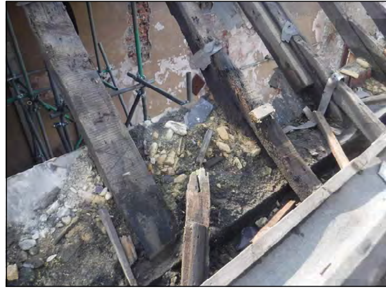
Plate 14. Rafters with carpenter's marks, looking south-east
