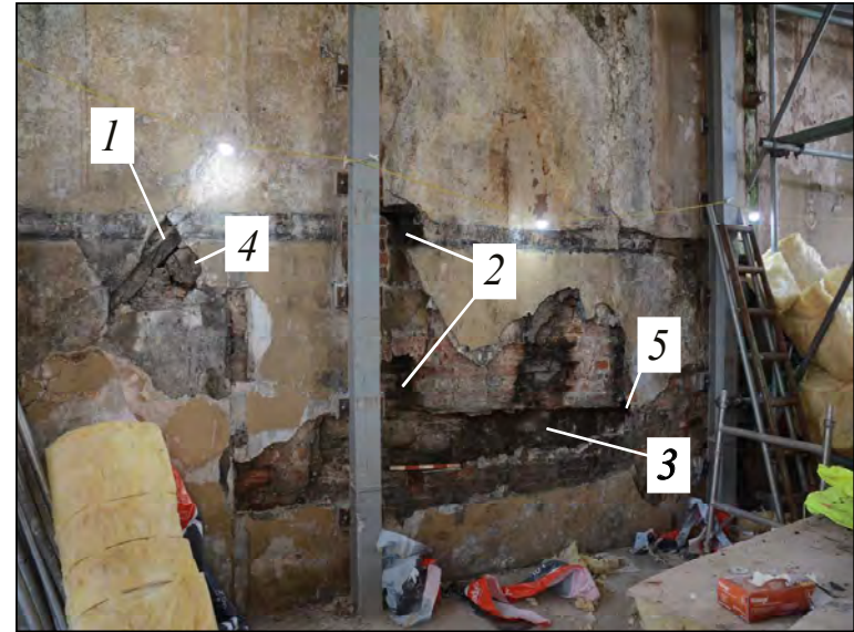
Plate 2. General view of the exposed timbers, looking east
