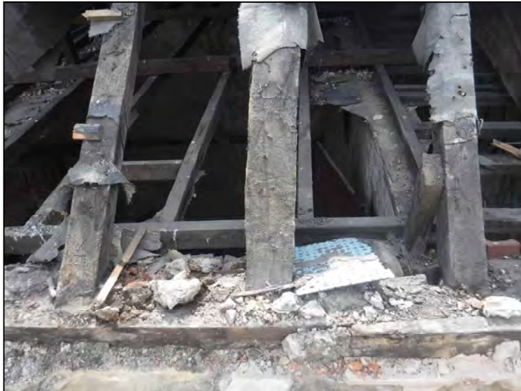
Plate 15. Rafters with carpenter's marks, looking east
