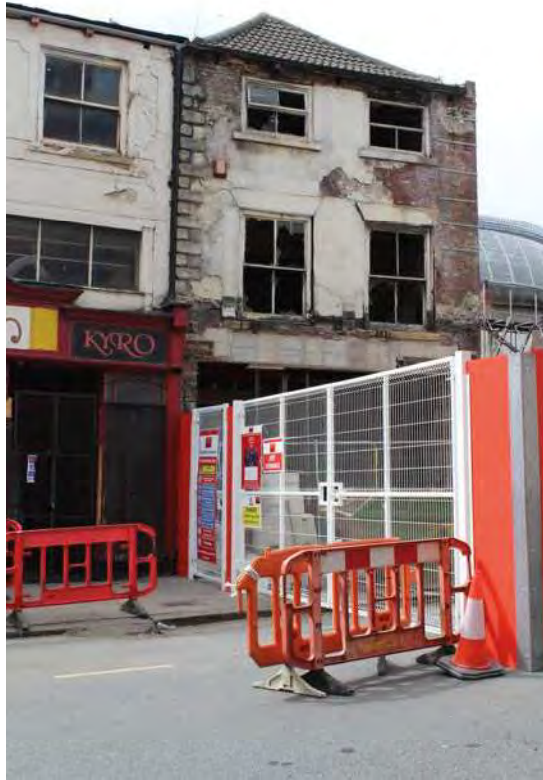
Plate 49 North exterior elevation of the east range
