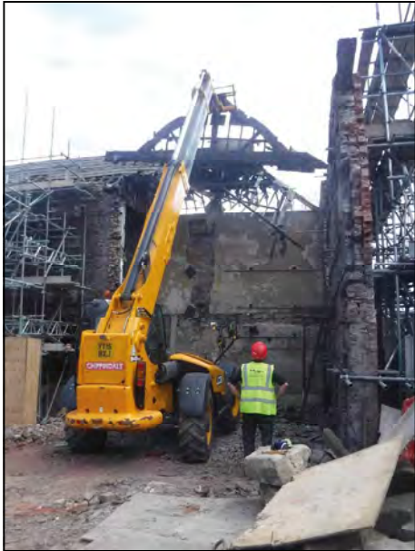
Plate 5. Removal of Truss 1, looking east
