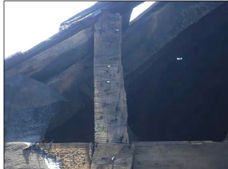
Plate 16. Rafters with carpenter's marks, looking east
