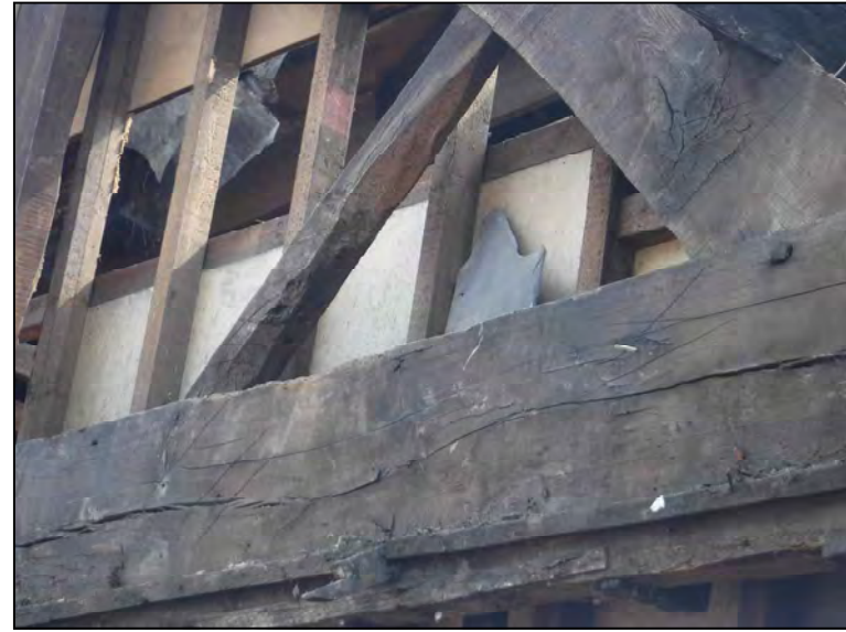
Plate 2. Truss 1, carpenter's marks, looking north-east
