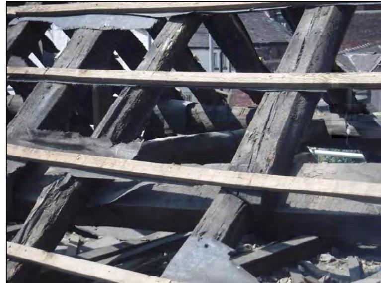
Plate 12. Horizontal beam, between Trusses 3 and 4, looking west
