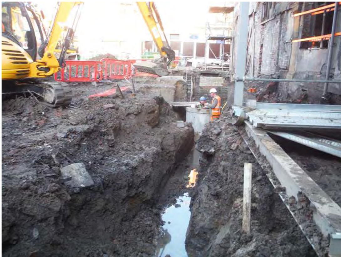
Plate 28 Installation of drain at the north end of the Pipe Trench
