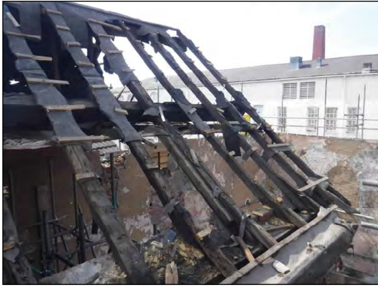
Plate 13. Original and replacement rafters, looking south-east
