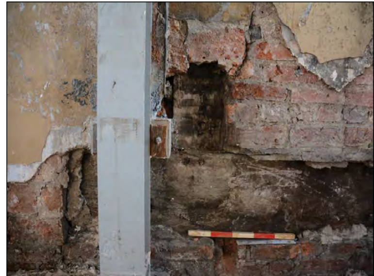
Plate 4. Joint of Timber 2 and 3, looking east
