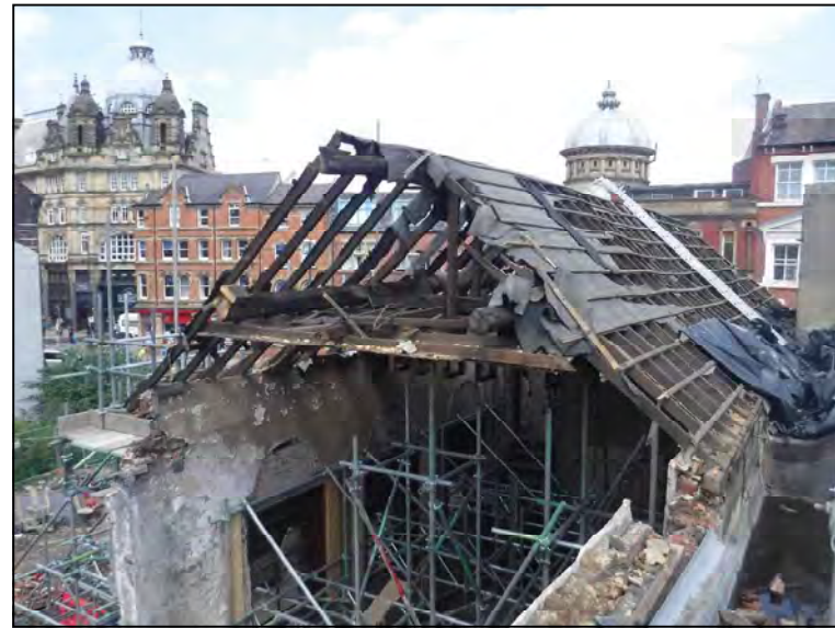
Plate 6. Location of Truss 2, following removal, looking north
