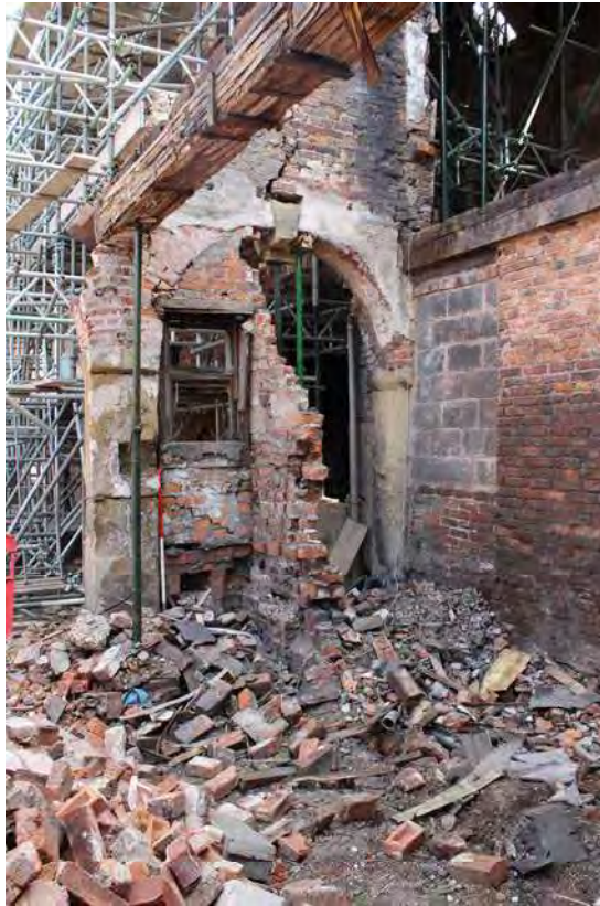
Plate 87 North interior elevation, showing east end arcade arch
