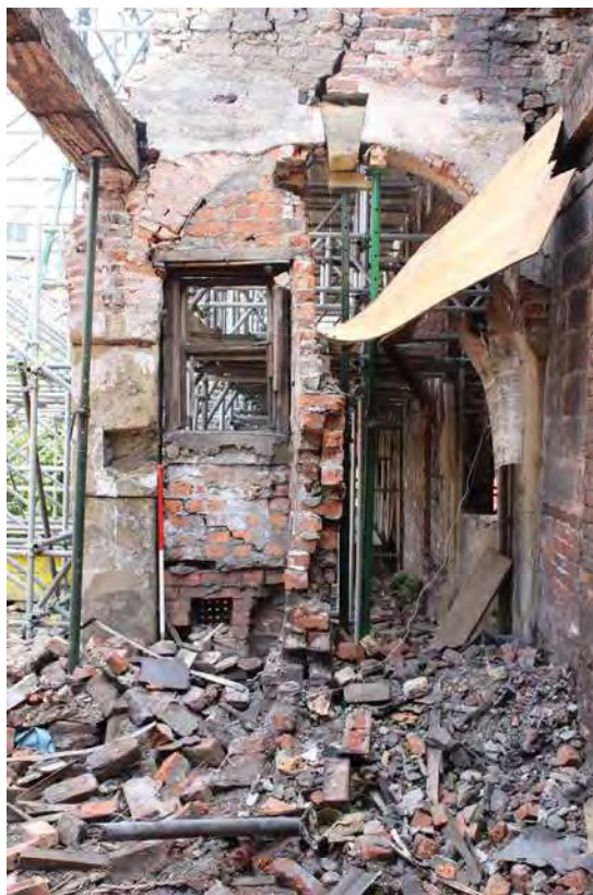
Plate 88 North interior elevation, showing east end arcade arch
