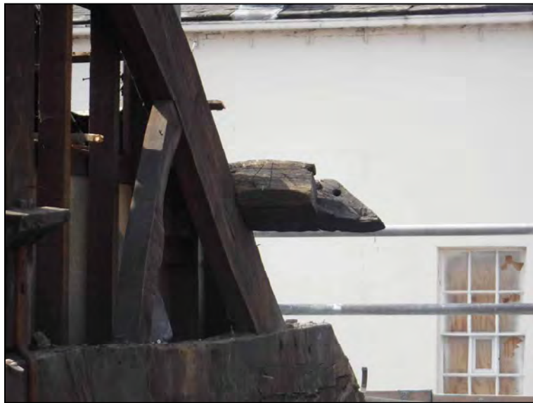
Plate 3. Truss 1, purlin with carpenter's mark, looking south
