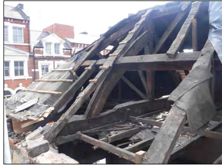
Plate 10. Truss 5, looking north-east
