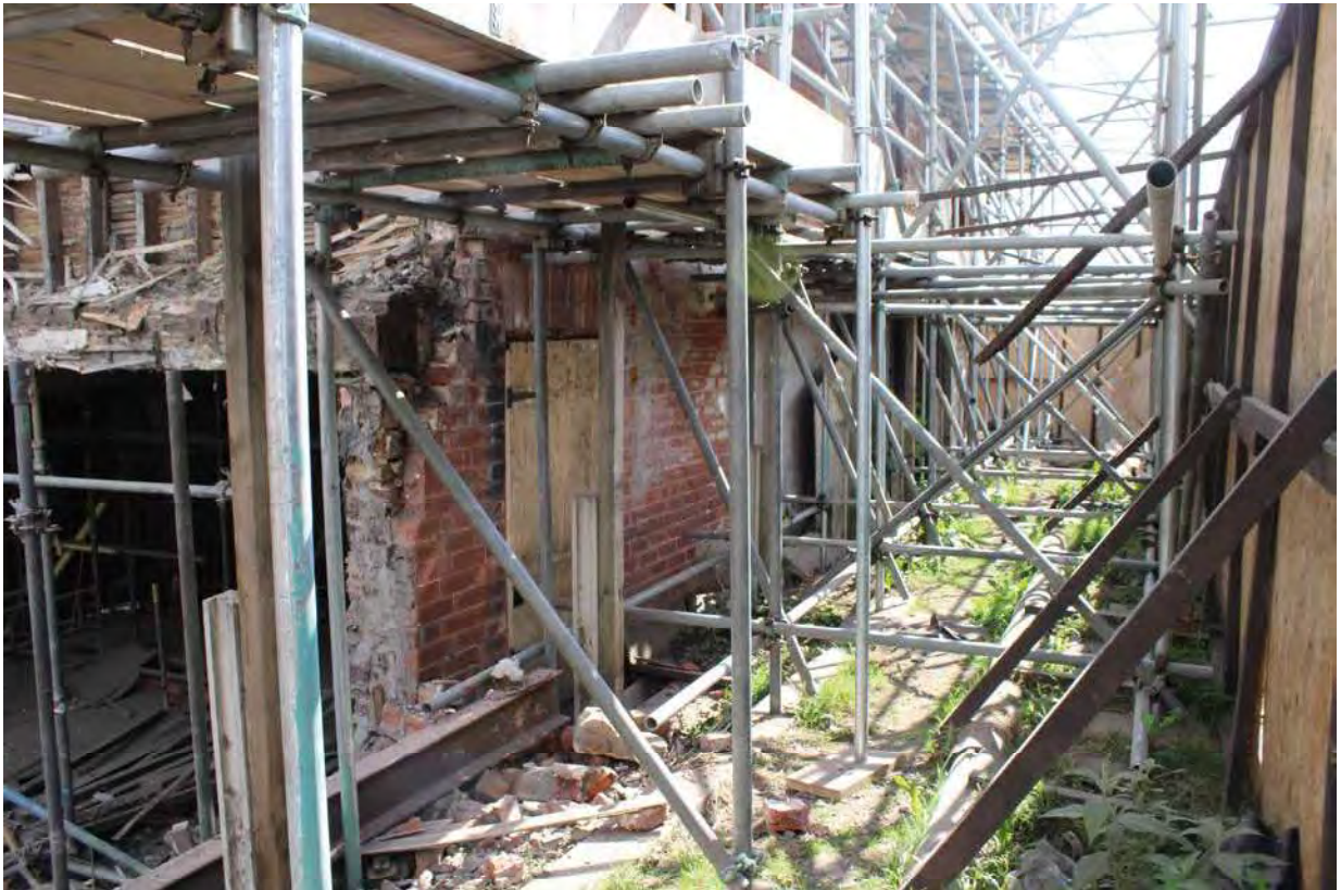
Plate 42 External view of south wall of south range
