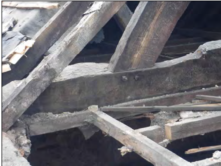
Plate 11. Truss 5 carpenter's marks, looking north-east
