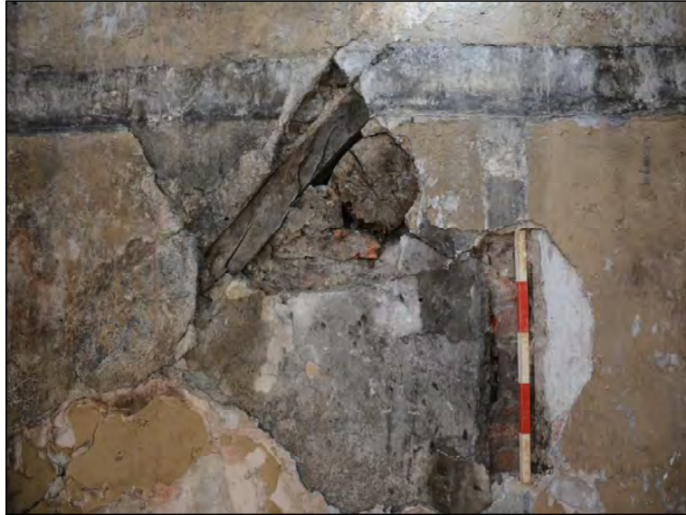
Plate 3. Timbers 1 and 4, looking east
