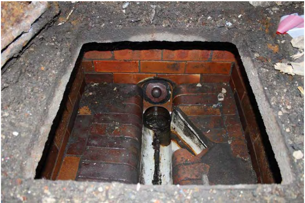
Plate 16 Drain access point in north corner of cellar
