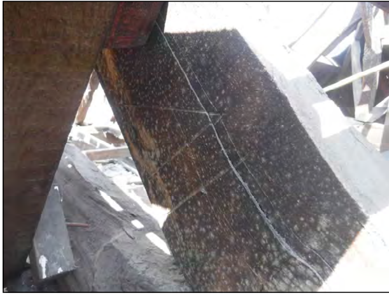
Plate 9. Truss 4 carpenter's mark, looking north-west
