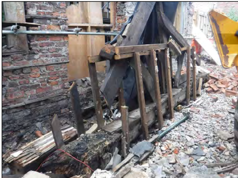
Plate 7. Truss 2 following removal
