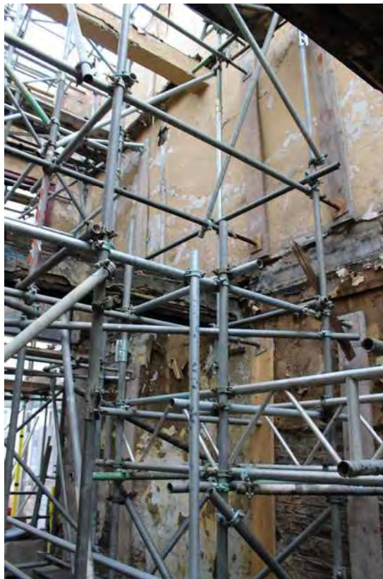
Plate 58 East wall of east range, north end
