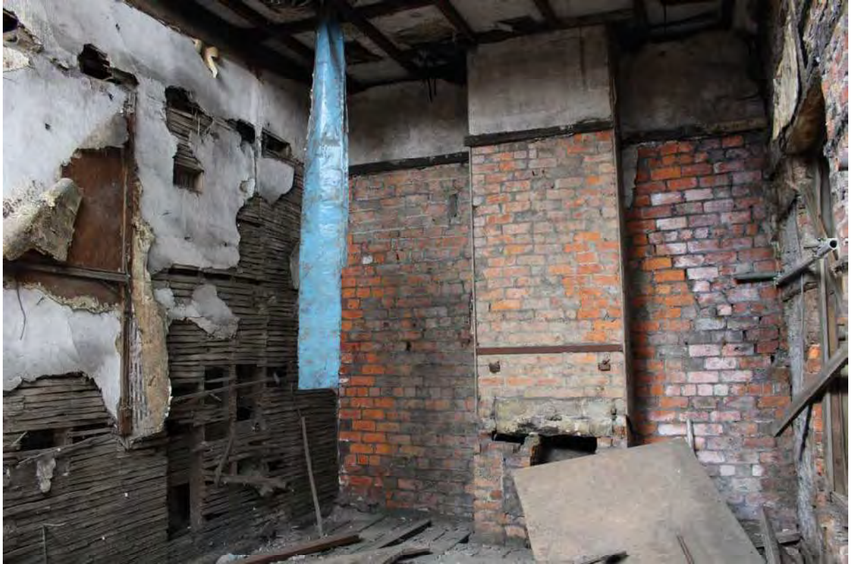
Plate 45 South range, south side room of the first floor
