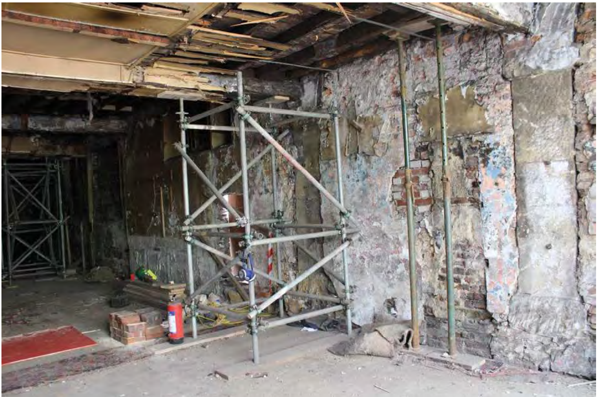
Plate 36 East range, west wall of ground floor
