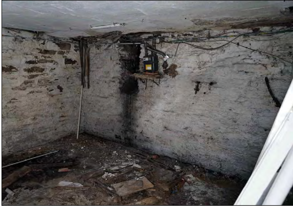
Plate 45. No. 2 cellar, looking south
