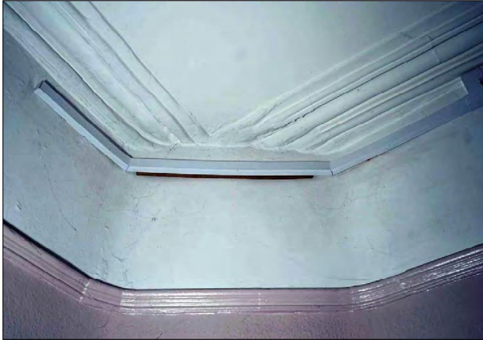
Plate 41. No. 2 ground floor middle room coving, looking north-west
