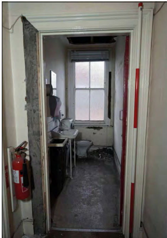
Plate 50. No. 2 WC, looking south-west
