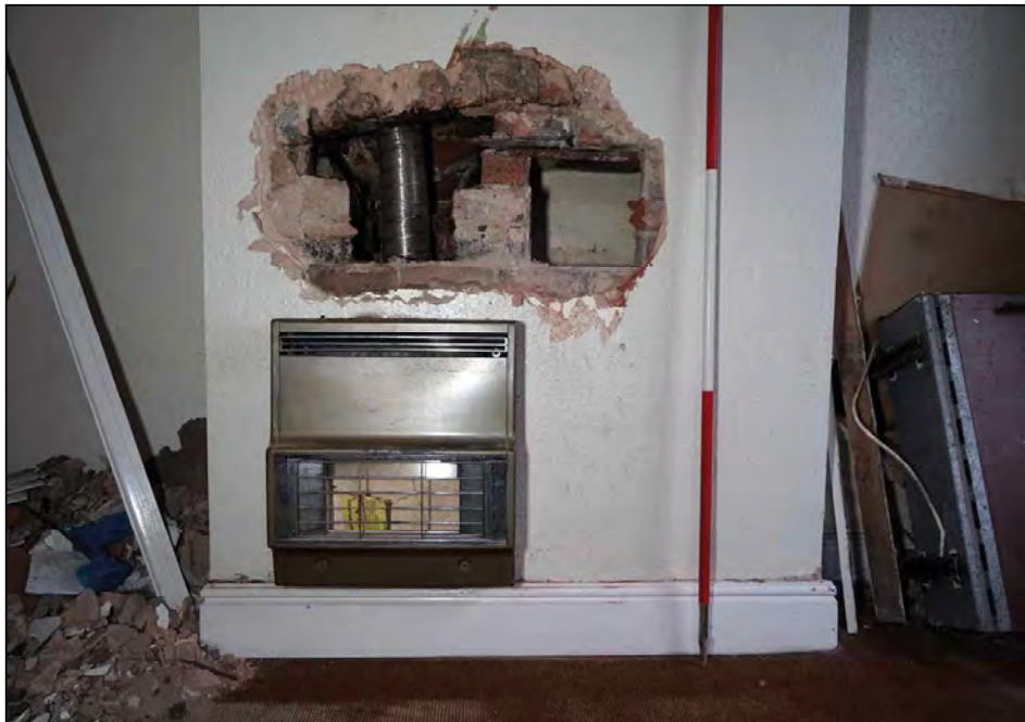
Plate 42. No. 2 ground floor backroom fireplace, looking north-west
