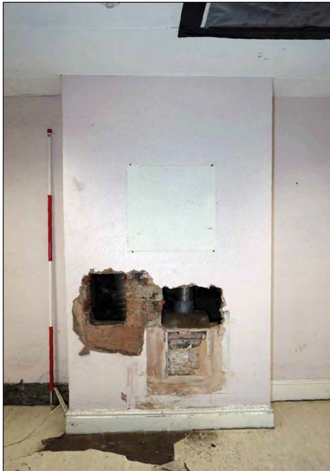
Plate 54. No. 2 first floor back room, looking north-west
