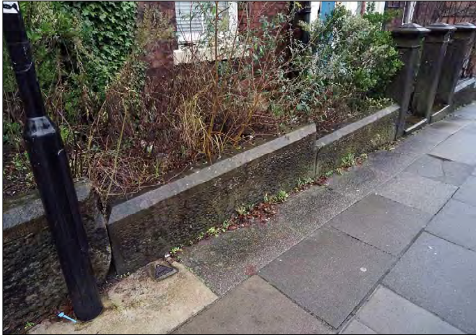
Plate 19. Yard wall of No. 4, looking east
