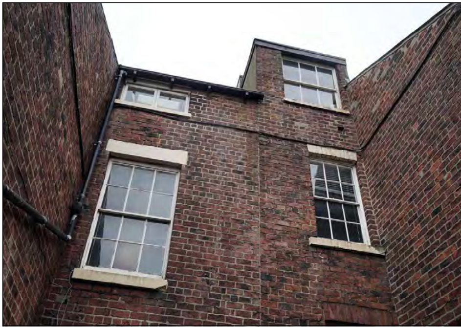
Plate 22. Nos. 4 and 6 upper windows, looking south-west
