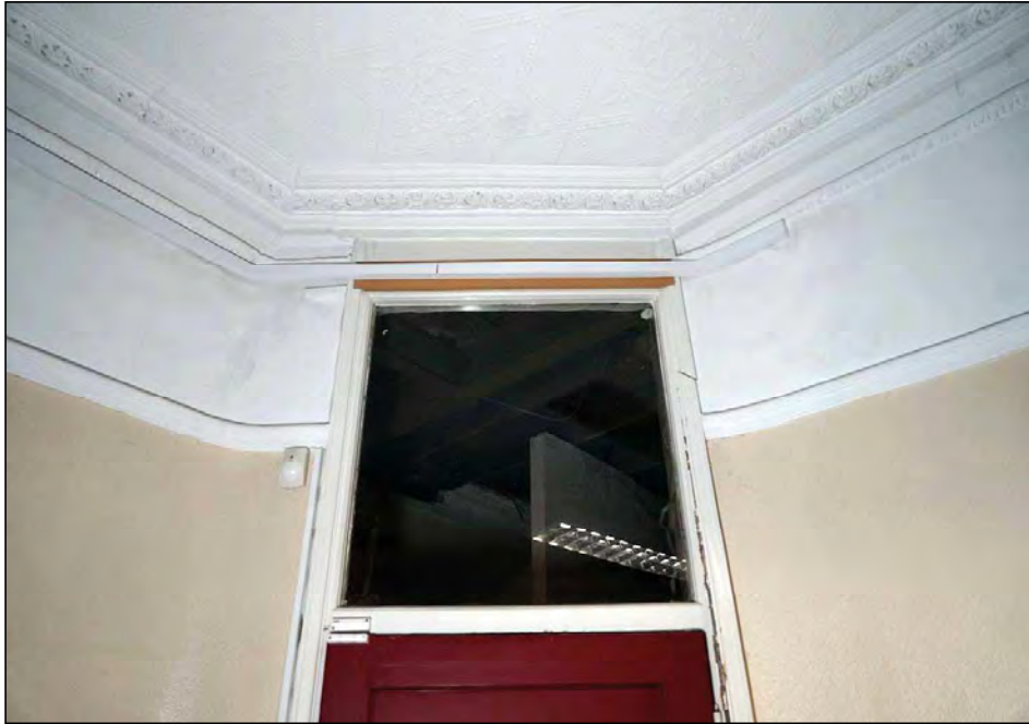
Plate 39. No. 2 ground floor front room coving and doorway, looking west
