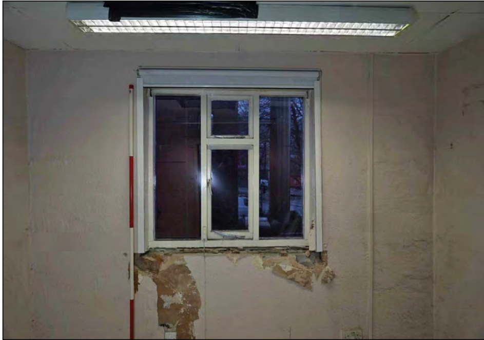
Plate 55. No. 2 first floor back bedroom window, looking north-east
