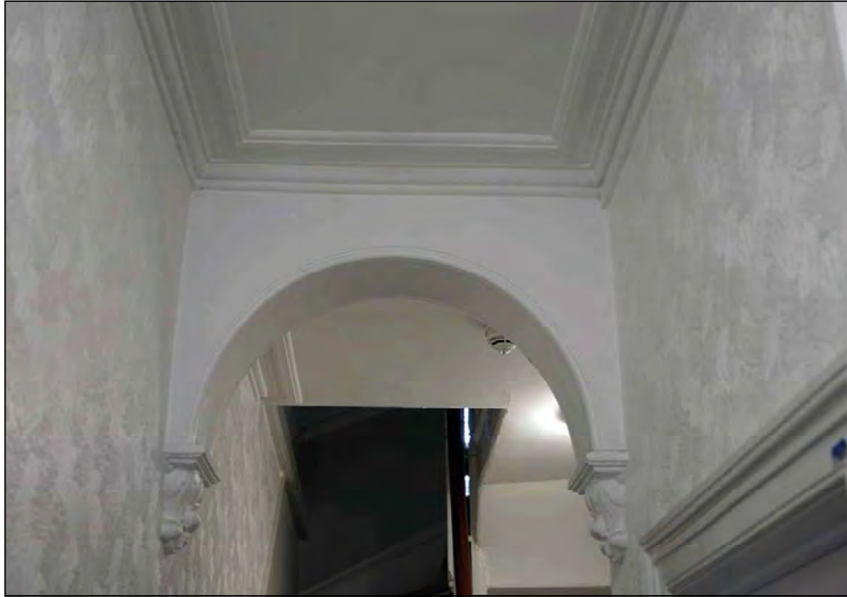
Plate 101. No. 6 hallway arch, looking north-east
