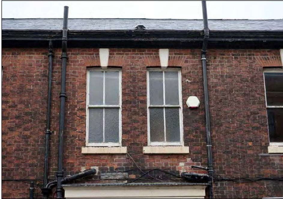
Plate 17. Smaller first floor windows of Nos. 2 and 4
