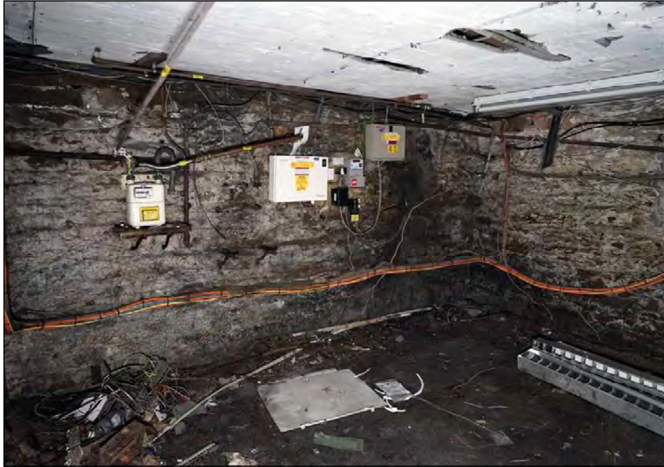
Plate 75. No. 4 cellar, looking south
