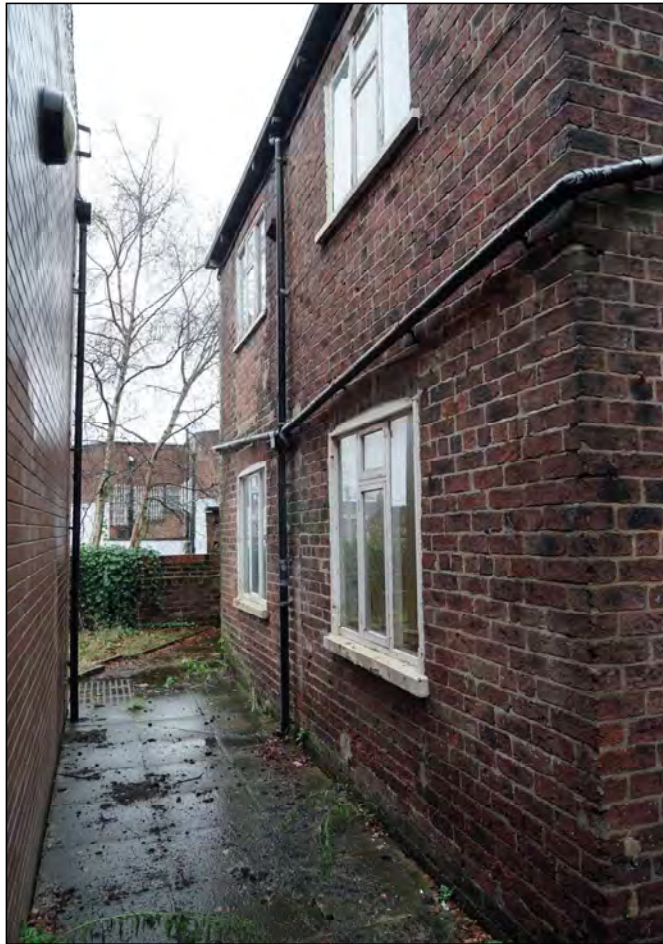
Plate 23. Rear of Nos. 2 and 4, looking south-east
