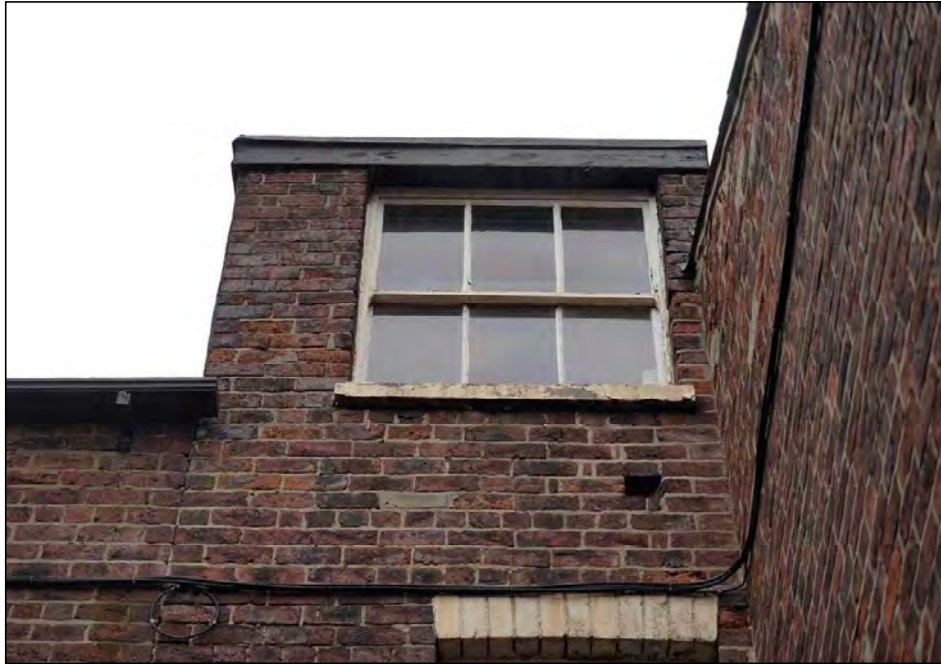
Plate 93. No. 6 rear second floor window, looking south-west
