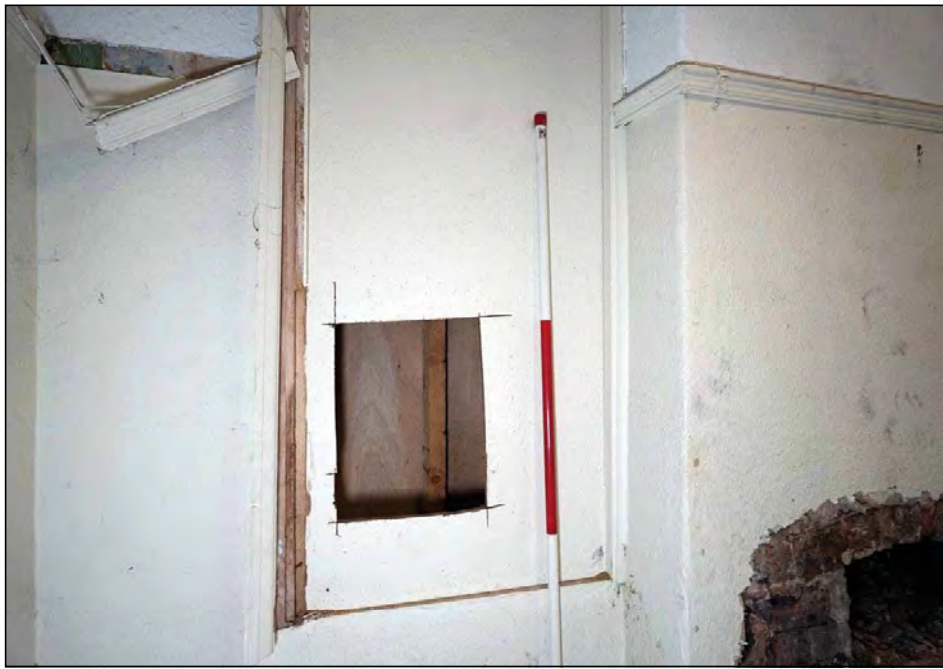
Plate 72. No. 4 ground floor middle room infilled niche, looking north-west
