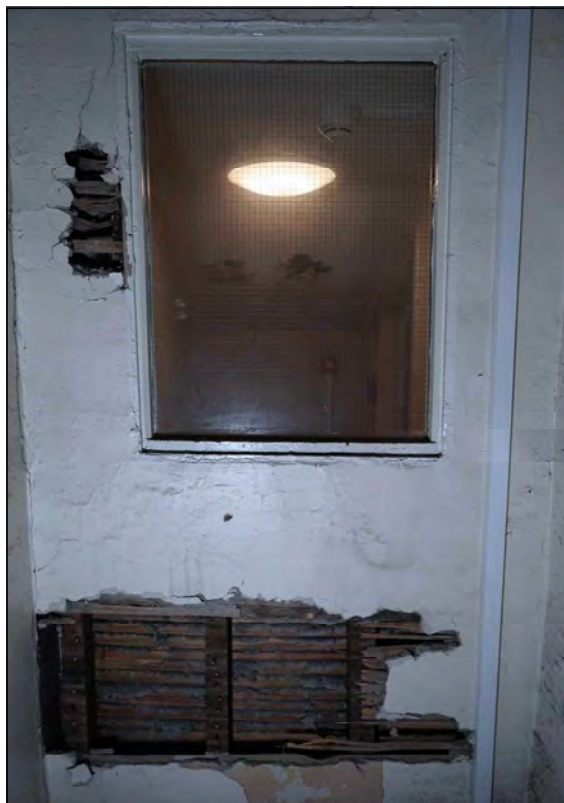
Plate 60. No. 2 second storey small room, looking north-east
