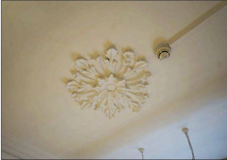
Plate 103. No. 6 ground floor ceiling rose, looking south
