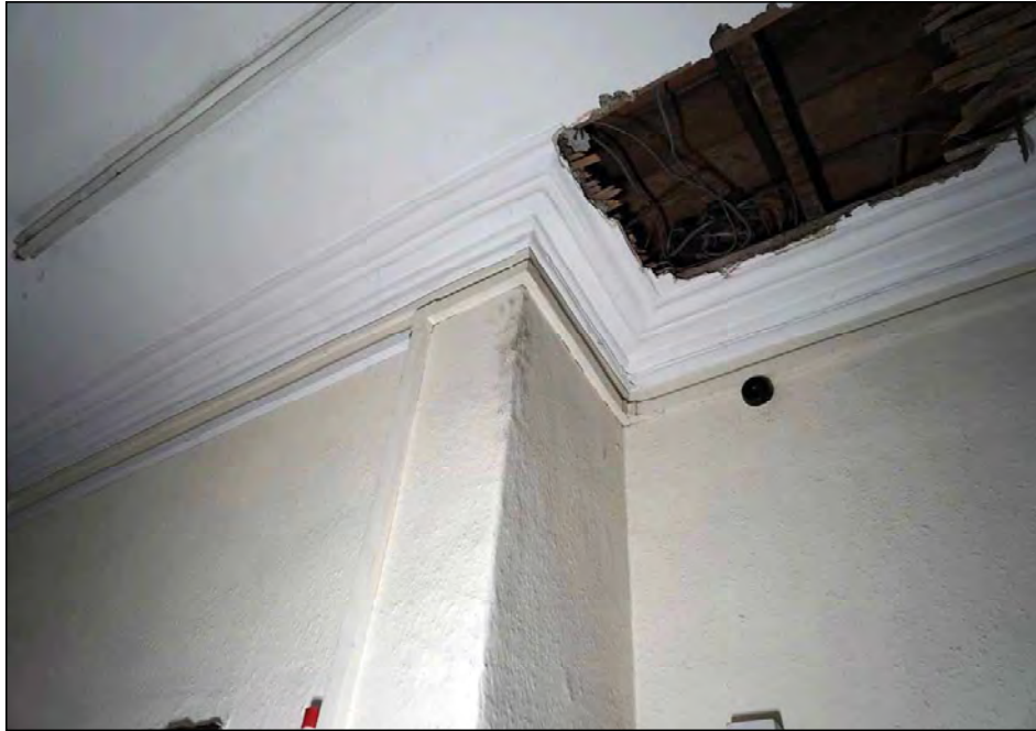
Plate 63. No. 4 hallway coving, looking west
