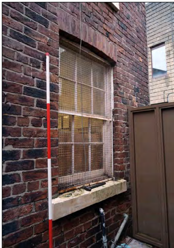
Plate 96. No. 6 rear ground floor window, looking west
