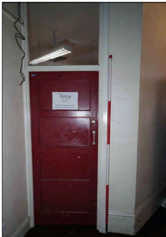
Plate 32. Doorway to the ground floor front room of No. 2, looking south
