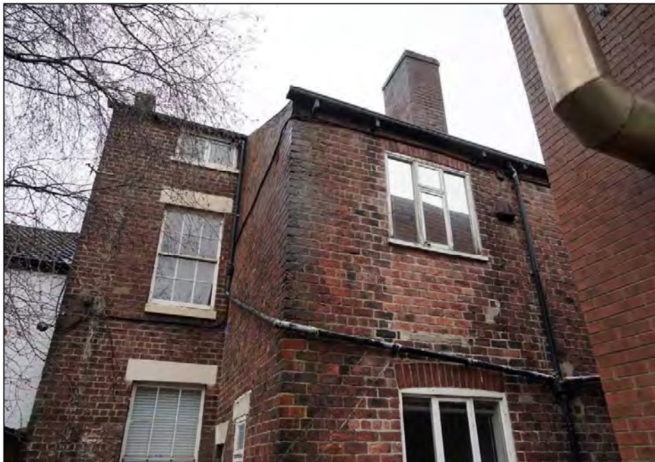
Plate 28. Nos. 2 and 4 rear chimney stack, looking south-west
