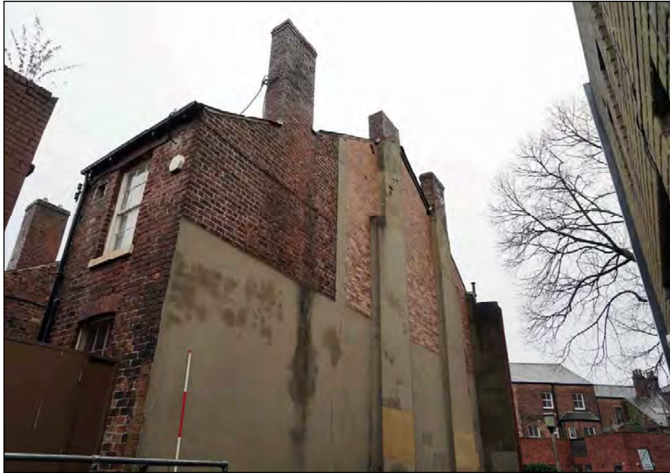
Plate 85. No. 6 north-west facing elevation , looking south
