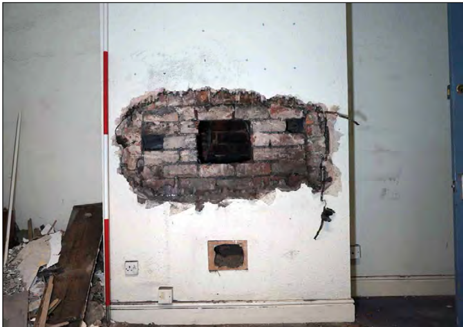
Plate 74. No. 4 ground floor back room fireplace, looking south-east
