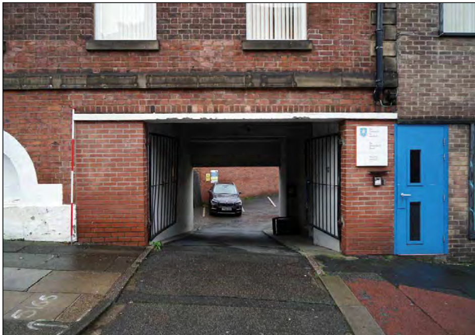
Plate 4. Car park entrance ramp, looking north-east
