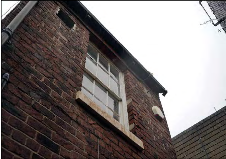
Plate 97. No. 6 rear first floor window, looking west
