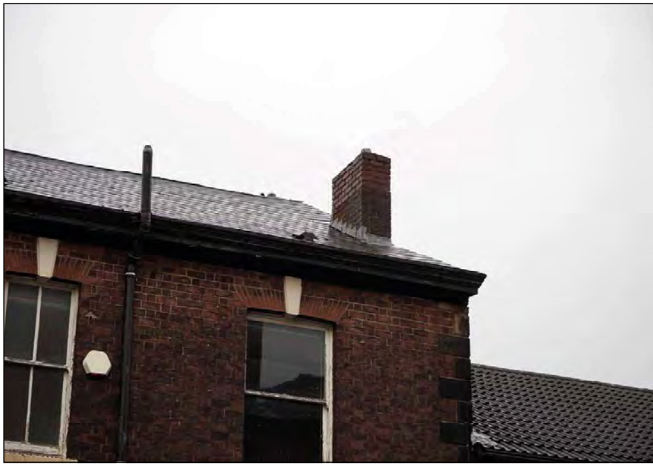
Plate 26. No. 2 chimney stacks, looking east
