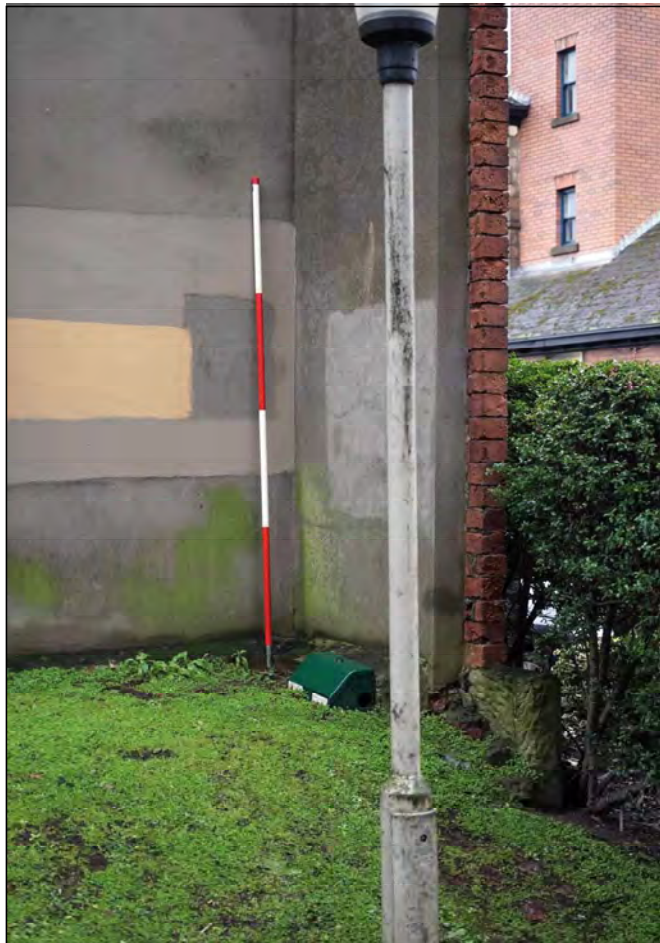
Plate 86. Wall extending north-west from No. 6 representing the remains of No. 8, looking south
