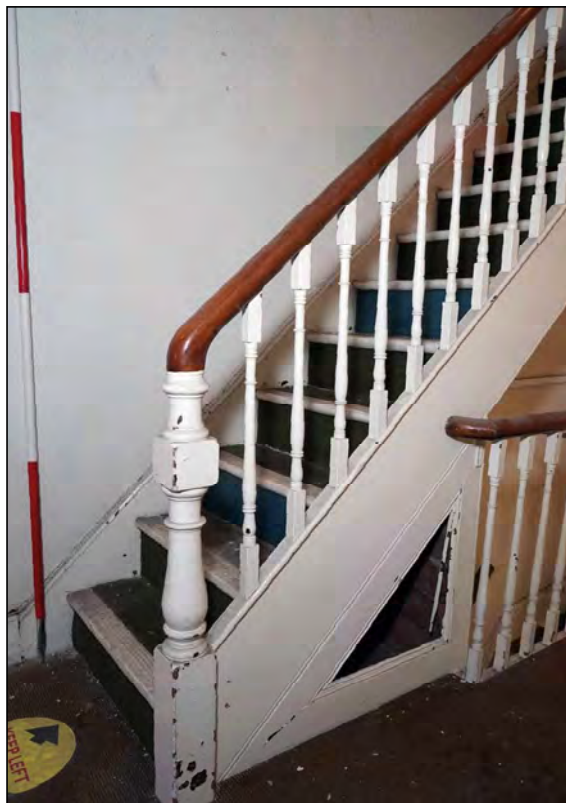
Plate 48. No.2 staircase to second floor, looking north
