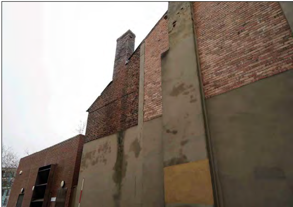
Plate 90. North-west facing elevation of No. 6, looking east
