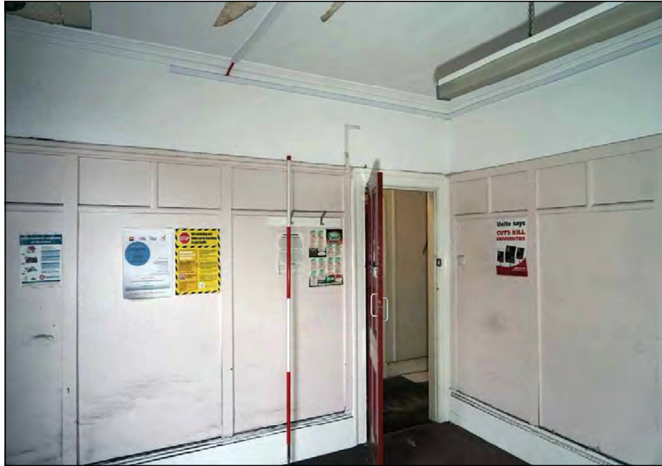
Plate 51. No. 2 first floor front room, looking north
