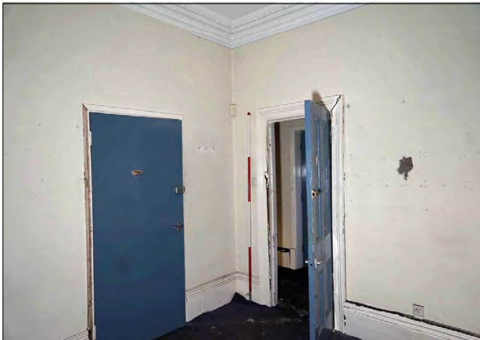
Plate 68. No. 4 ground floor front room, looking east
