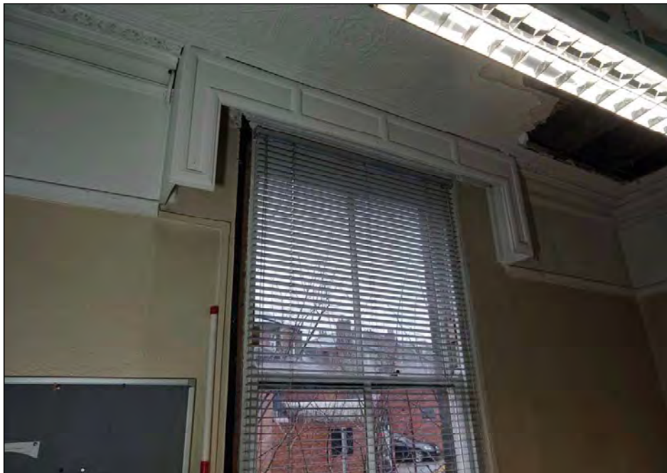
Plate 34. No. 2 ground floor front room window cornice, looking south-west
