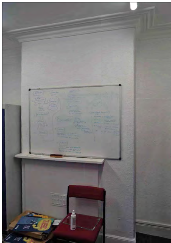
Plate 116. No. 6 first floor middle room fireplace, looking east
