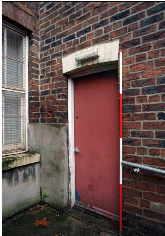
Plate 95. No. 6 rear door, looking west
