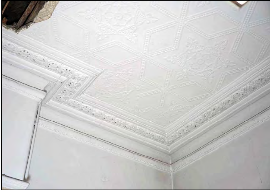
Plate 35. No. 2 ground floor front room coving, looking south
