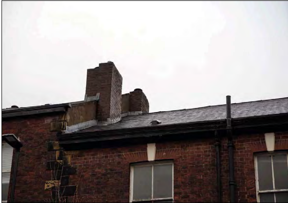
Plate 27. No. 4 chimney stacks, looking north
