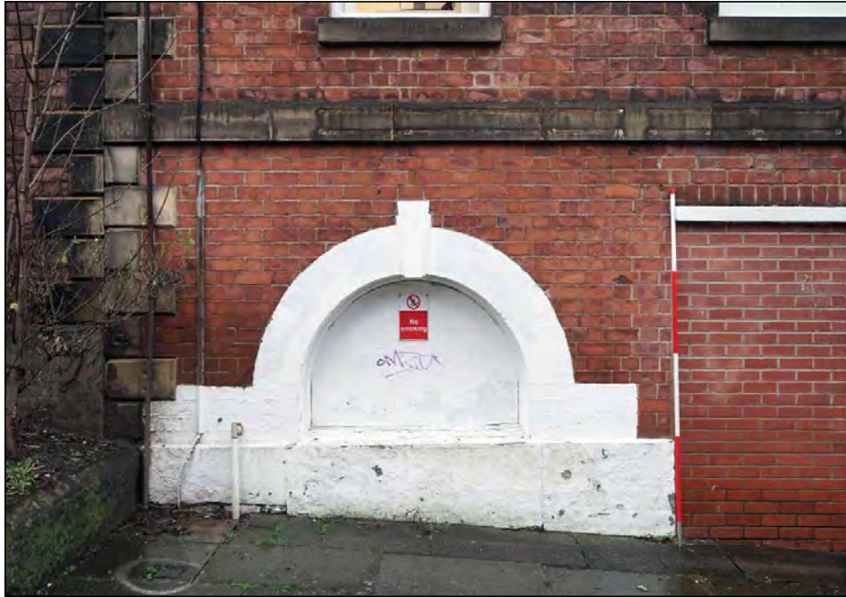
Plate 3. Blocked arched window, looking north-east
