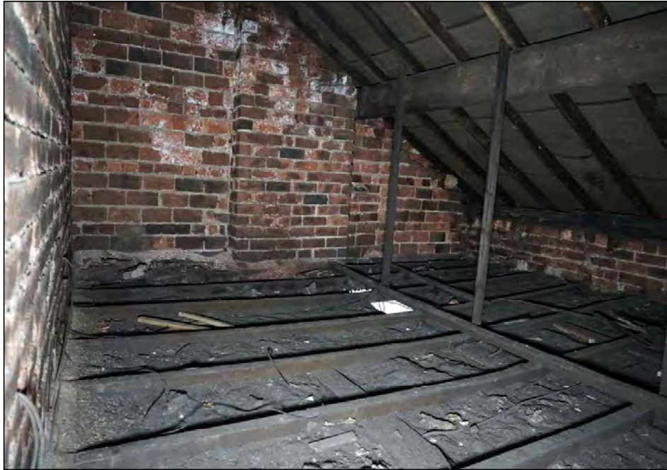
Plate 57. No. 2 roof space, looking south-east
