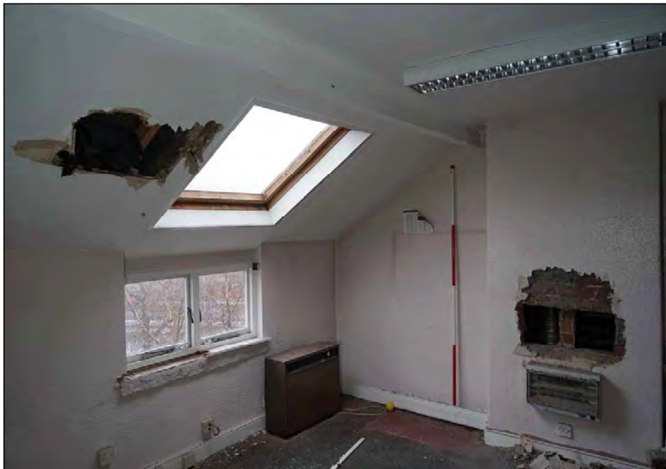
Plate 56. No.2 second floor large room, looking east
