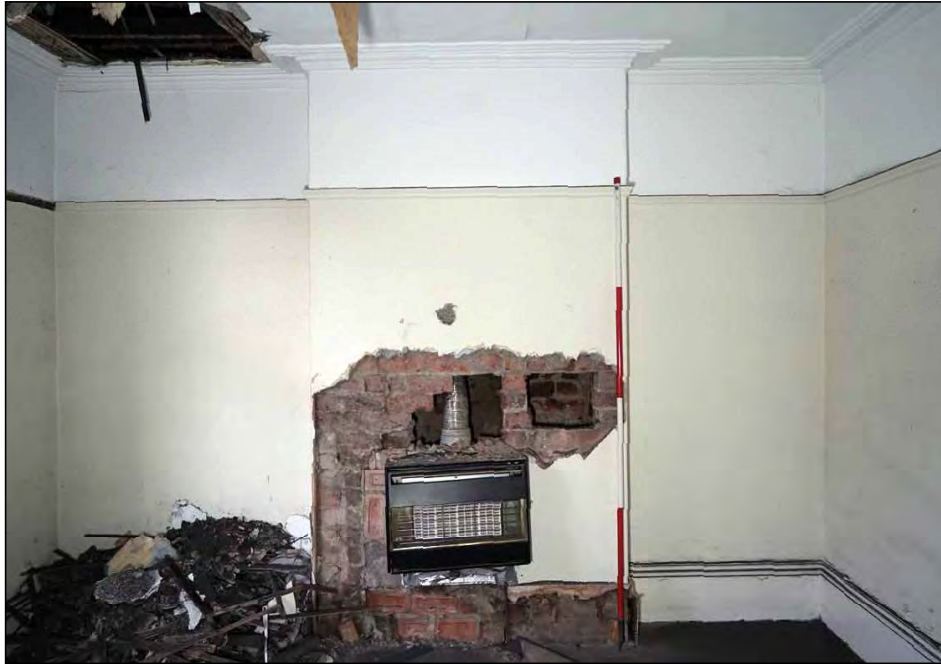
Plate 79. No. 4 first floor front room, looking north-west
