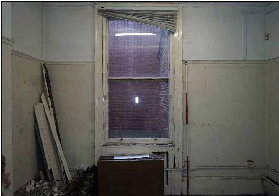
Plate 70. No. 4 ground floor middle room window, looking north-east
