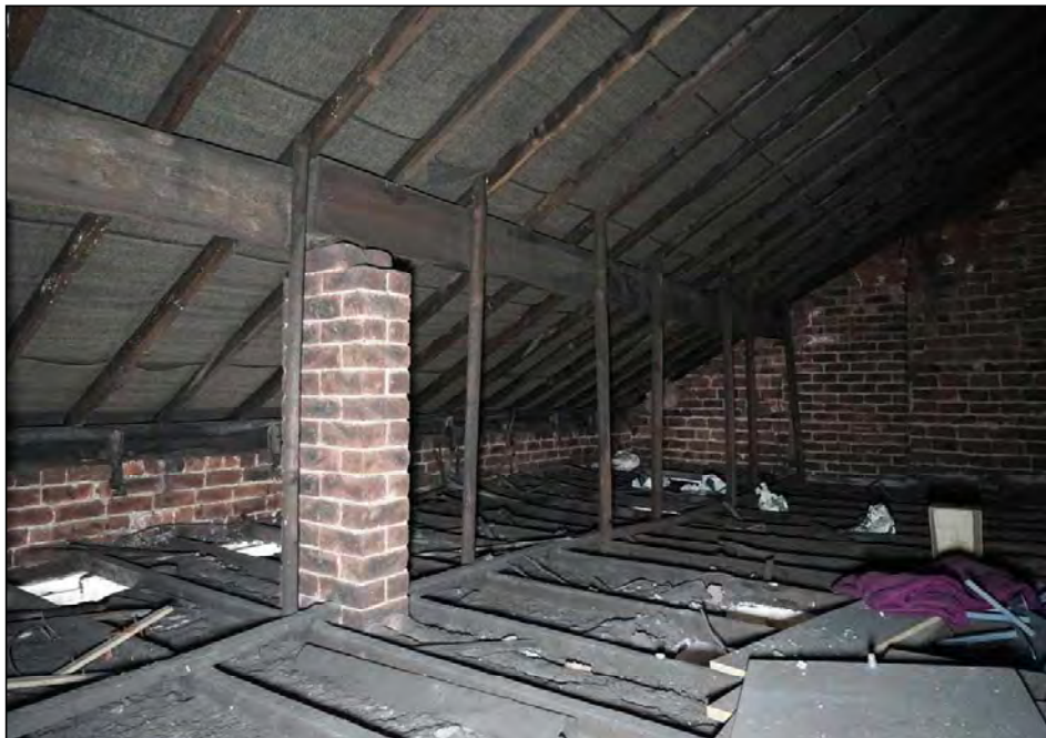
Plate 58. No. 2 roof space, looking west
