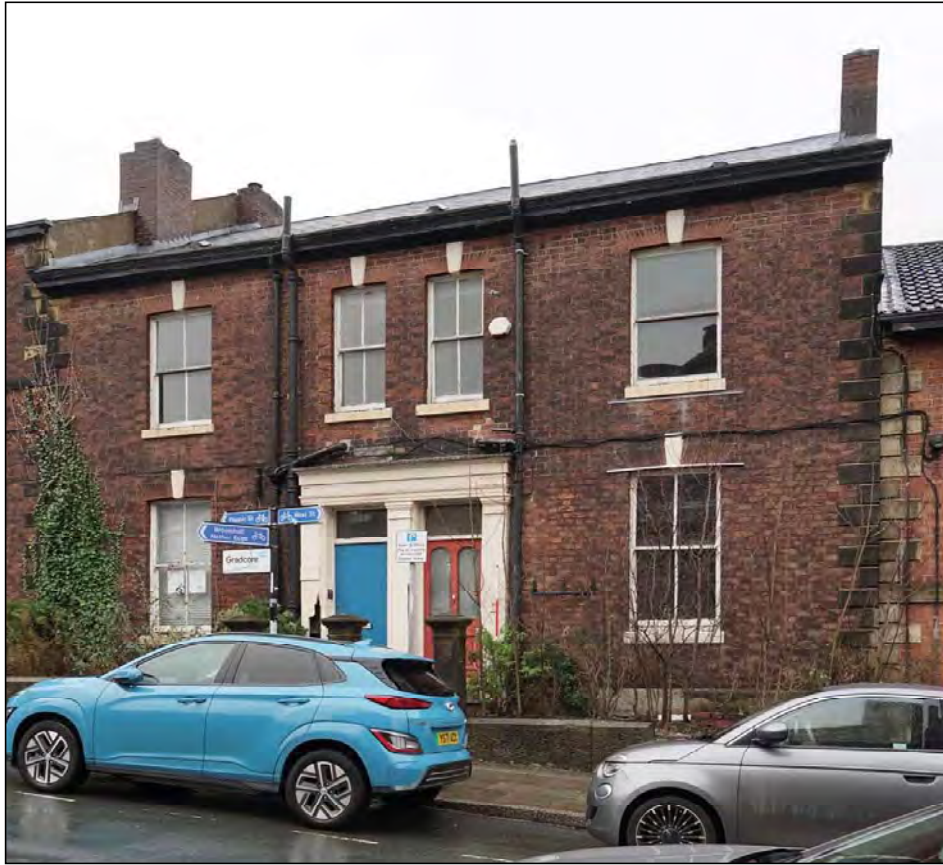
Plate 11. Nos. 2 and 4, looking north-east
