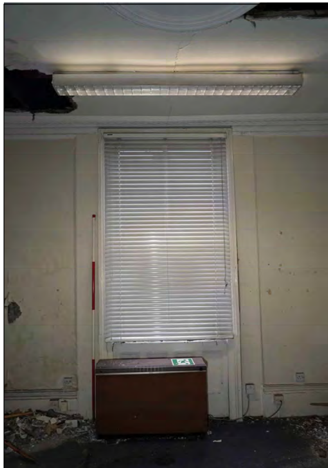
Plate 66. No. 4 ground floor front window, looking south-west
