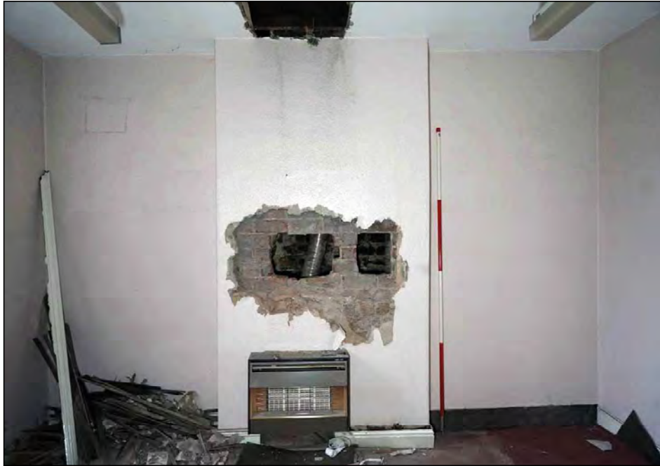
Plate 53. No. 2 first floor middle room fireplace, looking south-east
