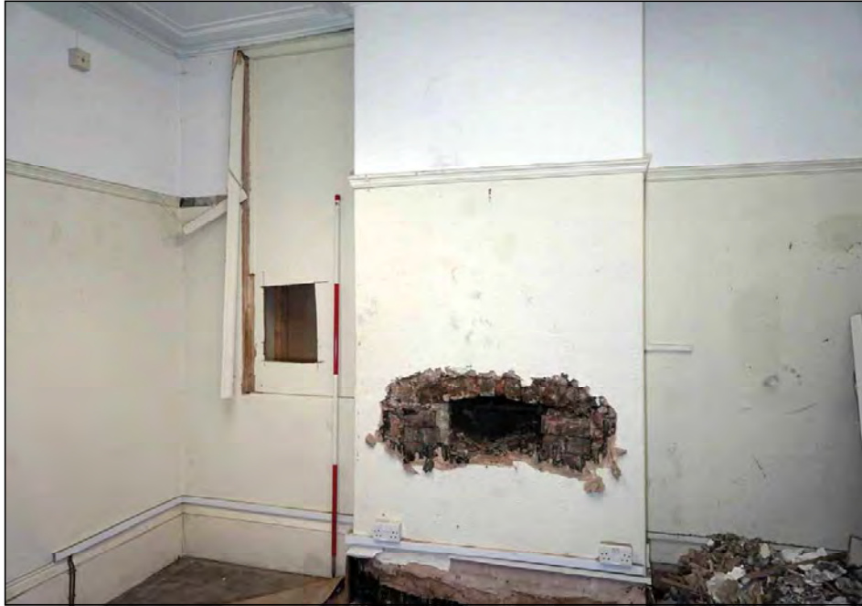
Plate 71. No. 4 ground floor middle room fireplace, looking north-west
