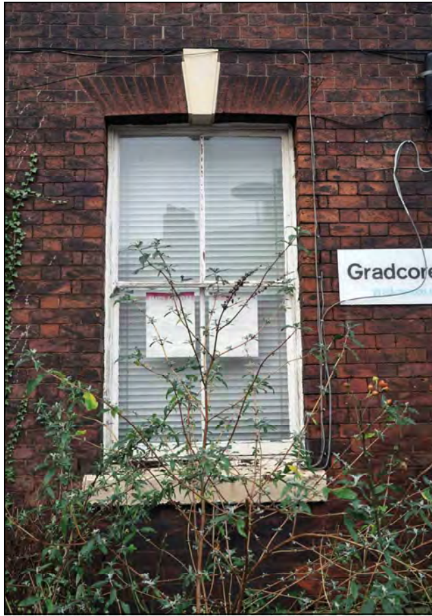
Plate 15. No. 4 ground floor sash window, looking north-east
