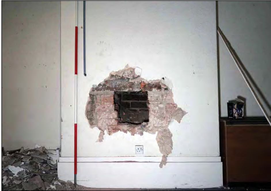
Plate 67. No. 4 ground floor front room fireplace, looking north-west
