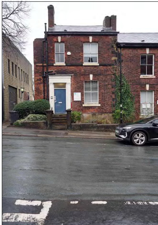
Plate 84. No. 6, south-west facing elevation, looking north-east
