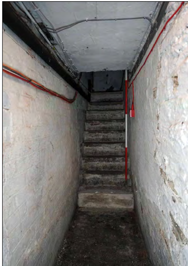
Plate 44. No. 2 cellar steps, looking north-east
