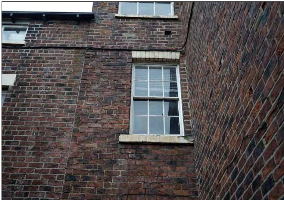
Plate 92. No.6 rear first floor window, looking south-west
