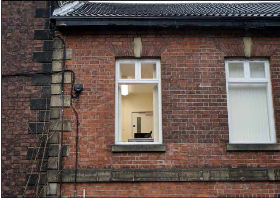
Plate 5. No. 2a first floor windows, looking north-east
