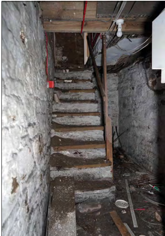
Plate 110. No. 6 cellar steps, looking north-east
