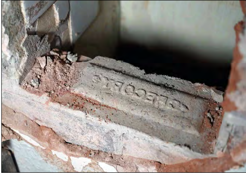
Plate 43. No. 2 ground floor middle room fireplace mortar impression
