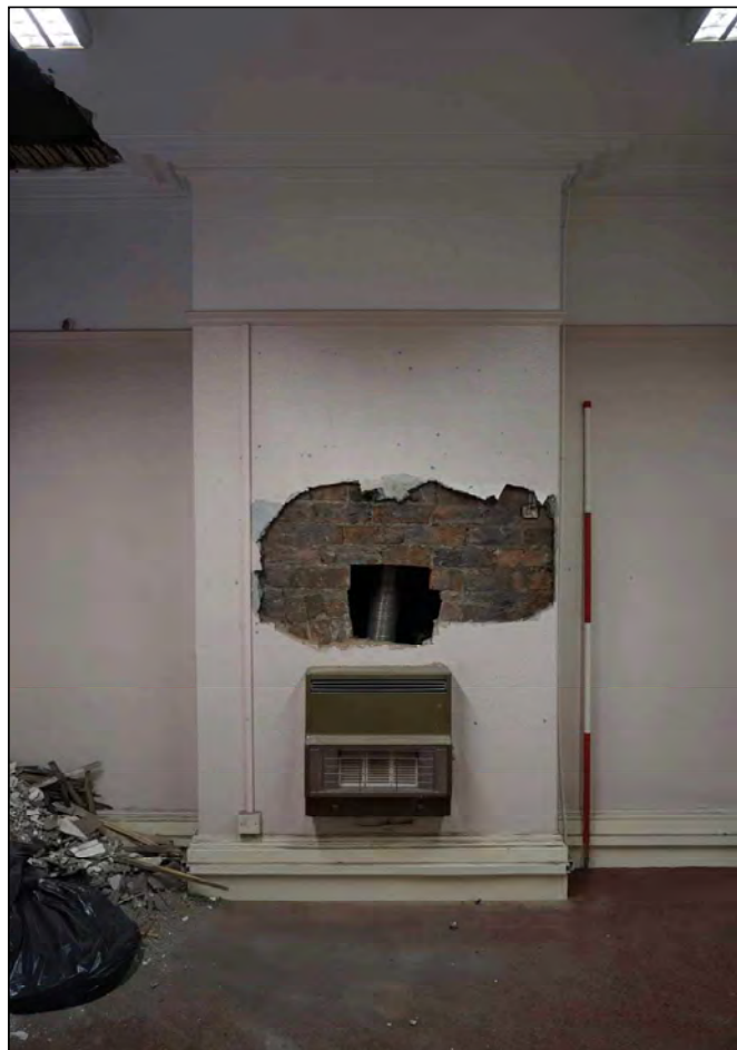
Plate 40. No. 2 ground floor middle room fireplace, looking south-east
