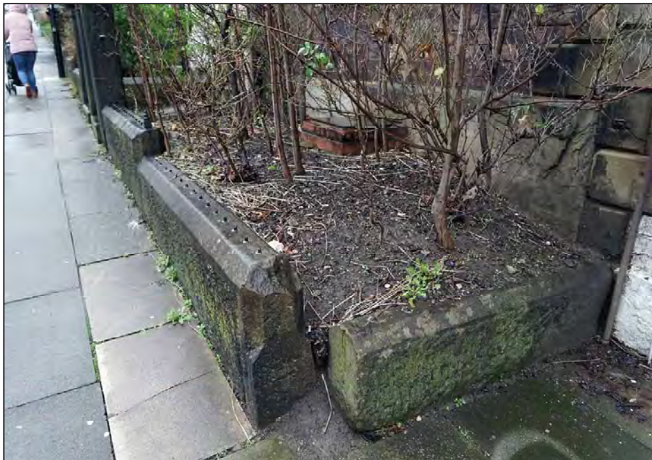
Plate 18. Yard wall of No. 2, looking north
