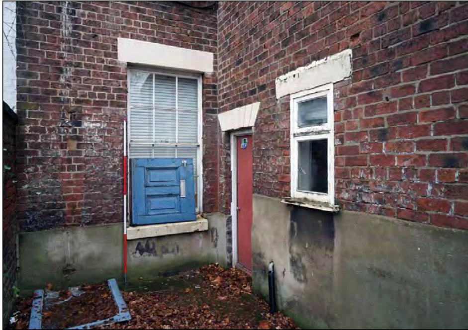
Plate 25. Rear yard of No. 2, looking south-west
