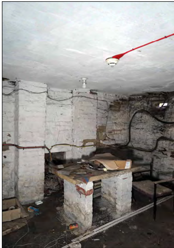
Plate 111. No. 6 cellar ash pit and table, looking east
