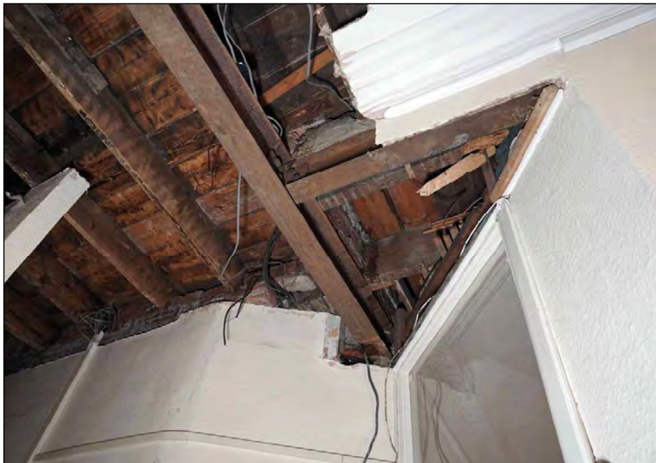
Plate 38. No. 2 ground floor front room wall modification
