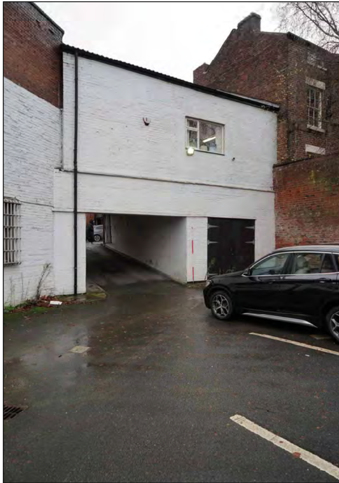
Plate 7. The rear of No. 2a, looking west
