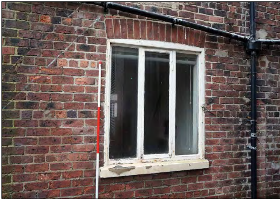
Plate 24. No. 4 rear window, looking south-west
