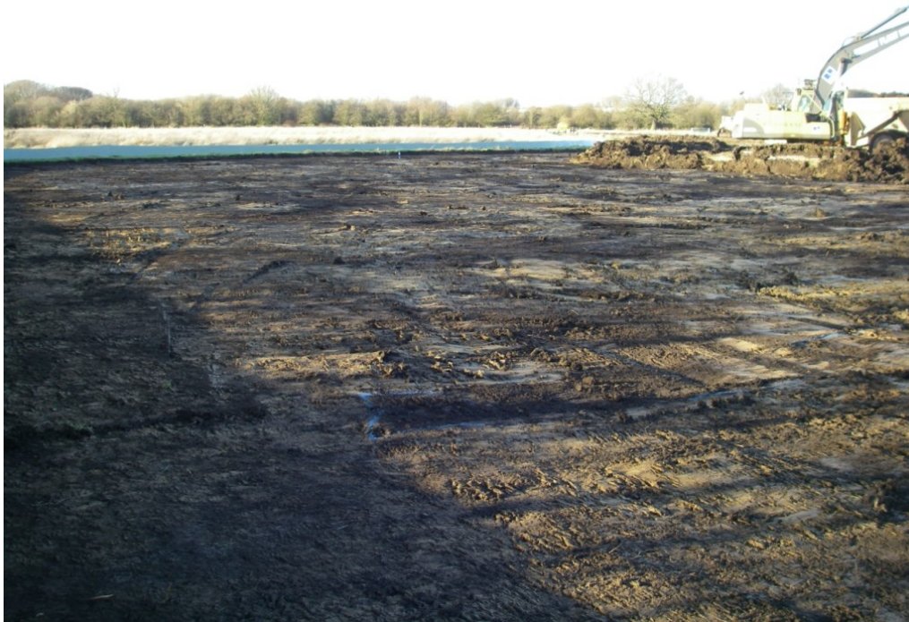
Plate 1: General shot of site during the topsoil strip
