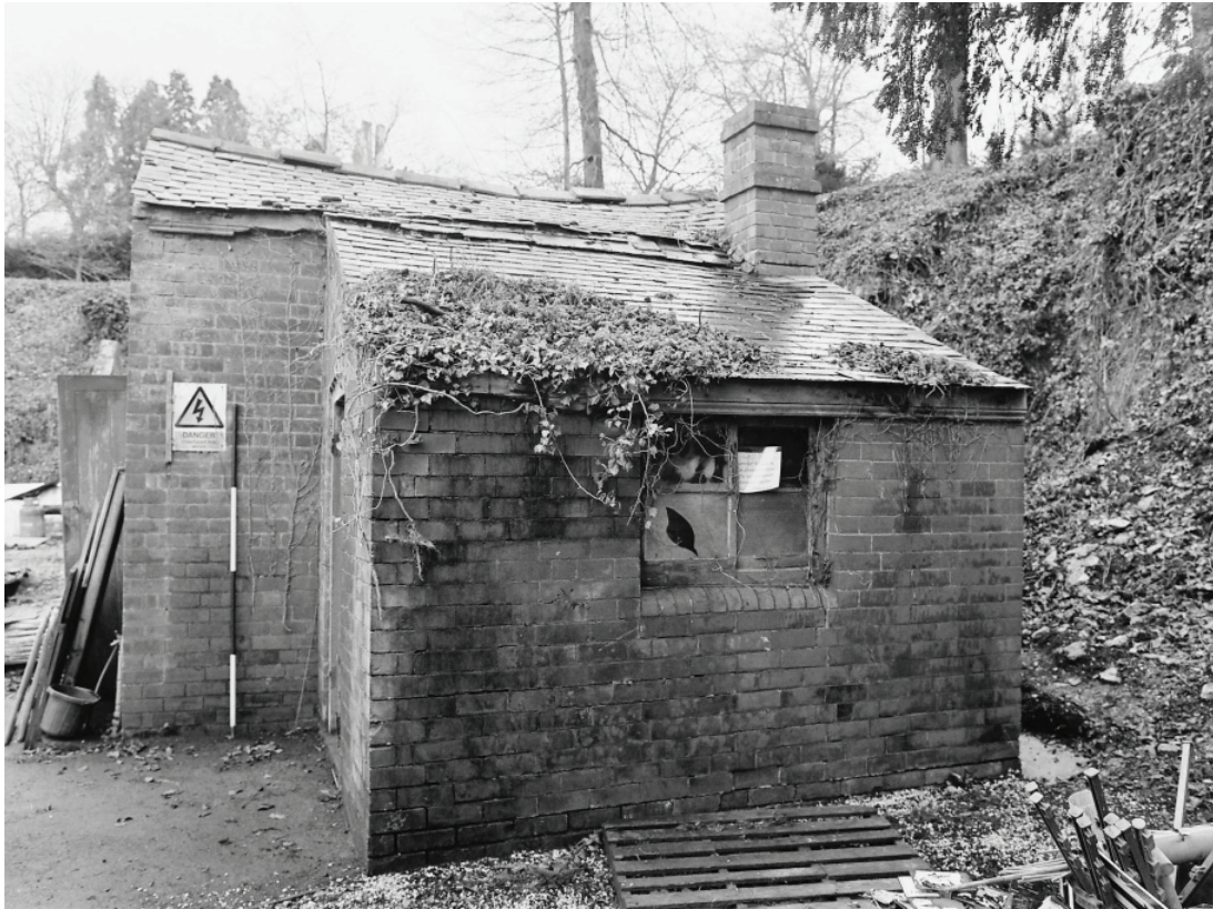
Photograph 11 Film 2_15 Direction SE
