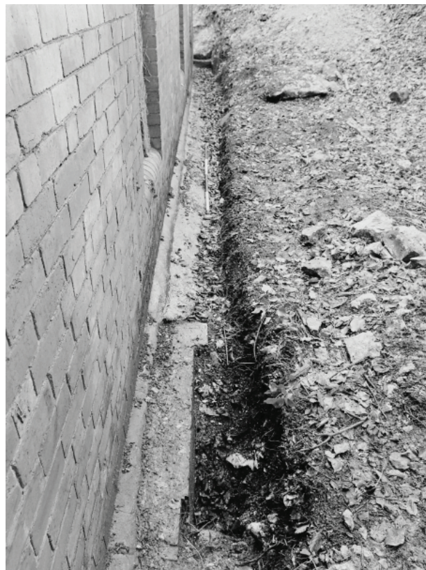
Photograph 14 Film 3_2 Direction SE
