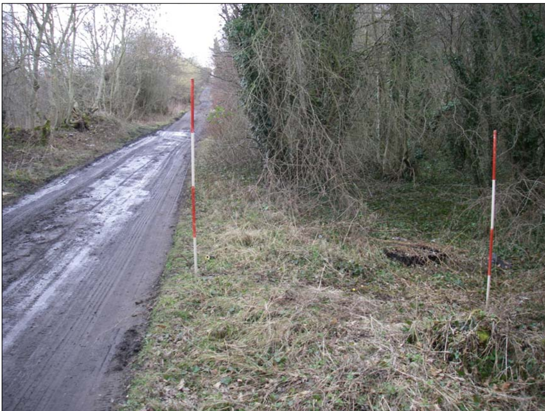
Plate 34. Length of scarp on the eastern side of the modern road in Section 8, looking north-west
