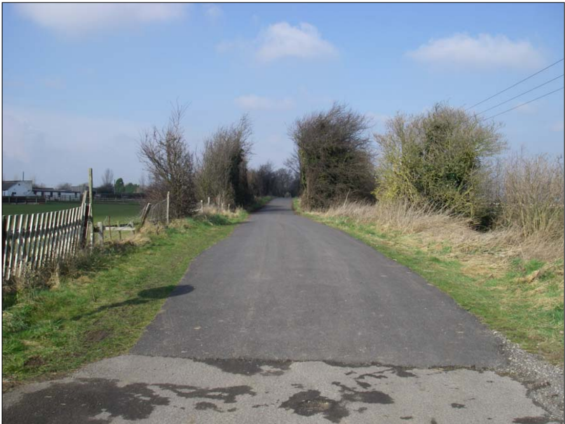
Plate 58. The southern end of Section 11, looking north-west
