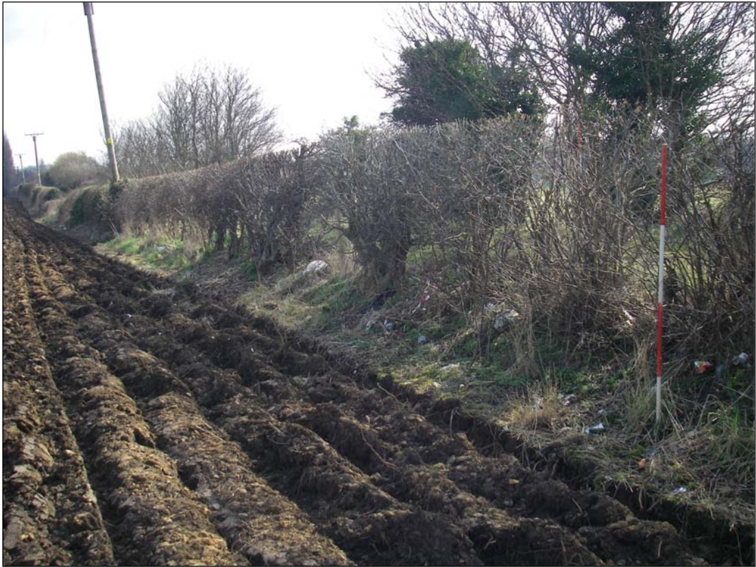
Plate 71. Part of the north-eastern side of the agger in Section 13, looking south
