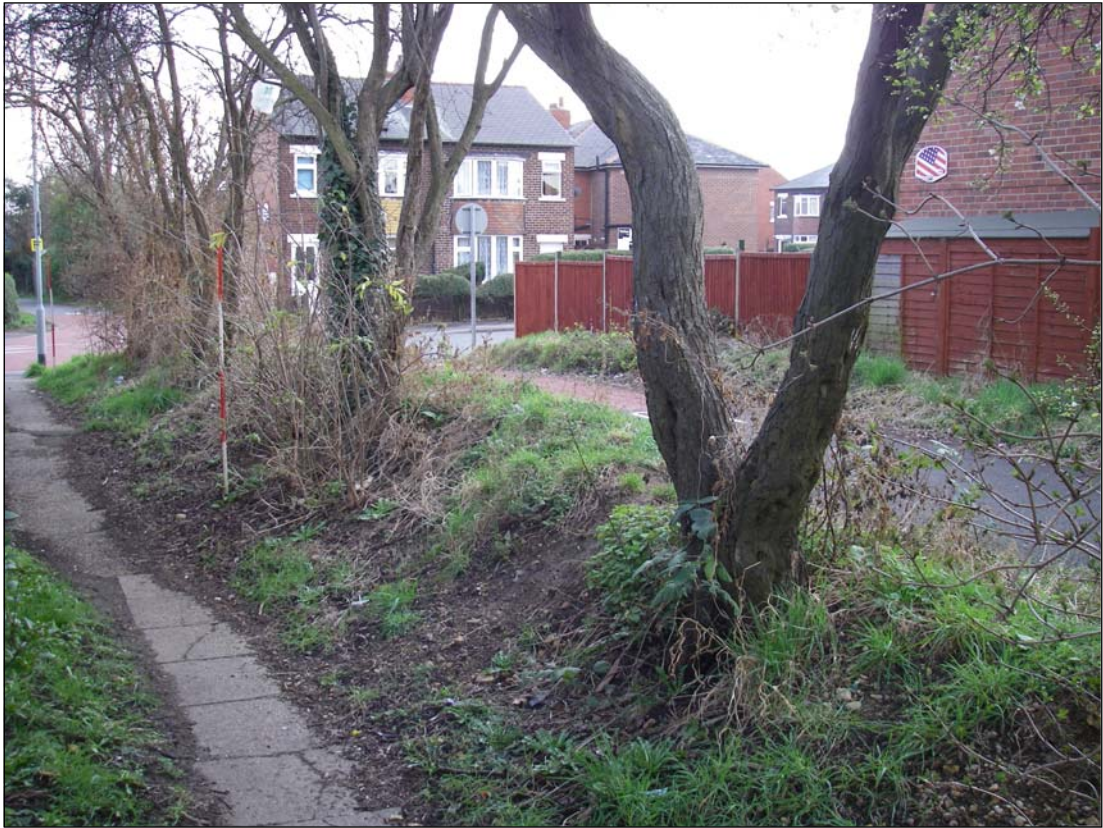
Plate 77. The length of bank at the corner of Sledmere Road and Alwyn Avenue, possibly the remains of the north-eastern side of the agger, in Section 14, looking south
