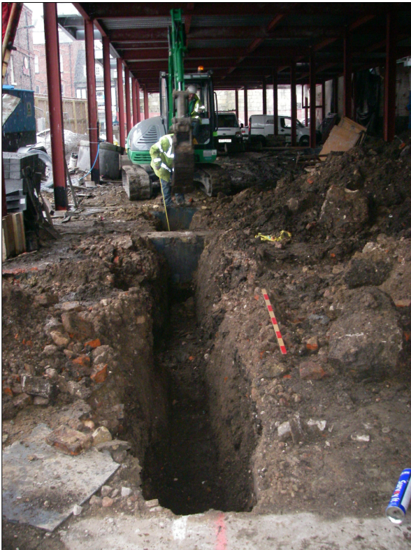
Plate 2. Deepest portion of south-eastern service trench, looking south-west
