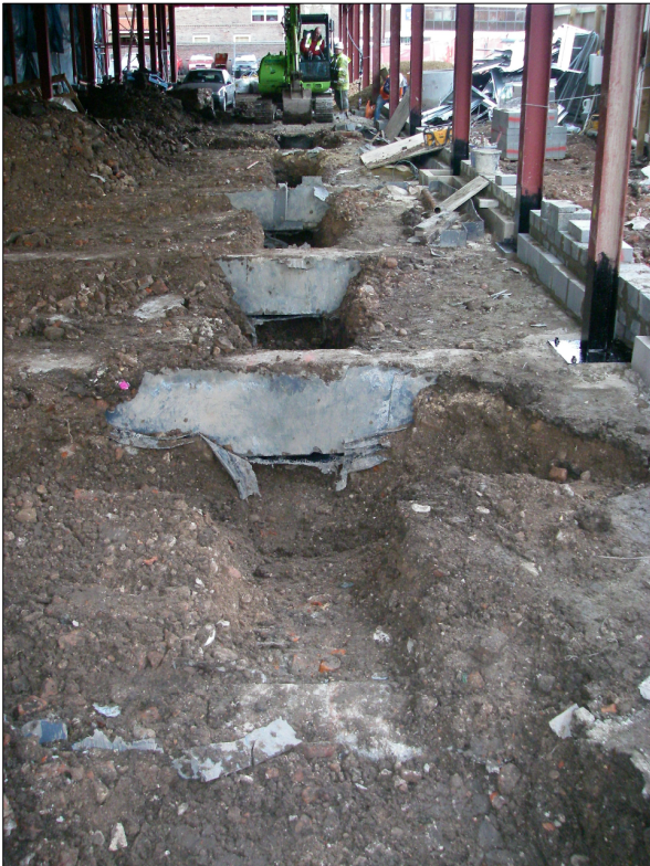
Plate 1. Excavations of south-eastern service trench running from Bootham to the north-east
