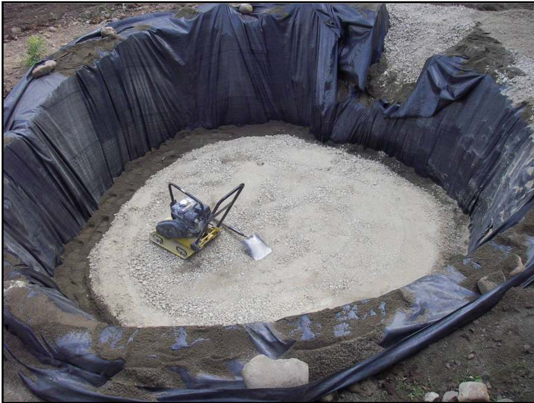
Plate 27: The Type 1 hardcore was regularly compacted with a single direction vibrating plate
