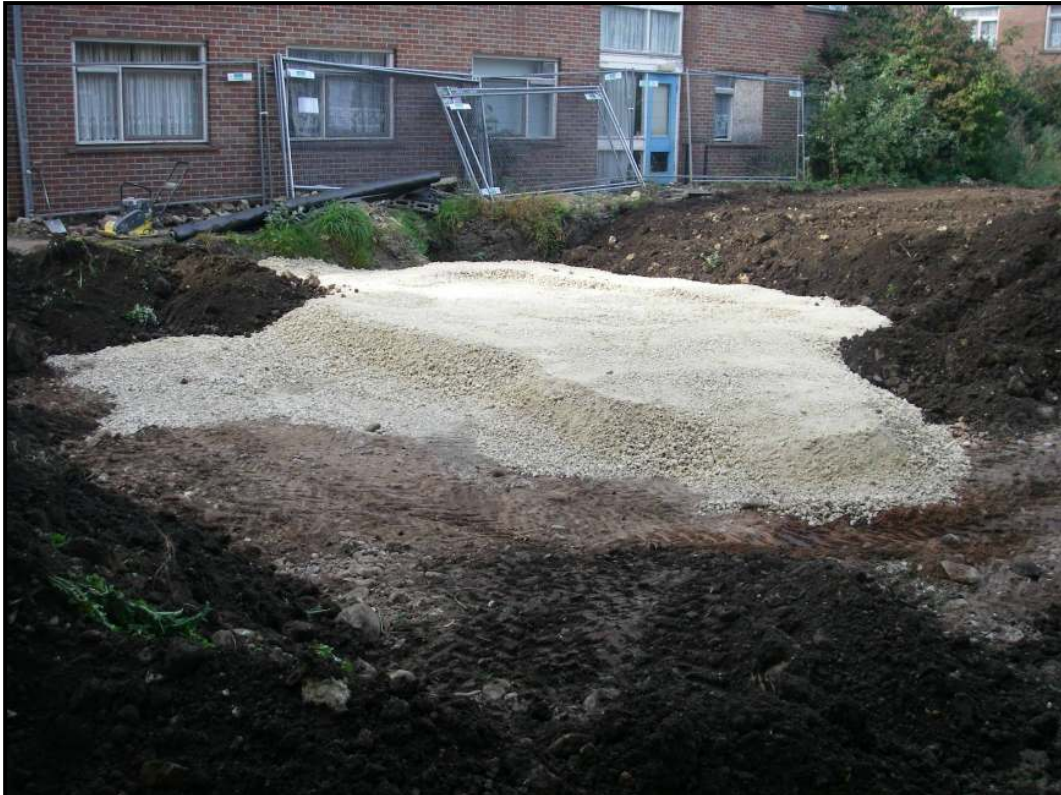
Plate 27: The Type 1 hardcore was regularly compacted with a single direction vibrating plate
