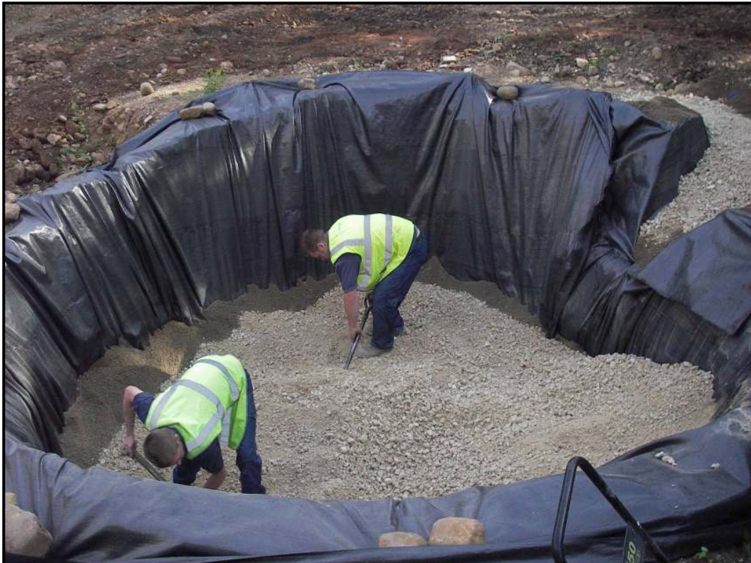
Plate 26: The kiln with a lower, outer layer of clean sharp sand followed by Type 1 hardcore
