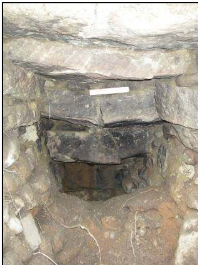
Plate 11: View into structure 1001
