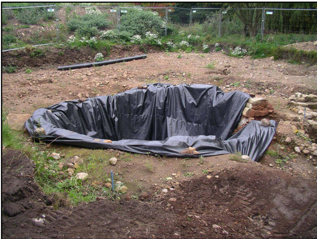
Plate 24: The kiln with the Terram lining in place
