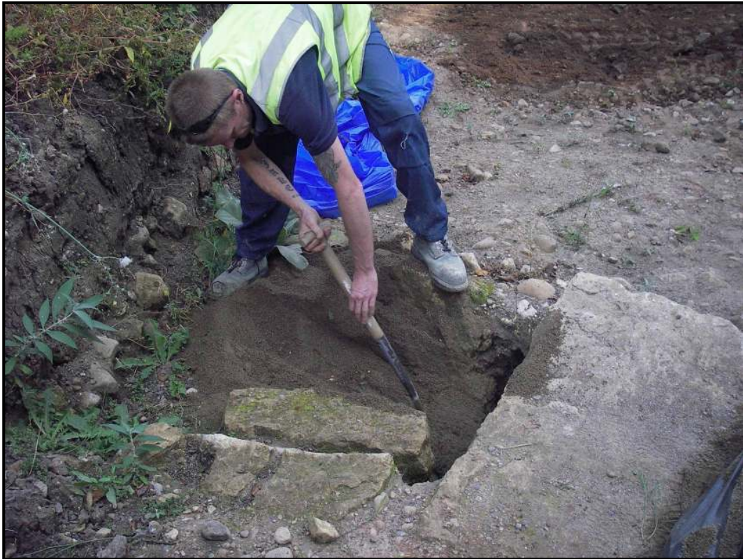
Plate 25: Backfilling the north-western flue with clean sharp sand
