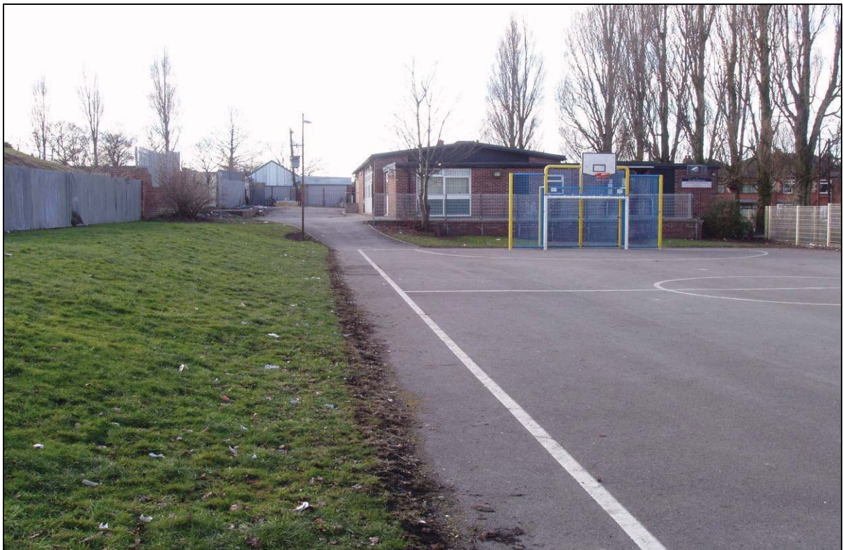
Plate 2. The Tom Hill Youth Centre viewed facing west from the south-eastern corner of the ball court
