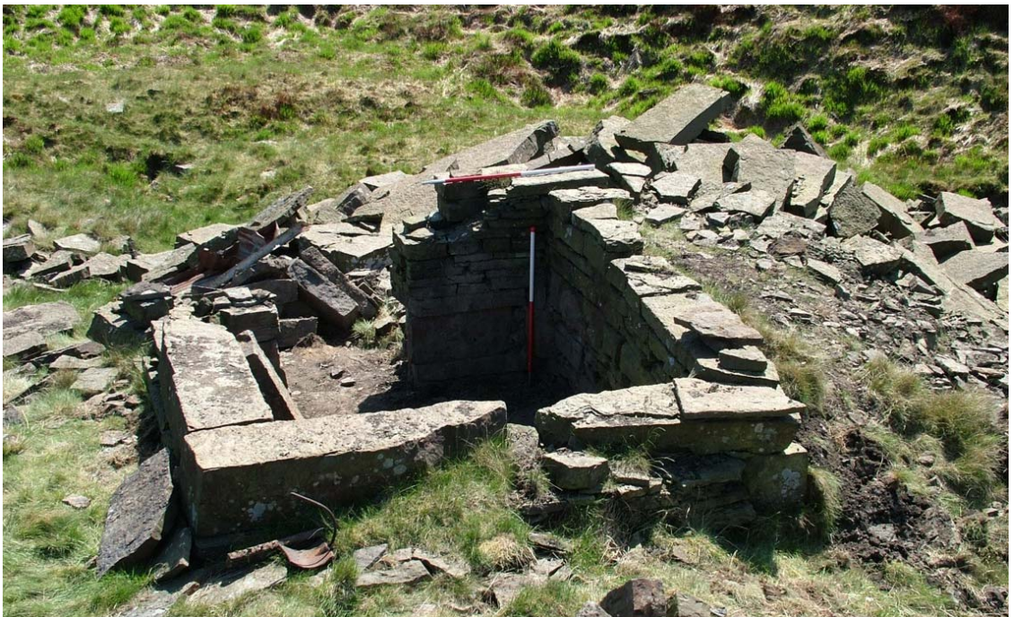
Plate 8: Looking into Hut 34 from North after Clearance
