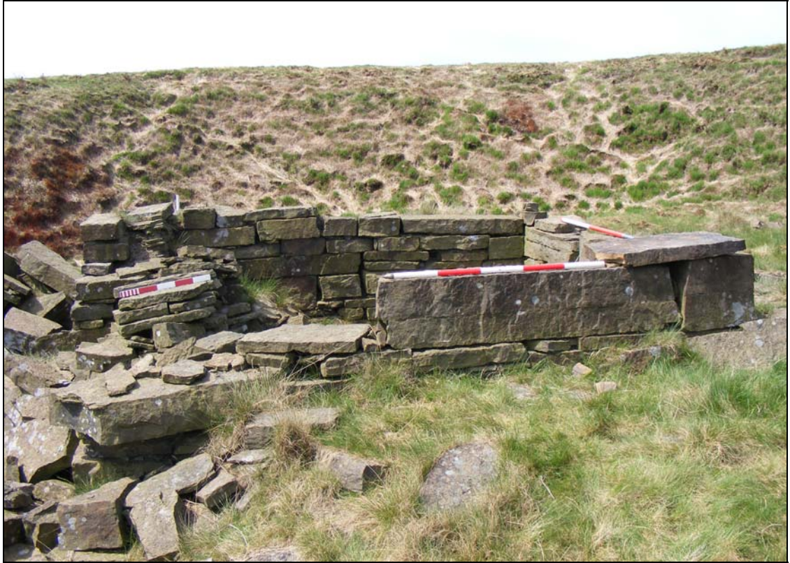
Plate 3: Close up of East Elevation
