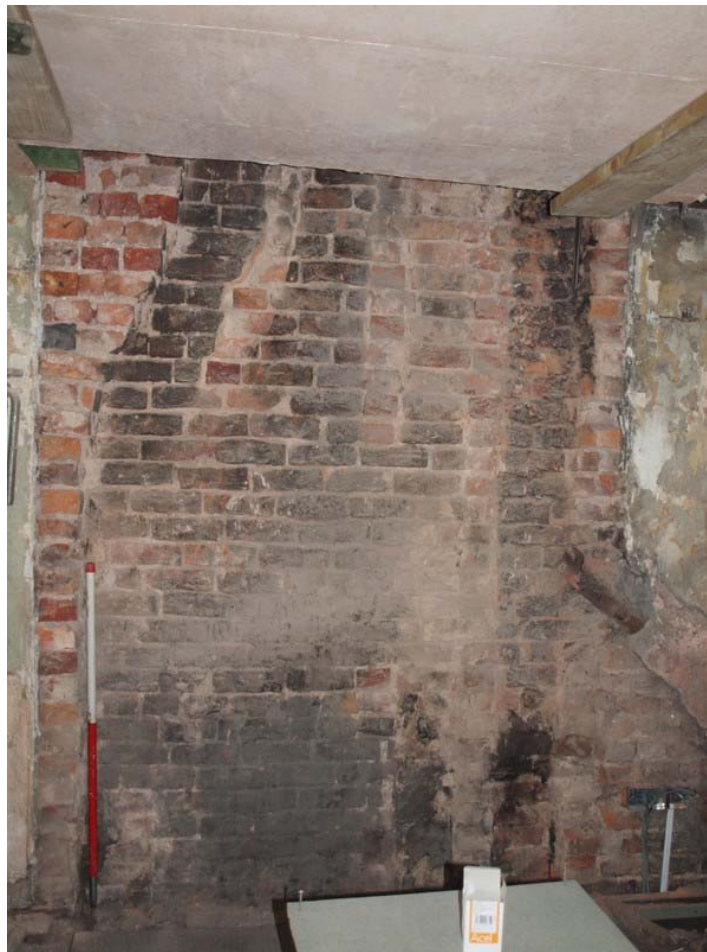
Plate 32: Chimney breast in room 6 after removal of rubble
