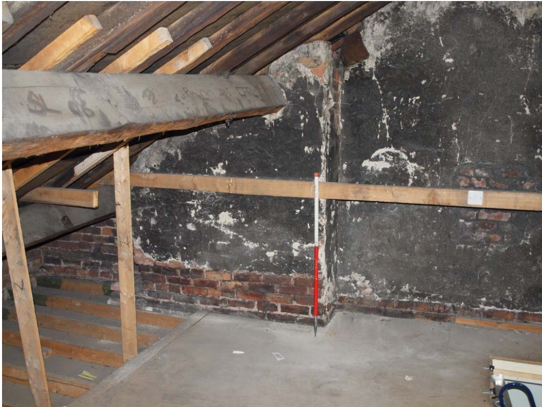
Plate 21: Detail of western chimney breast
