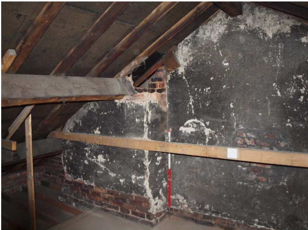
Plate 24: Western chimney breast showing it supporting purlin
