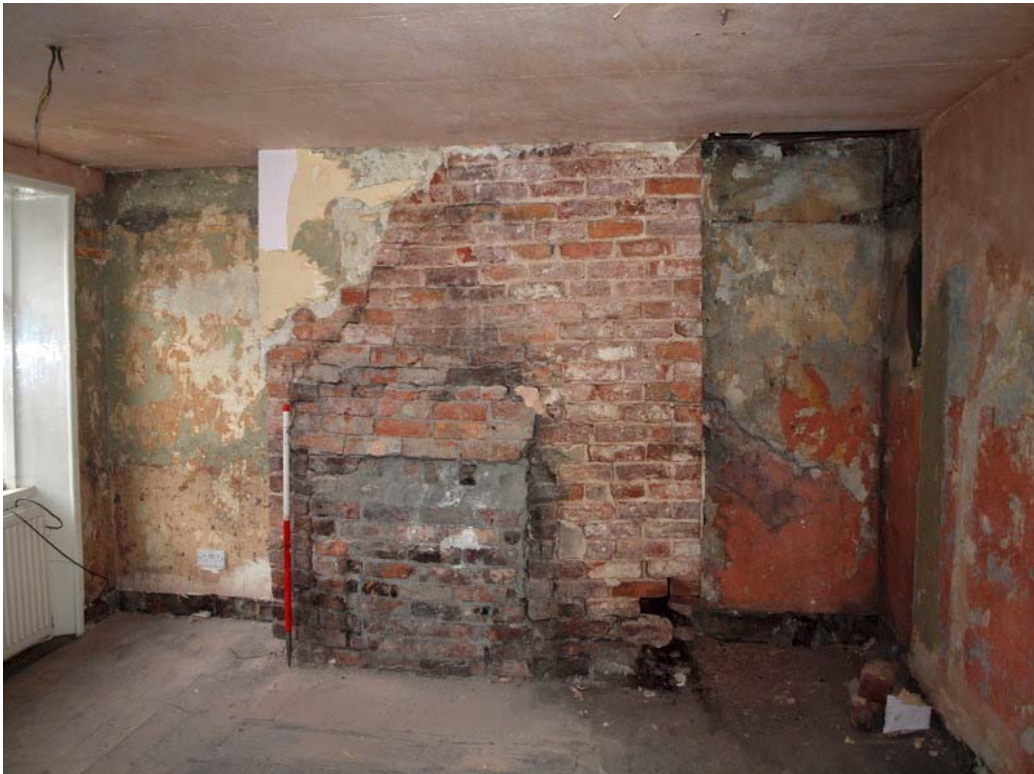
Plate 29: Chimney breast in room 6 after uncovering blocked fireplace
