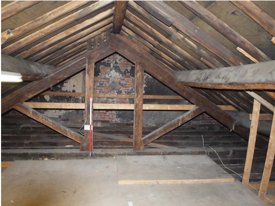
Plate 23: Southern end of attic showing roof truss
