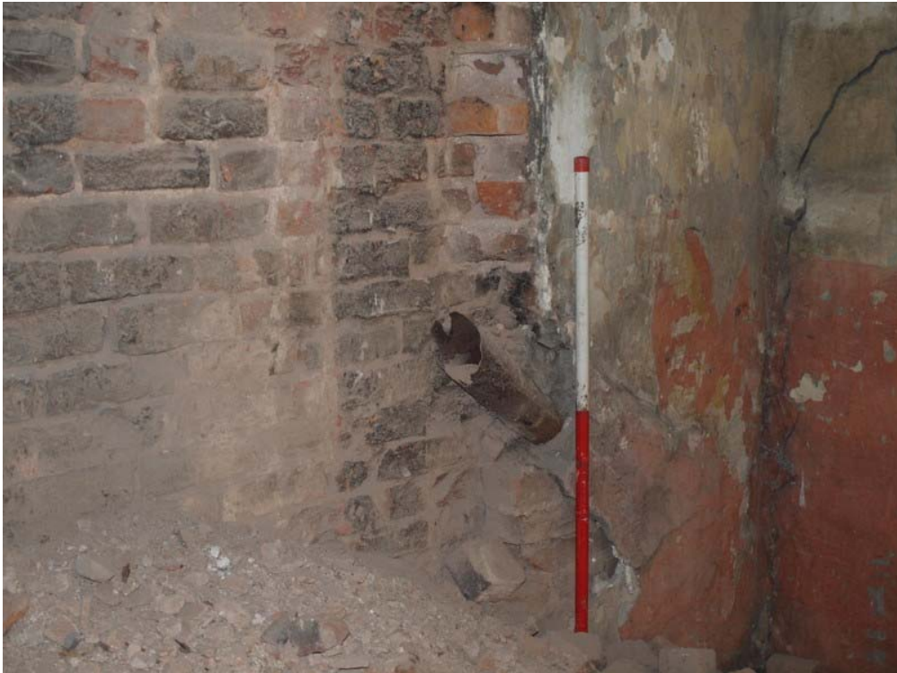
Plate 31: Detail of metal pipe in chimney breast in room 6
