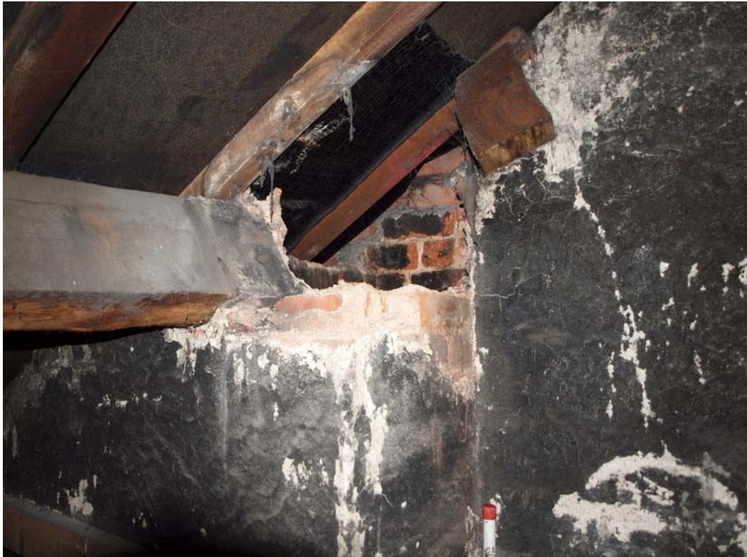
Plate 25: Detail of western chimney breast showing it supporting purlin
