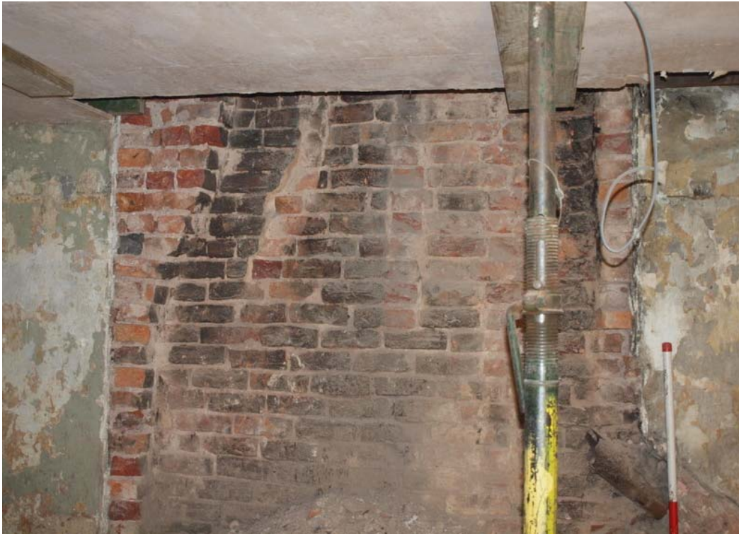
Plate 33: Detail of flue curve in room 6
