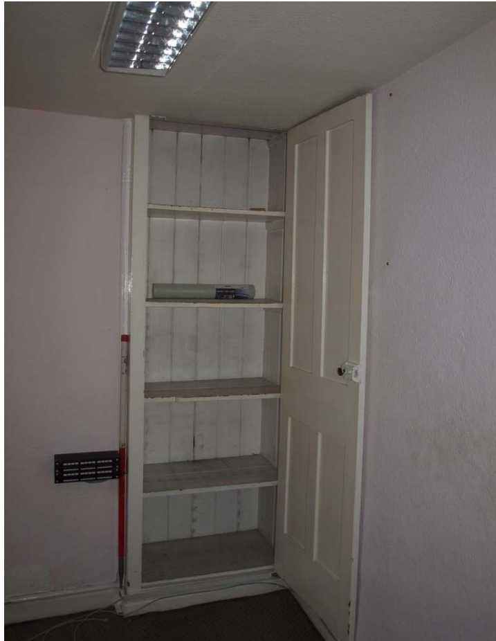
Plate 17: Detail of cupboard in room 6
