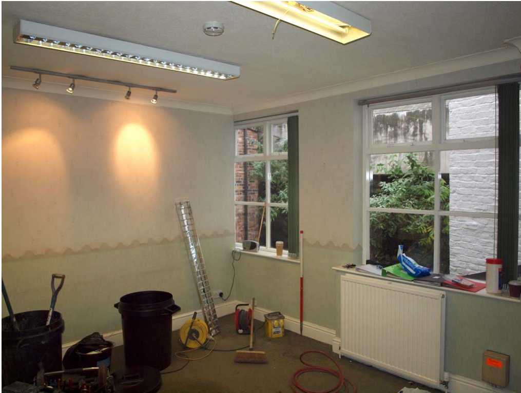
Plate 3: Room 1 looking north-east towards rear of property
