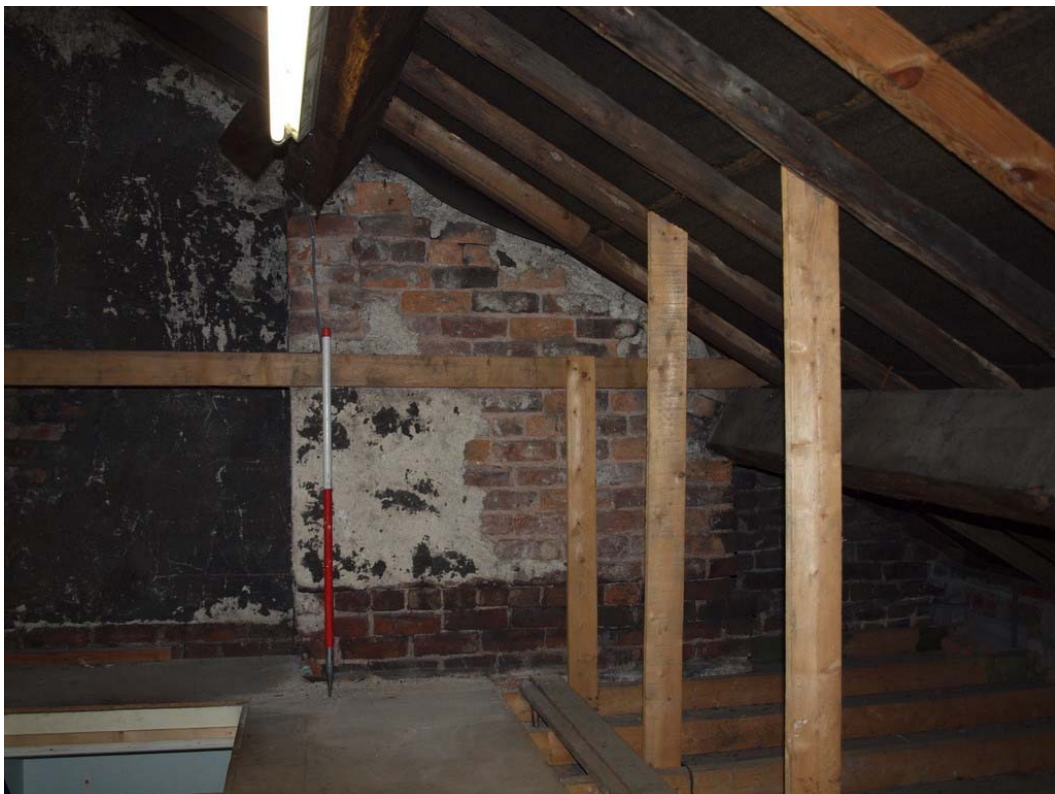
Plate 22: Eastern chimney breast
