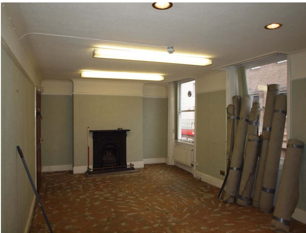
Plate 4: Room 2 looking south-west
