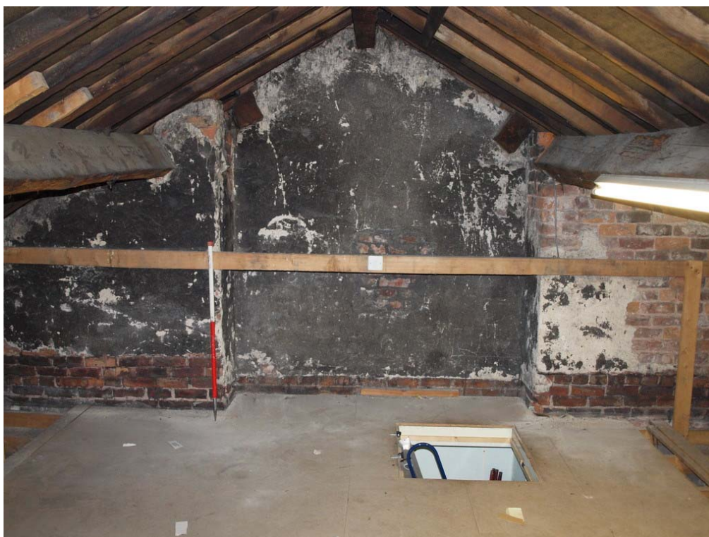
Plate 20: Attic looking north east showing chimney breasts to be removed
