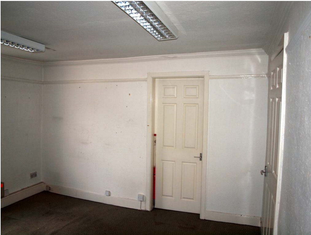
Plate 13: Room 5 looking north-east
