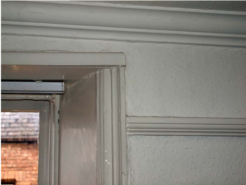
Plate 15: Detail of cornice, picture rail and door surround
