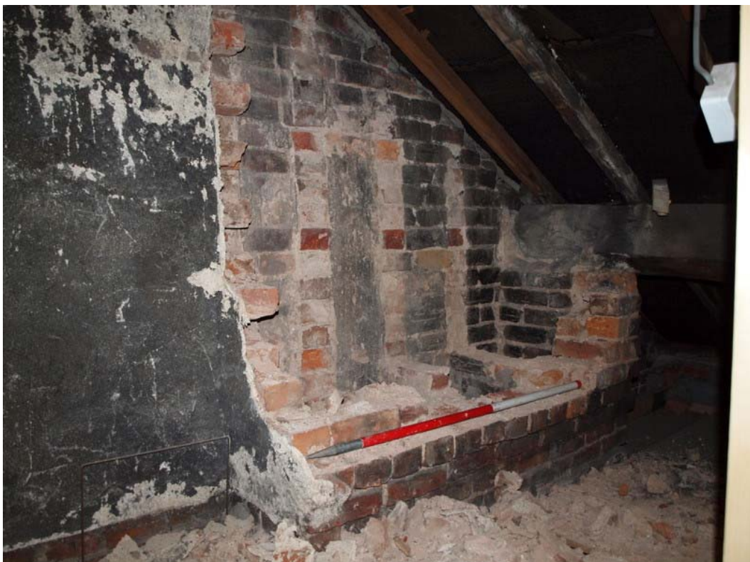
Plate 28: Eastern chimney breast after removal
