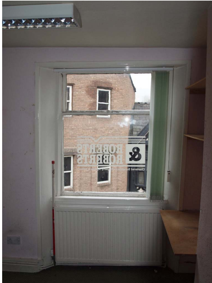
Plate 19: Detail of sash window in west wall of room 6
