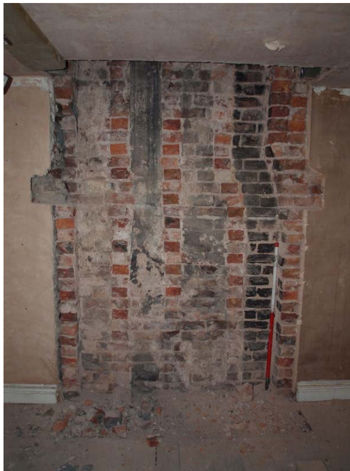
Plate 34: Room 4 after removal of chimney breast
