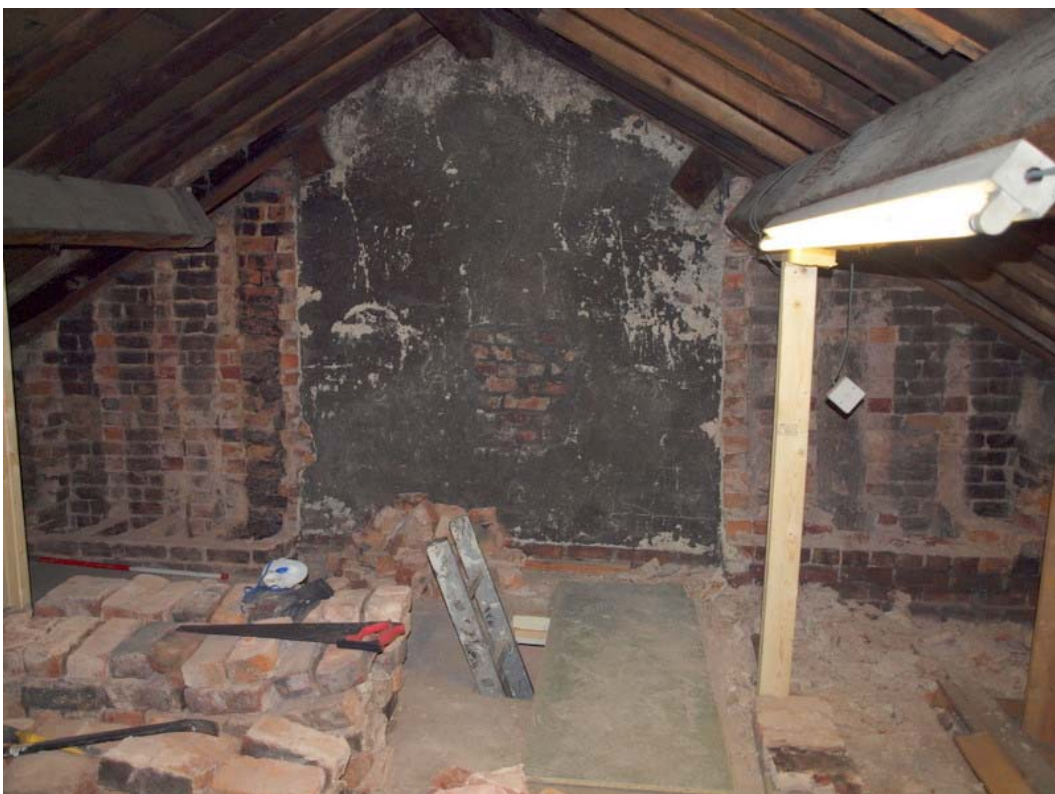
Plate 26: Attic after removal of both chimney breasts
