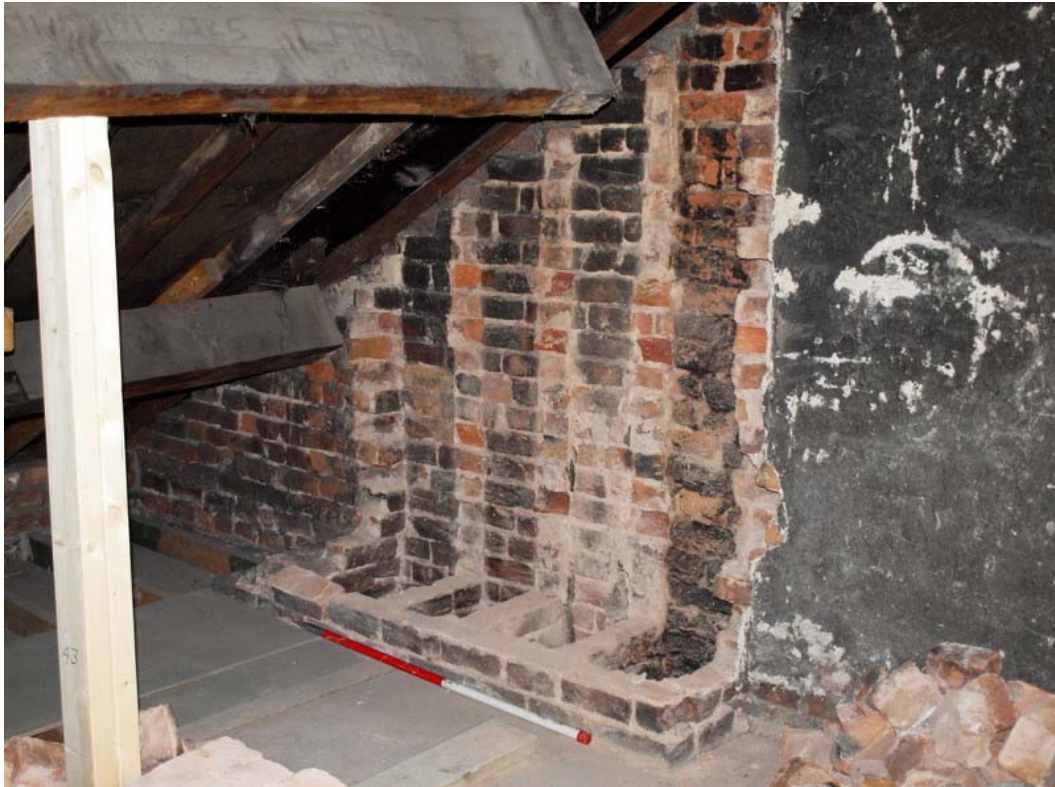
Plate 27: Western chimney breast after removal
