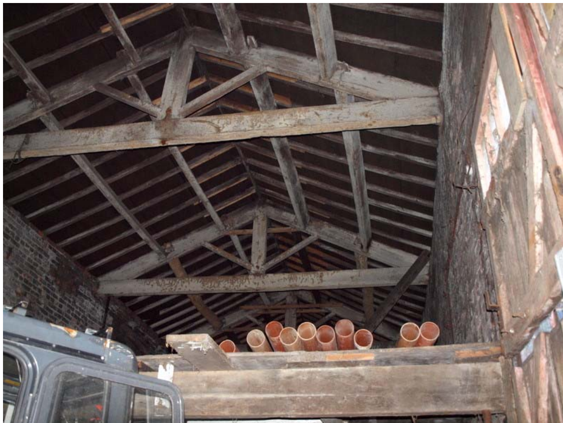
Plate 28: Machine cut timber king post trusses and line of first floor
