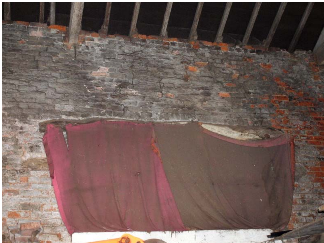
Plate 26: Covered hand cut timber lintel of east barn door
