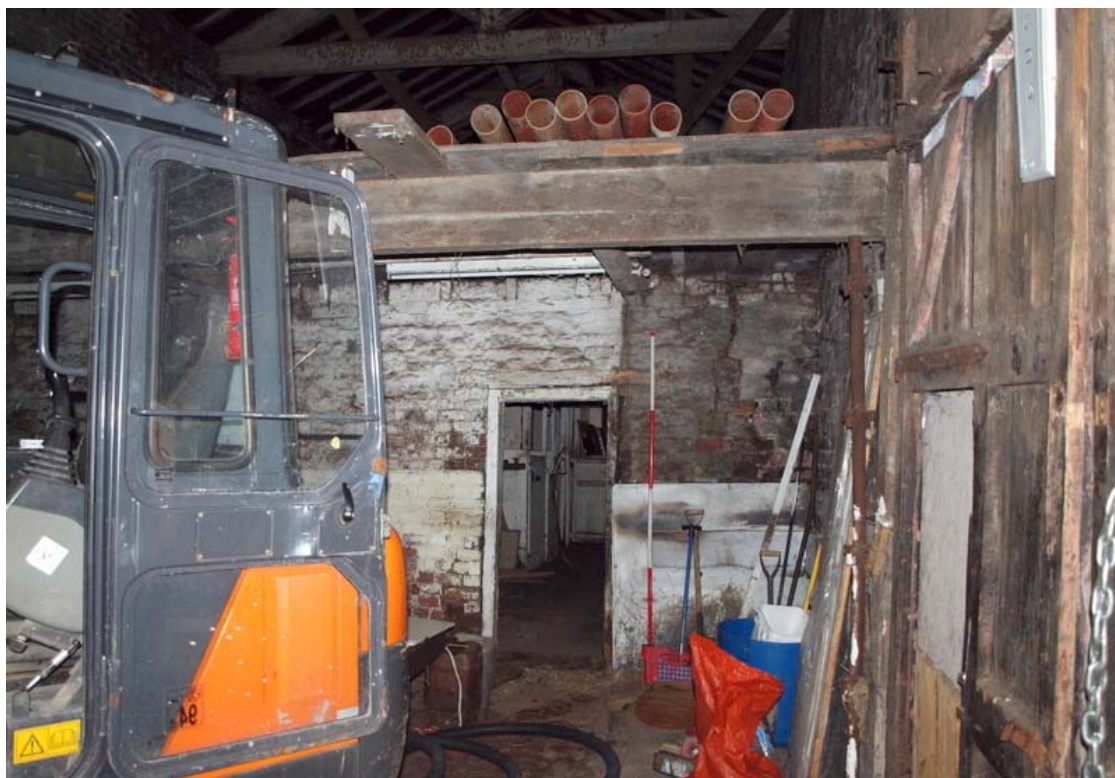
Plate 25: Internal wall in barn
