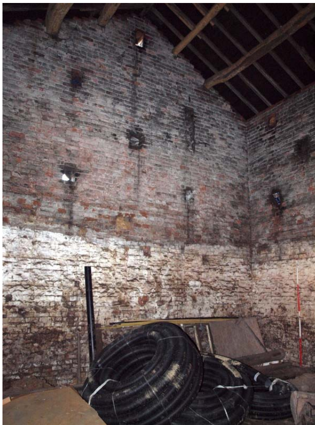
Plate 24: North end of barn
