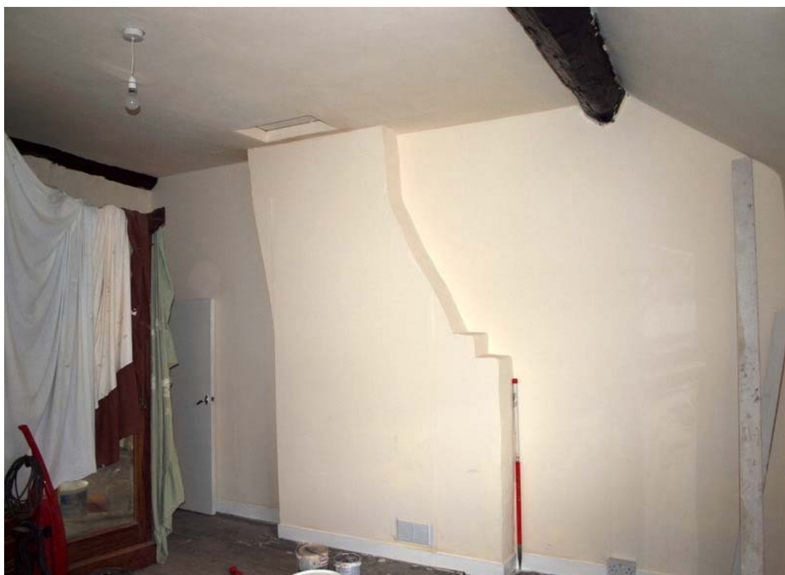
Plate 20: Chimney breast in room 5 of cottage
