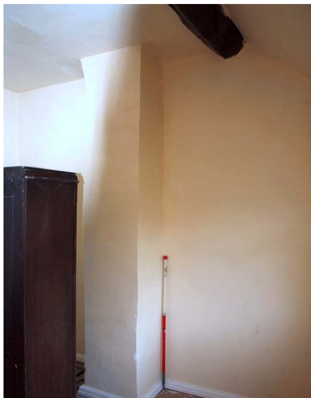
Plate 22: Chimney breast in room 6 of cottage
