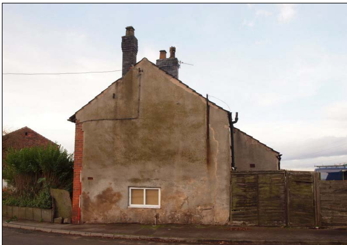
Plate 4: East elevation of cottage
