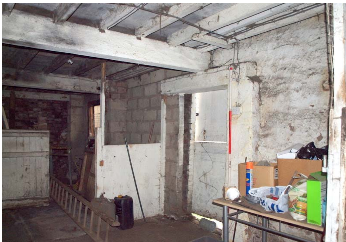
Plate 31: Loading door and rebuilt concrete block wall to the south
