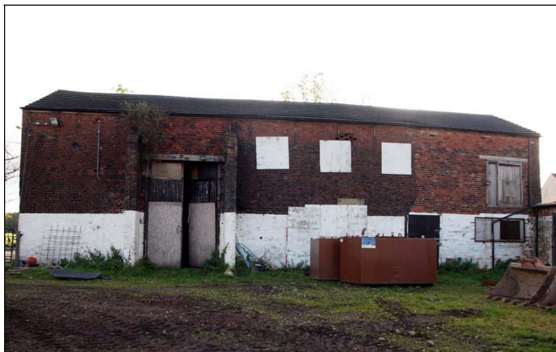
Plate 6: West elevation of barn
