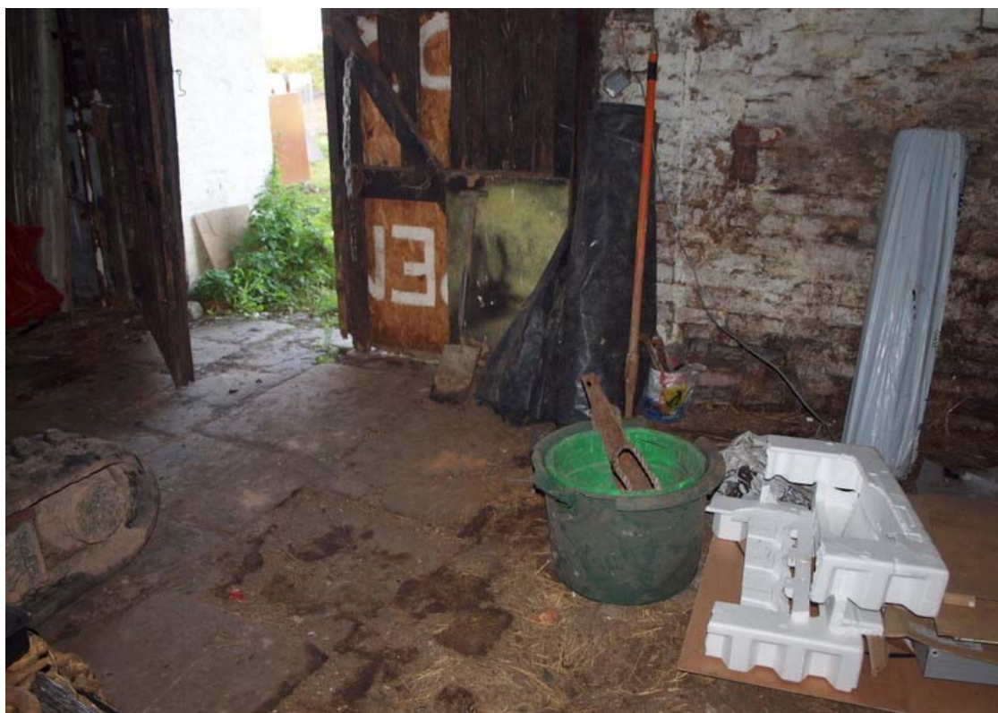
Plate 27: Flag surface with cobbles to the north
