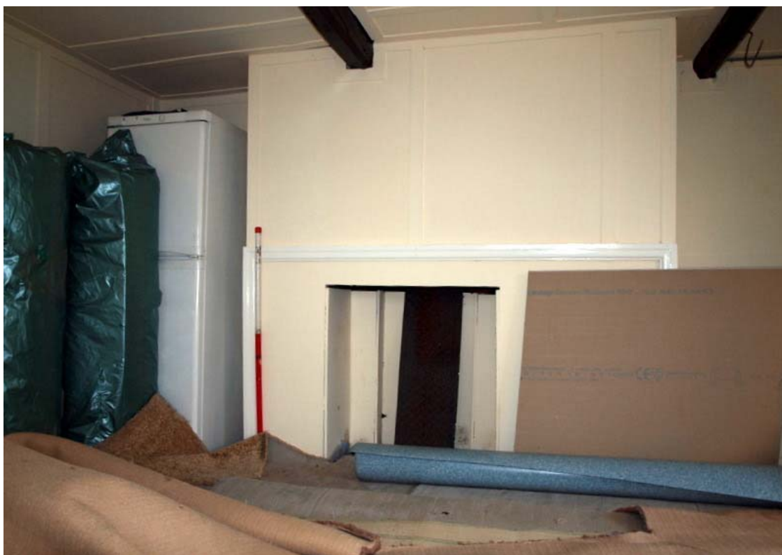
Plate 12: Cottage Room 1 Fireplace
