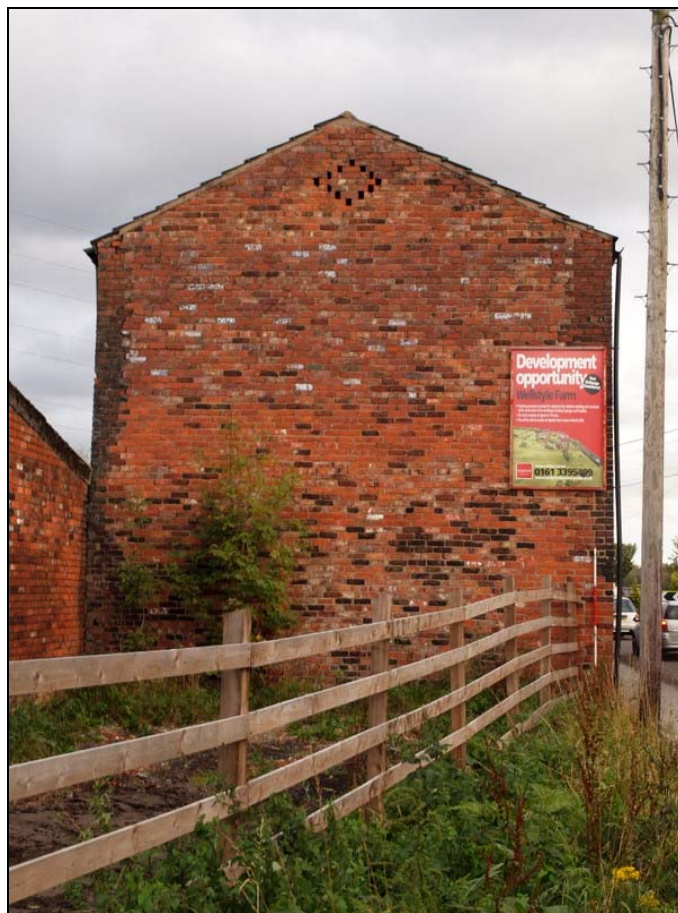
Plate 5: South elevation of barn
