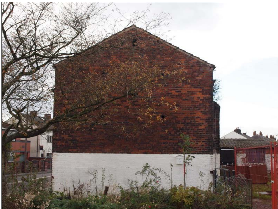
Plate 7: North elevation of barn
