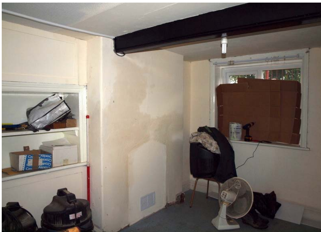
Plate 13: Cottage Room 2 Fireplace
