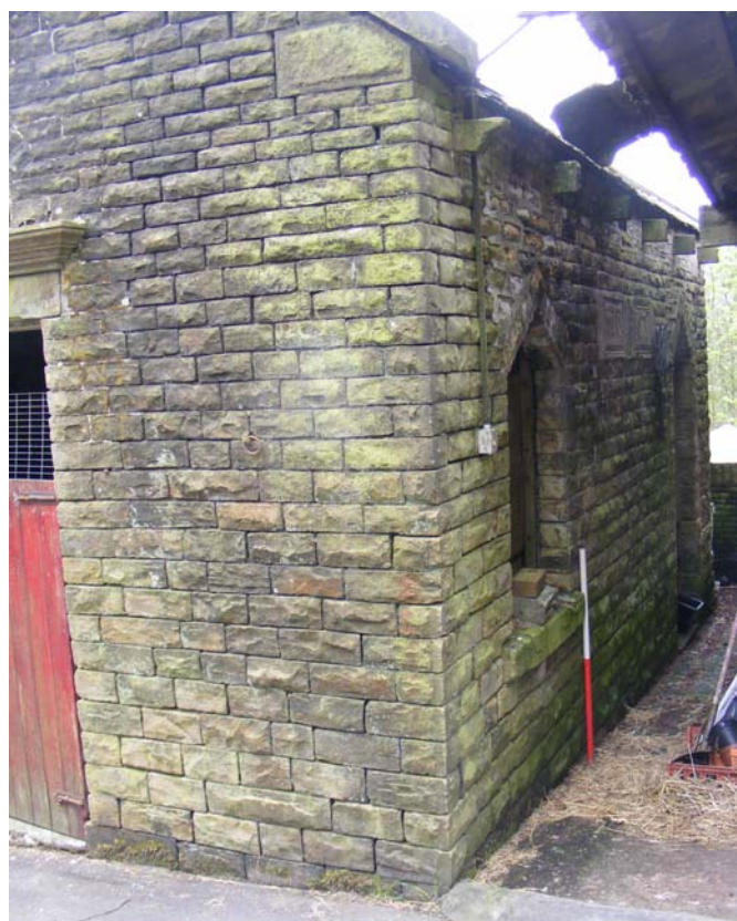
Plate 10: South Elevation of Subject Building
