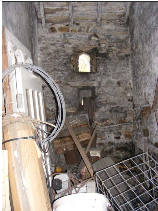
Plate 18: Interior of East Cell from South
