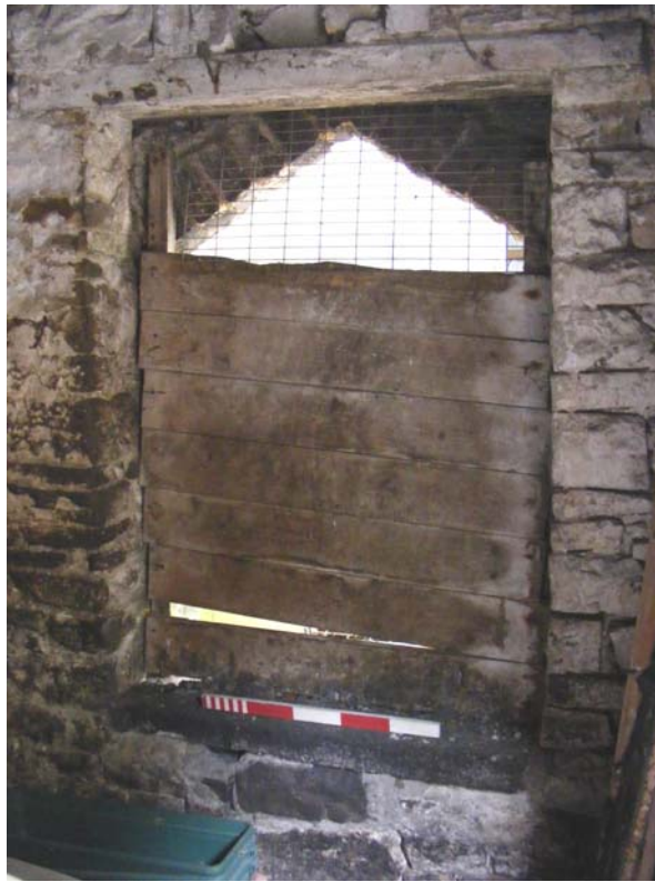
Plate 17: Window in south Wall of West Cell
