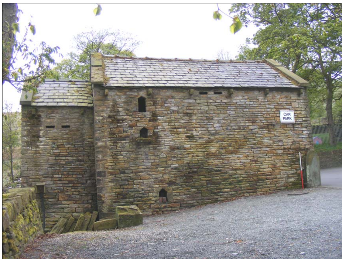
Plate 7: North Elevation of Subject Building
