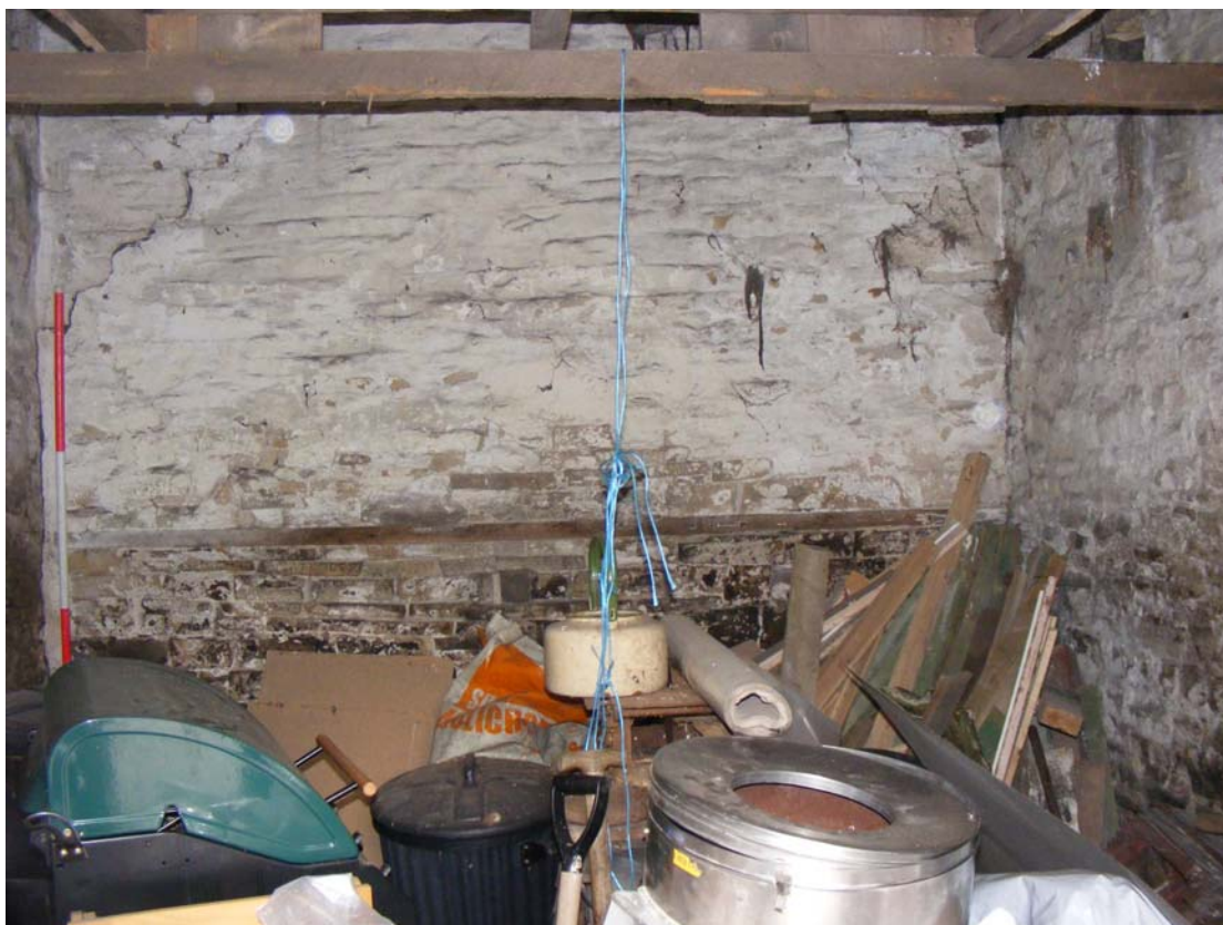
Plate 16: Interior of West Cell from West
