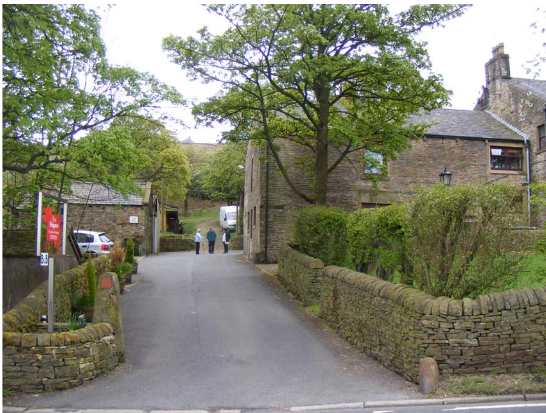
Plate 5: Freestanding Subject Building east of Farmhouse and Barn
