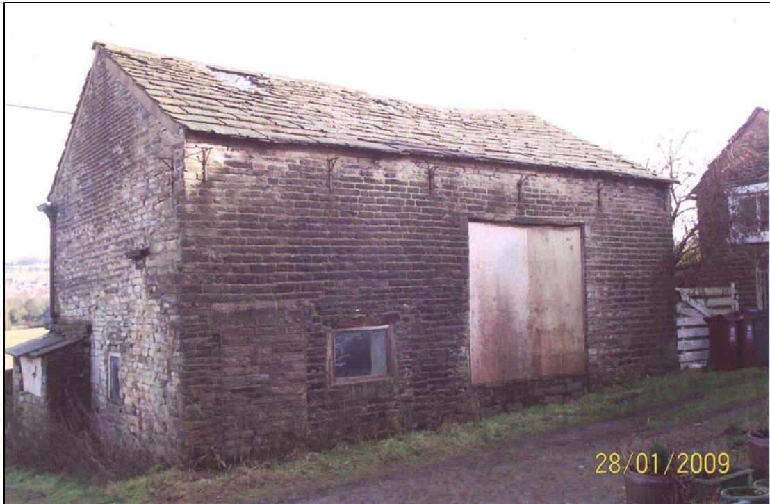
Plate 7: South-west elevation, taken 28/1/09. Courtesy of Trevor Jones.
