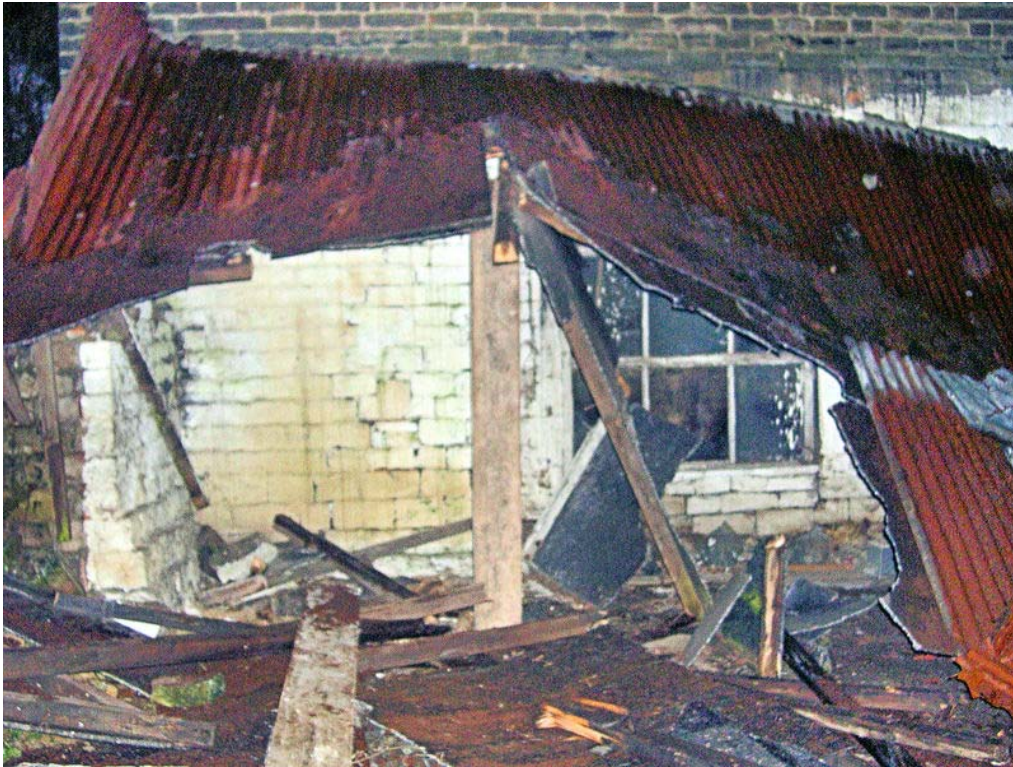
Plate 11: Window in north-east wall, taken 10/1/11. Courtesy of Trevor Jones.
