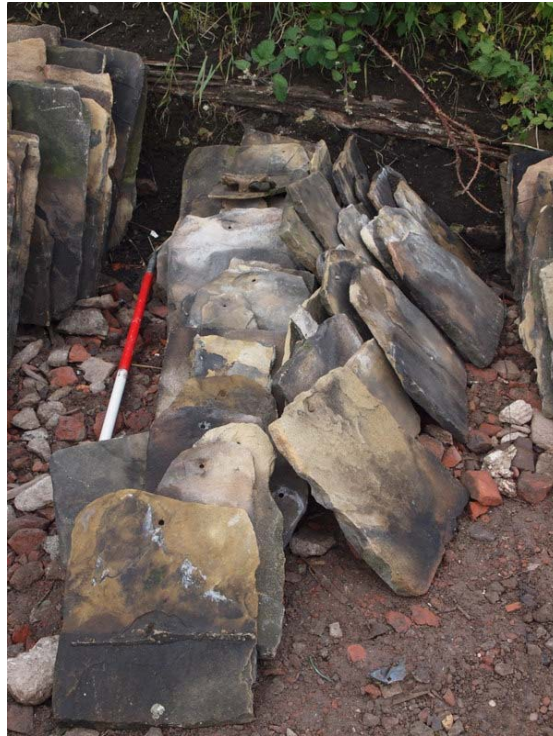
Plate 5: Sandstone roof slabs
