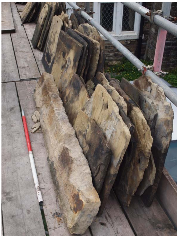
Plate 39: Sandstone roof slabs
