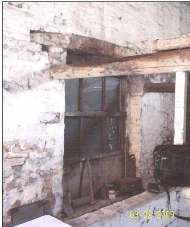
Plate 18: Interior showing window (former barn door) with hand-cut timber lintel in north-eastern wall. Provided by R. Schofield.
