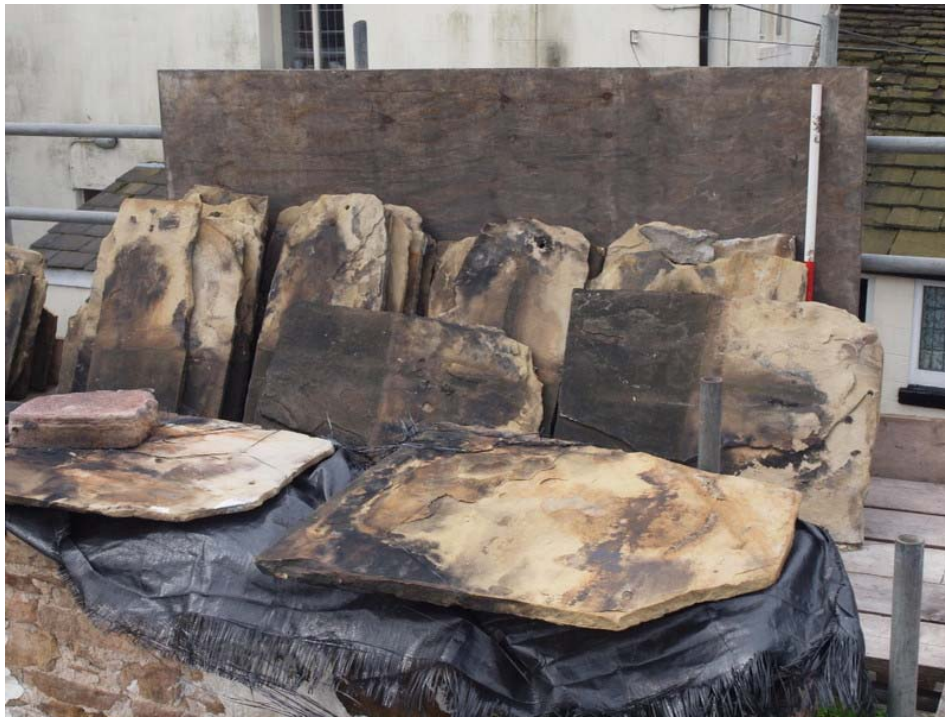
Plate 37: Sandstone roof slabs
