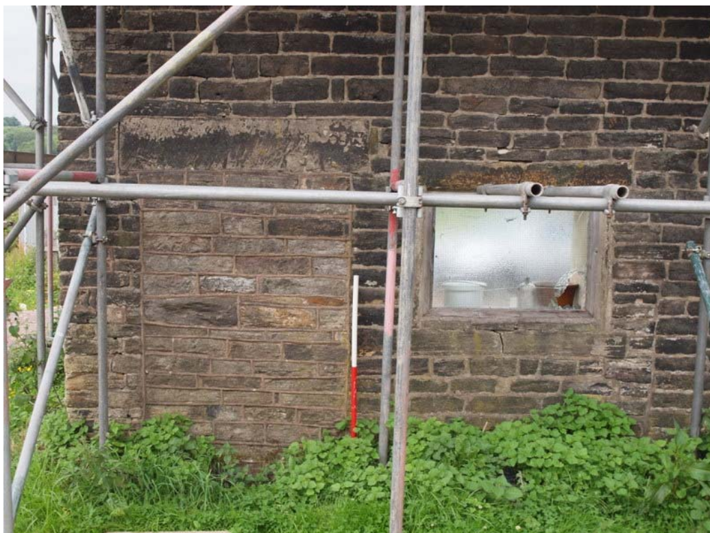
Plate 6: Detail of window and blocked doorway in south-west elevation
