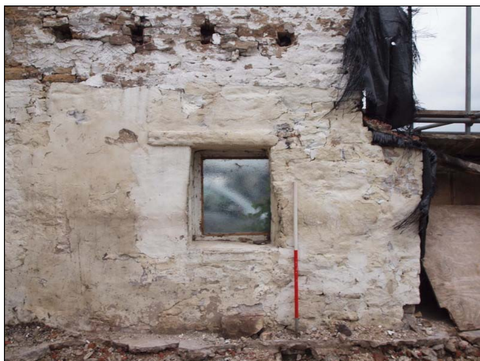
Plate 16: Window in north-west wall.
