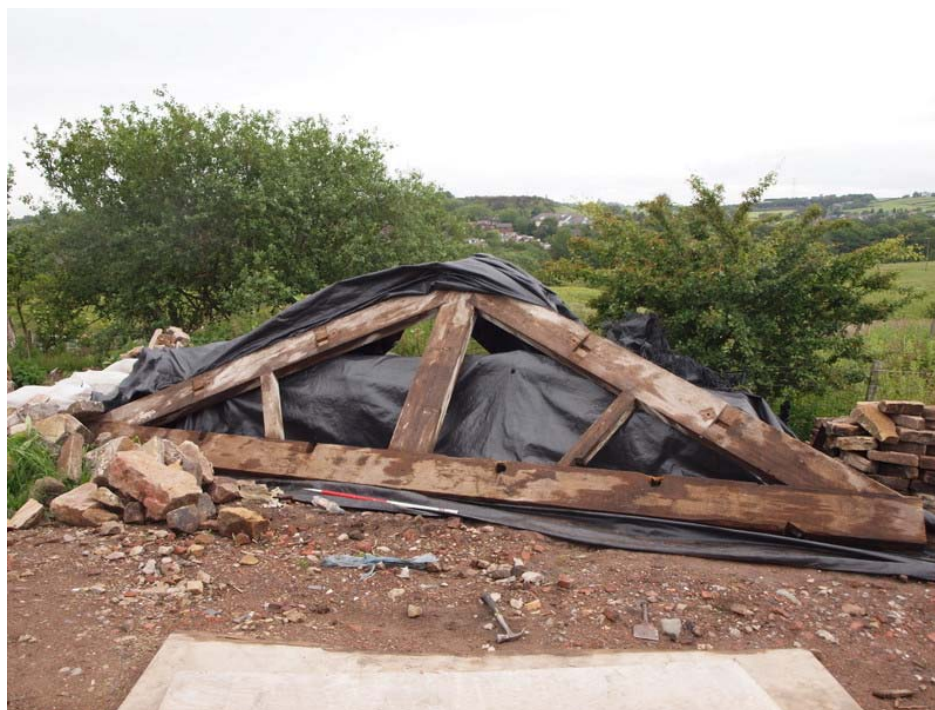
Plate 12: King post roof truss
