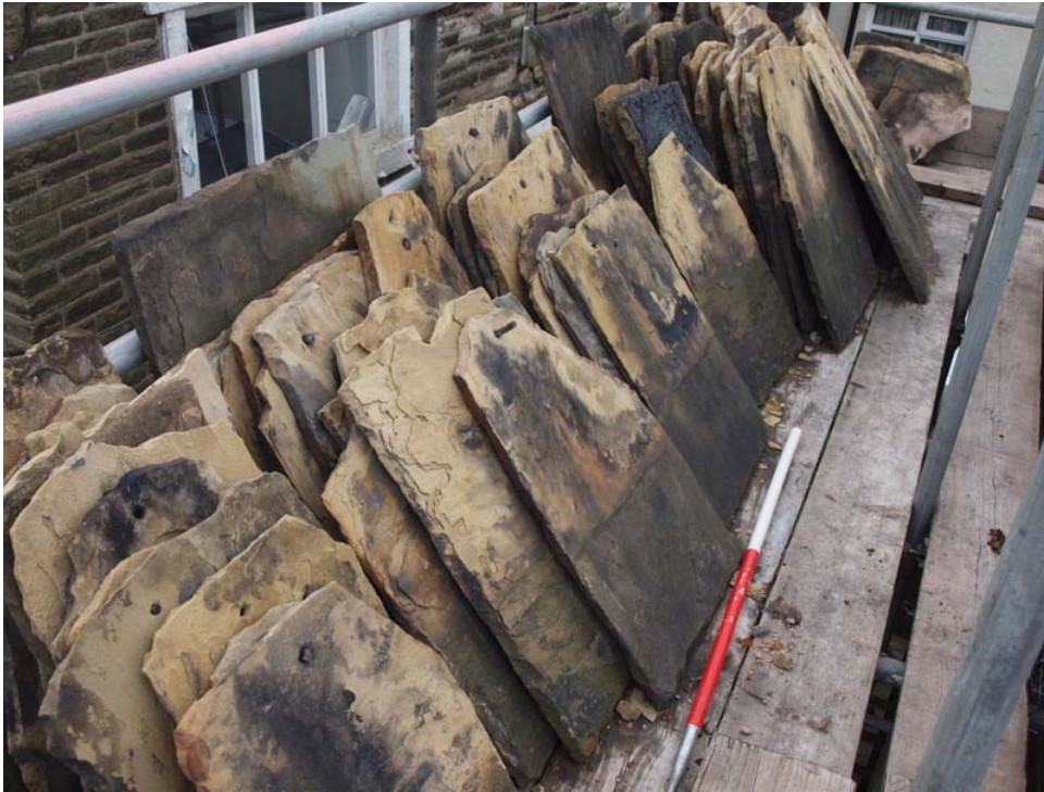
Plate 43: Sandstone roof slabs
