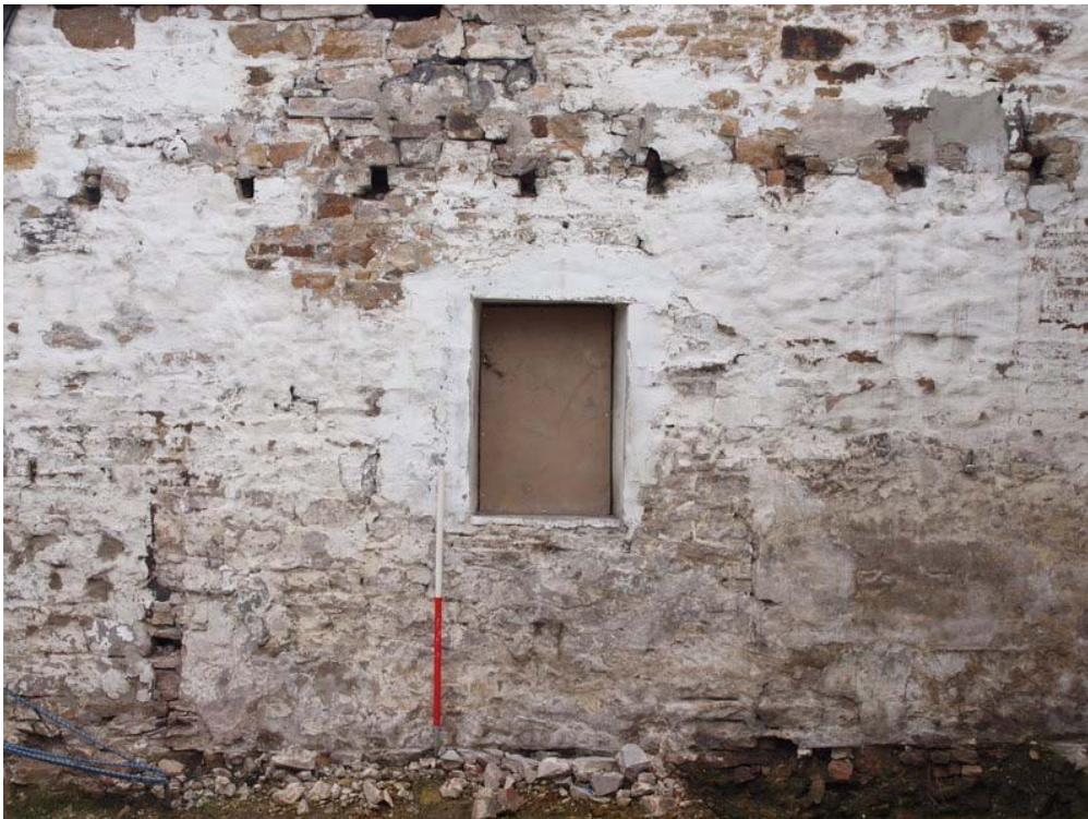
Plate 13: blocked window in south-east wall
