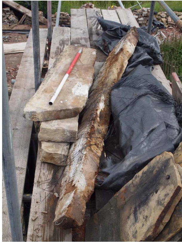
Plate 45: Handcut timber lintel
