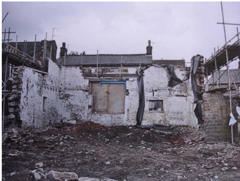
Fig.2: Condition of barn following partial demolition
