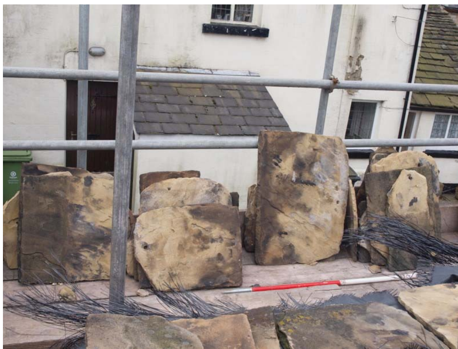
Plate 40: Sandstone roof slabs
