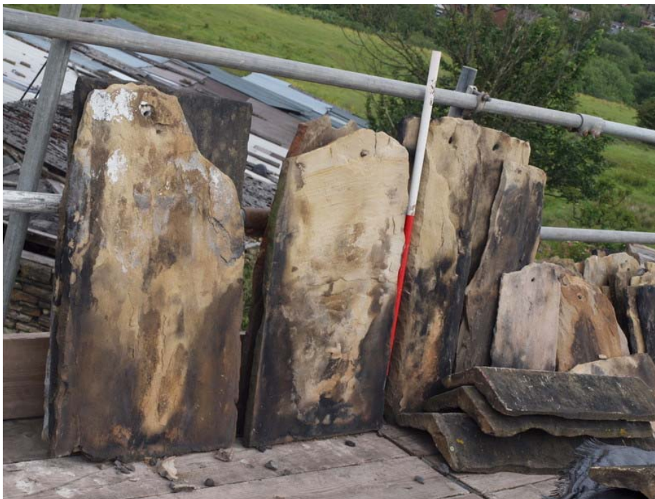
Plate 36: Sandstone roof slabs
