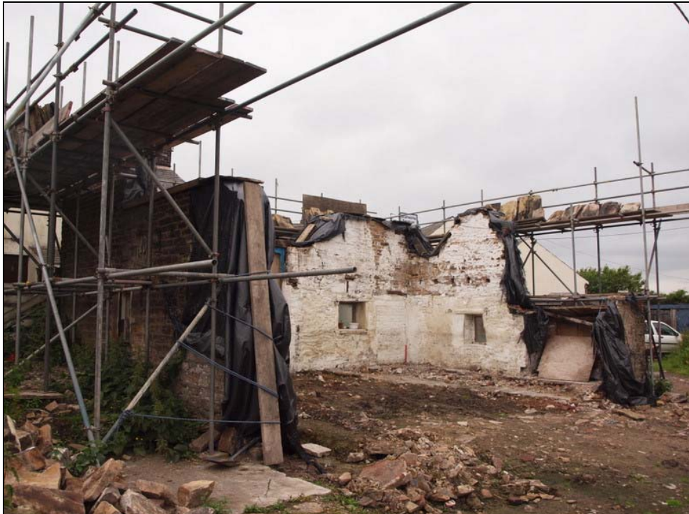
Plate 12: Interior view towards south-west corner
