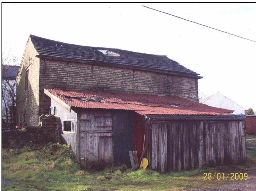
Plate 9: North-east elevation, taken 28/1/09. Courtesy of Trevor Jones.
