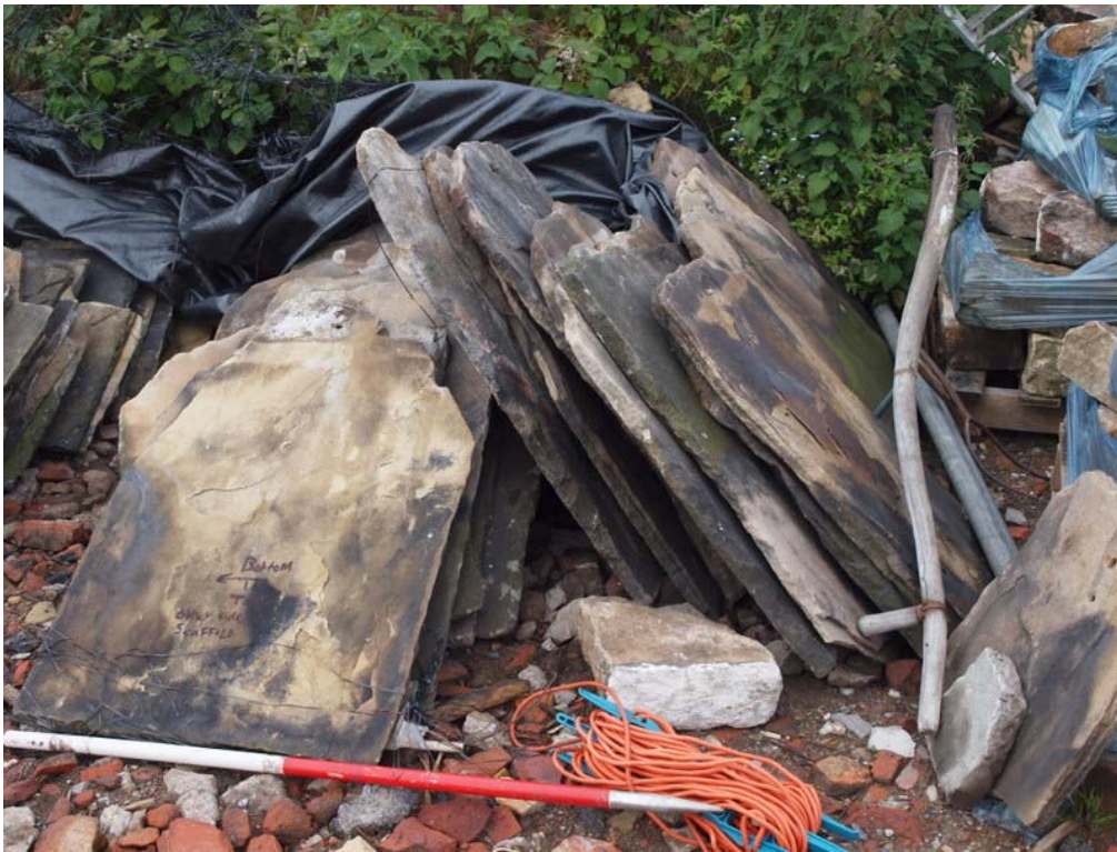
Plate 1: Sandstone roof slabs
