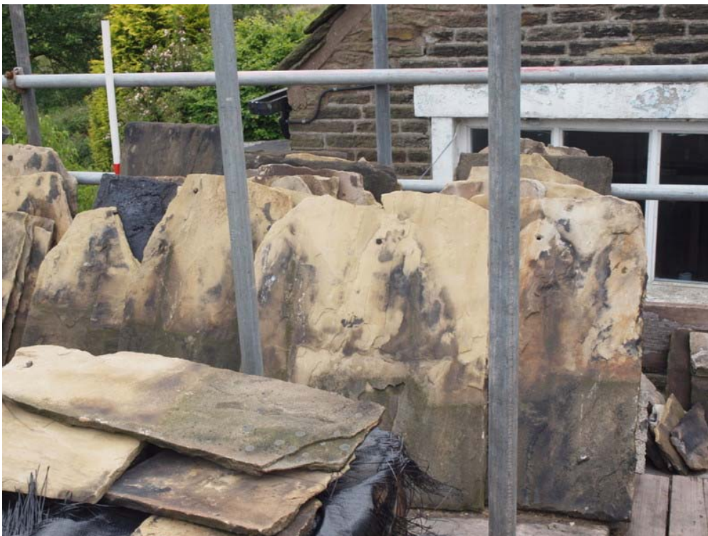
Plate 42: Sandstone roof slabs
