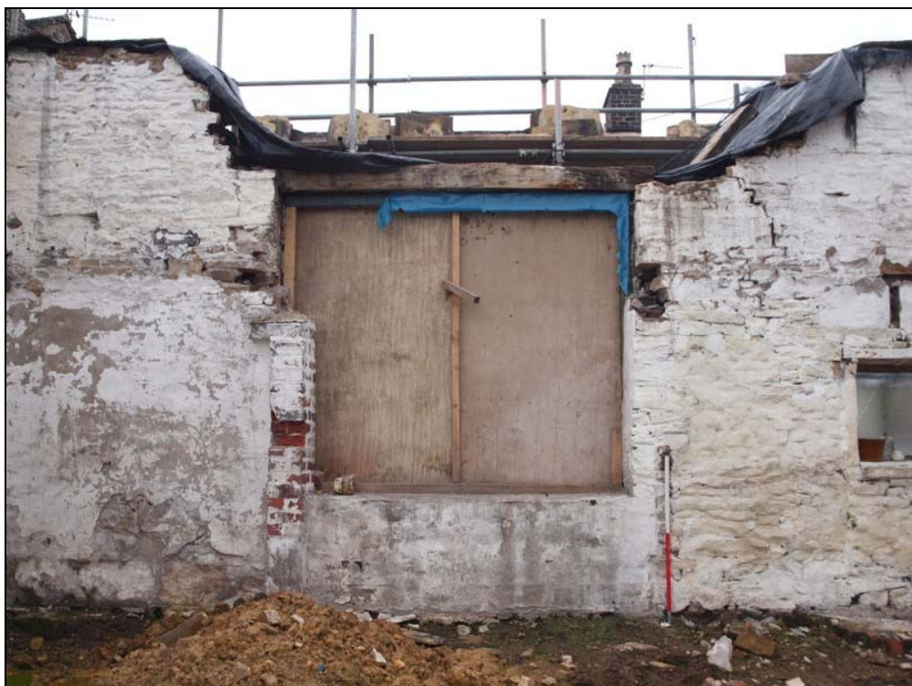
Plate 14: barn door in south-west wall, blocked at the bottom
