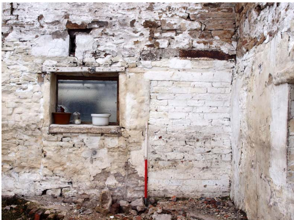
Plate 15: Window and blocked doorway at north end of south-west wall
