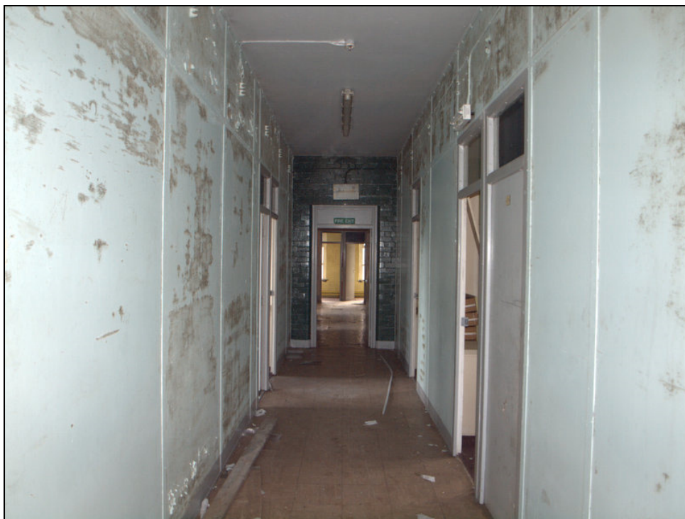
Plate 30: First floor corridor
