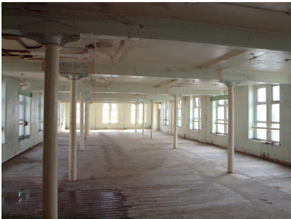
Plate 56: West block first floor after soft strip
