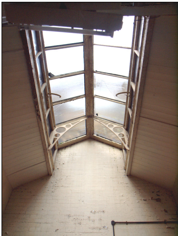
Plate 38: Skylight in roof of north office
