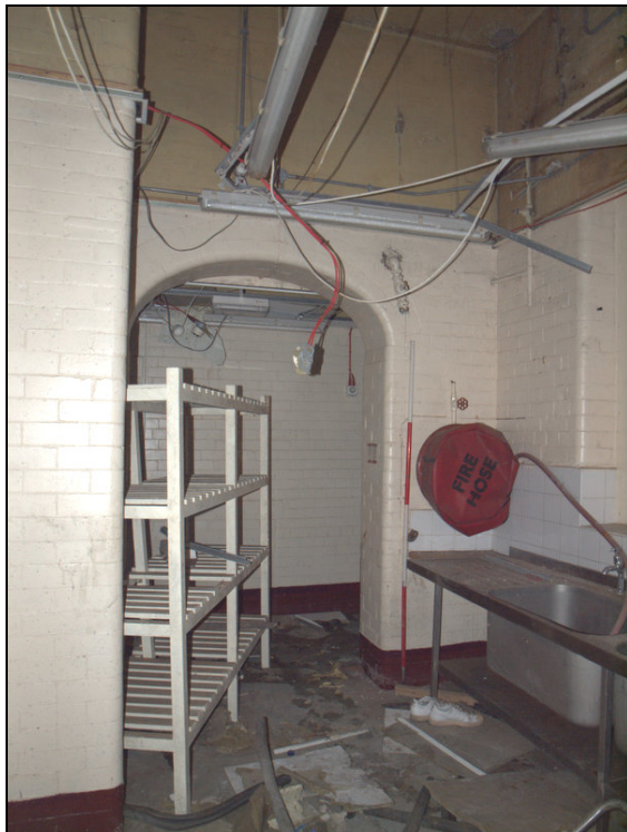
Plate 43: Arched opening to central area of north block
