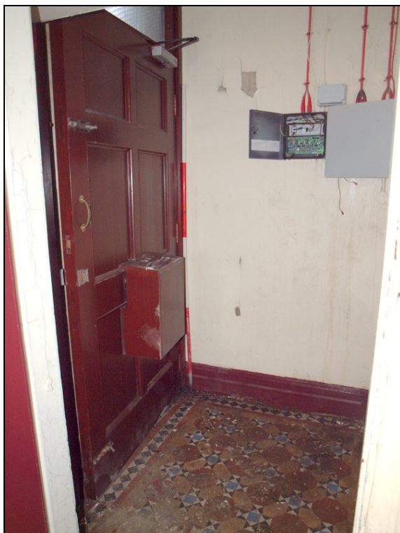
Plate 40: Tiled porch and doorway to exterior in southeast corner of atrium
