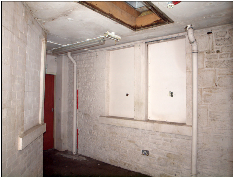
Plate 47: Angled corridor with blocked windows in east side of north block
