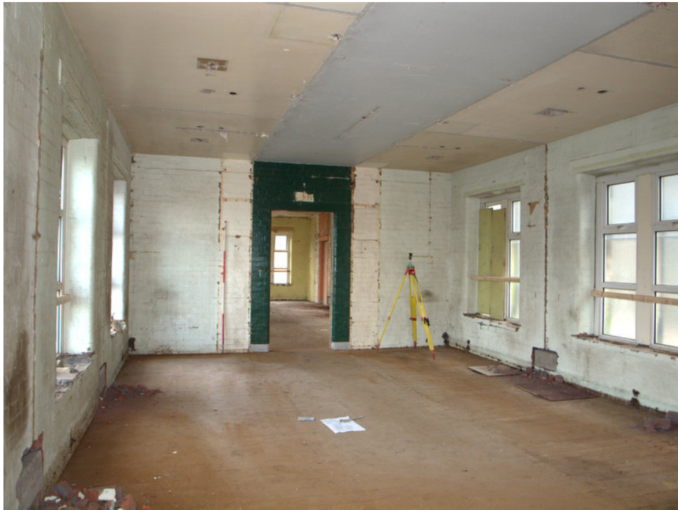
Plate 55: East block first floor, north end, after soft strip
