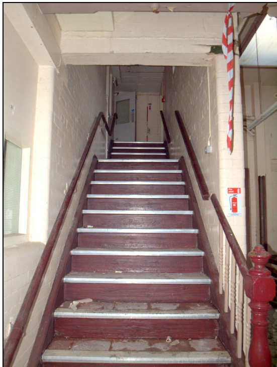
Plate 39: Staircase to first floor at south end of atrium
