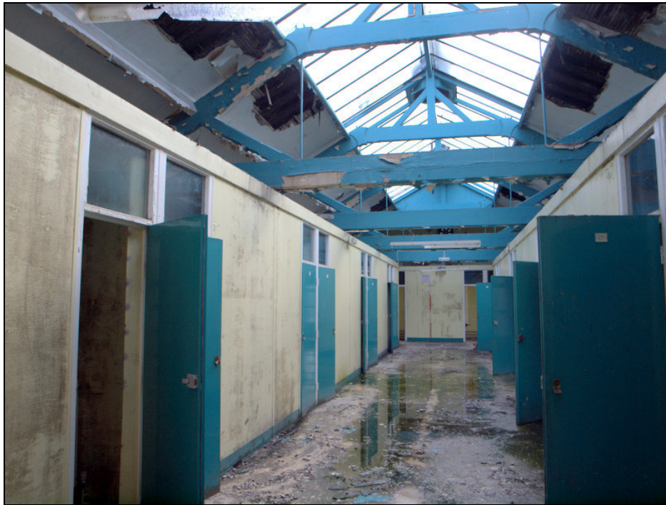
Plate 23: Second floor central corridor showing trusses
