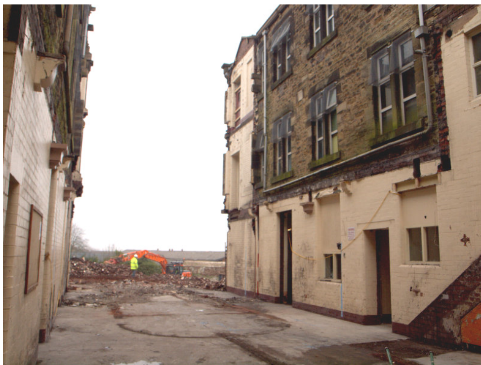
Plate 61: Site of atrium after removal
