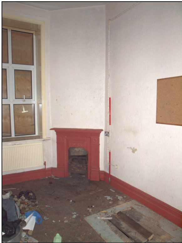
Plate 29: Northern room showing angled cast iron fireplace
