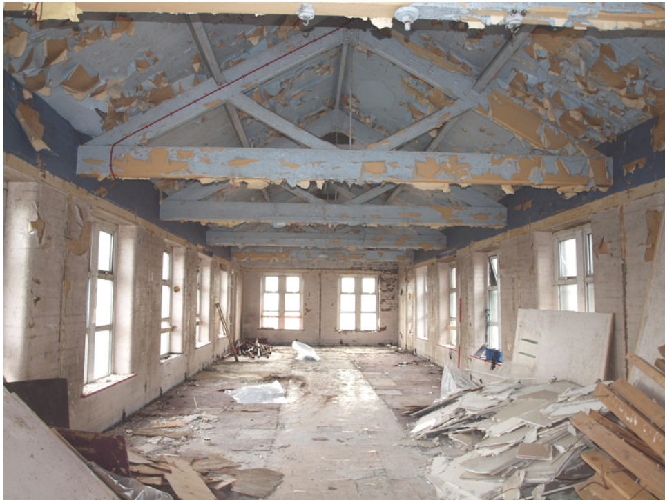
Plate 57: East block second floor after soft strip
