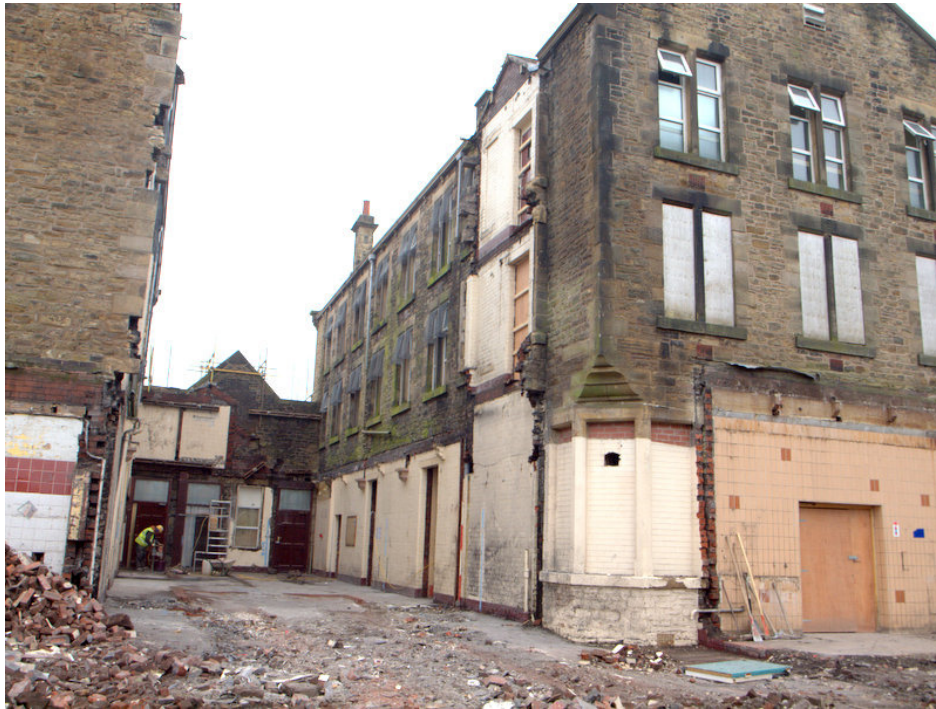
Plate 59: East elevation of west block after atrium removal
