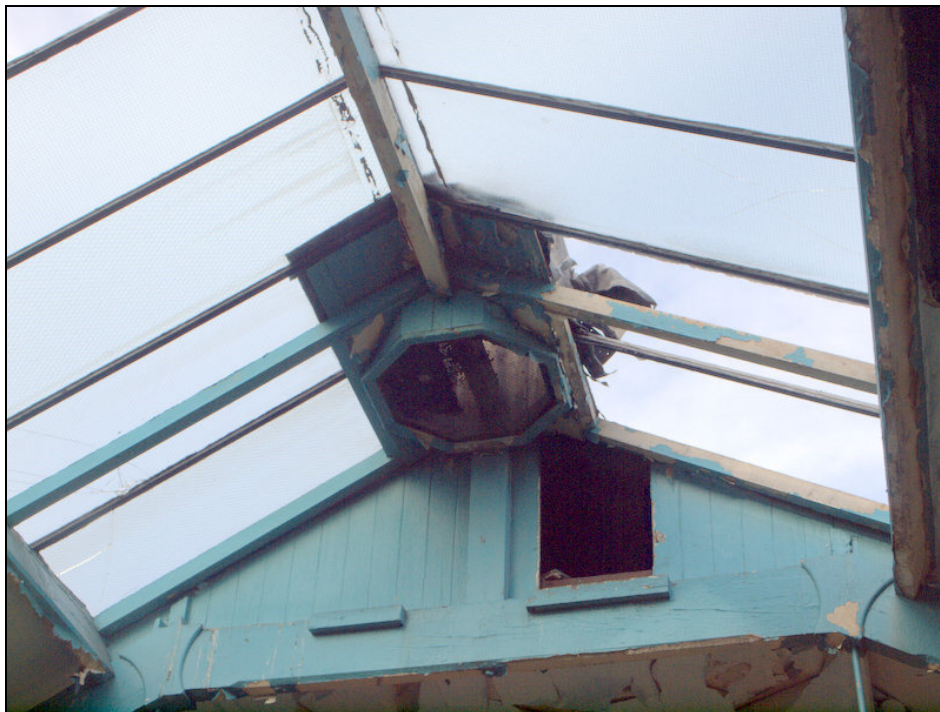
Plate 24: Attic space and vents at north end
