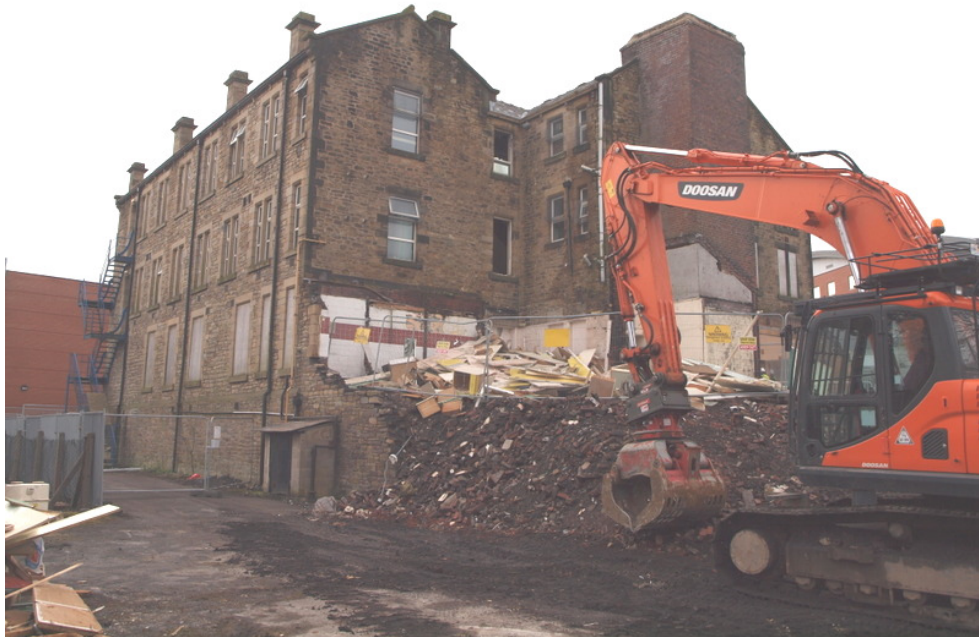
Plate 53: North elevation of east block after removal of north block
