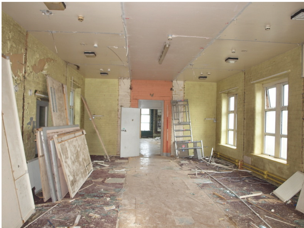
Plate 54: East block first floor, south end, after soft strip
