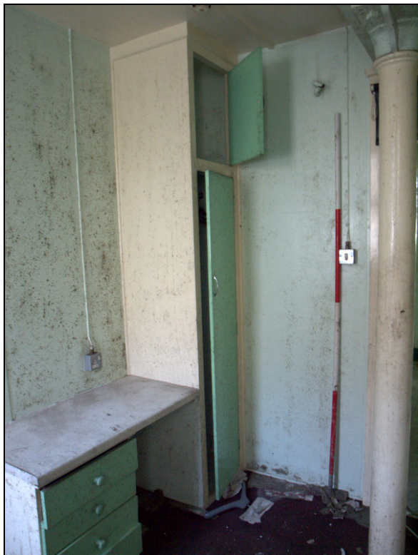
Plate 20: Interior of first floor room showing small wardrobe
