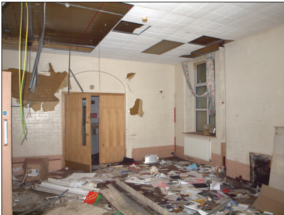
Plate 26: North side in ground floor of east block
