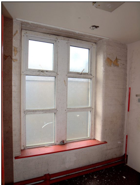
Plate 34: Room on second floor
