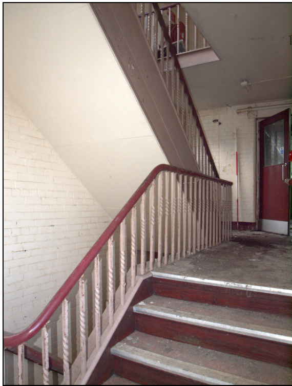
Plate 41: First floor staircase at north end of the atrium
