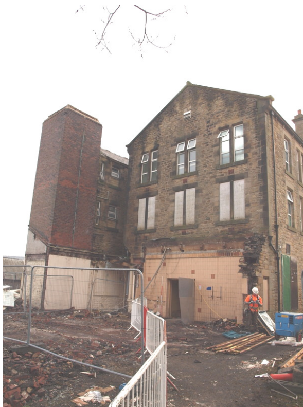
Plate 50: North elevation of West block after removal of north block
