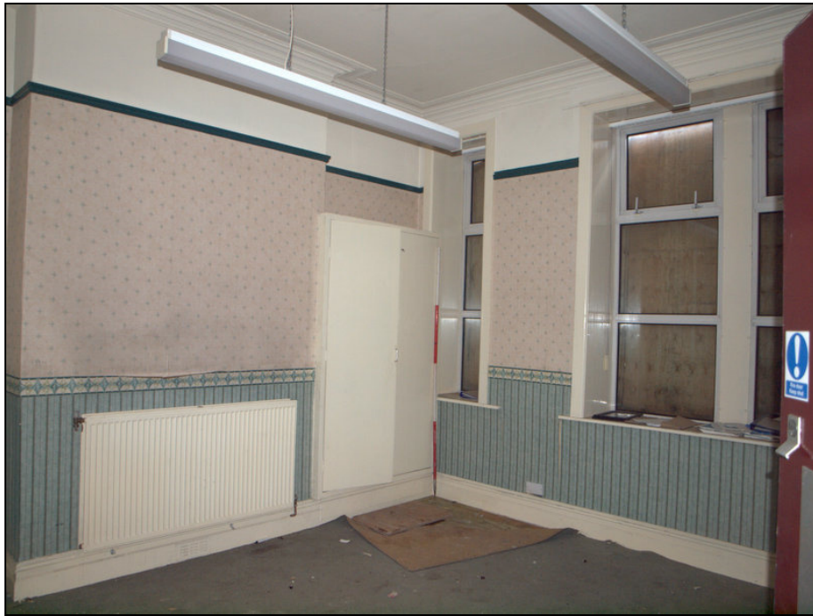
Plate 27: Southern room in south side of east block showing skirting, picture rail and cornice
