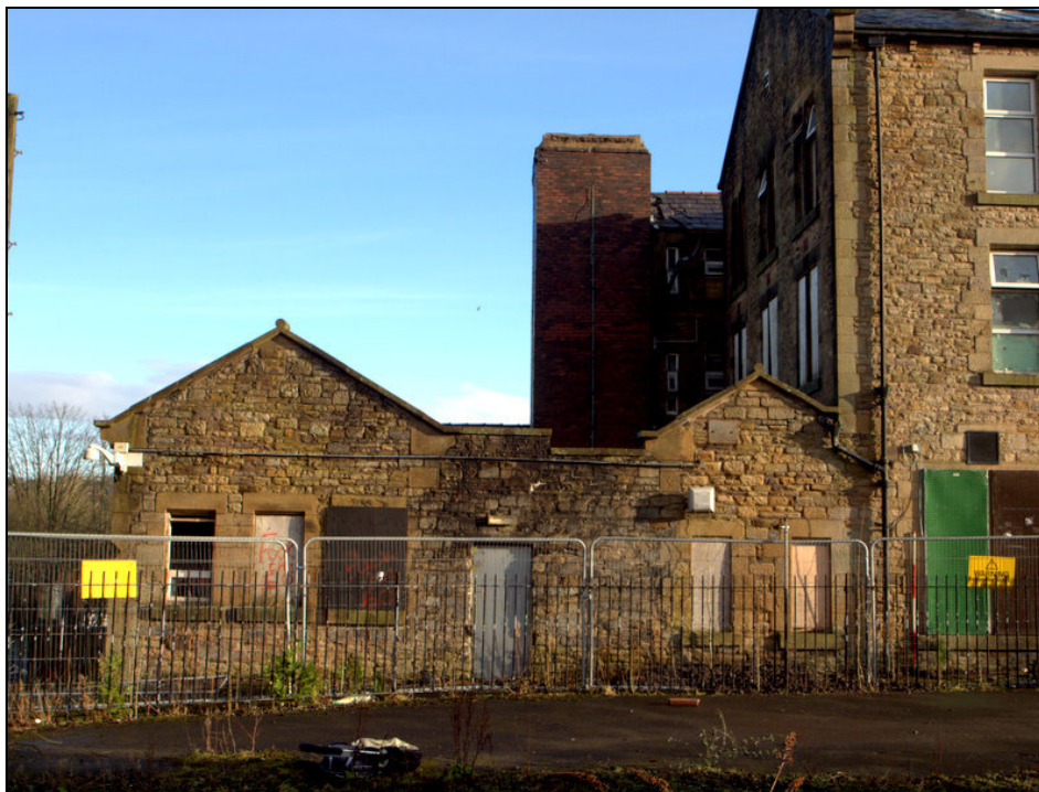
Plate 14: West elevation of the north block
