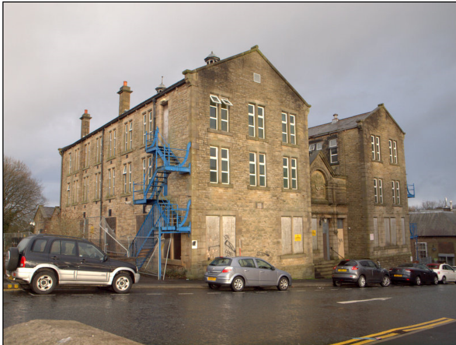
Plate 1: General shot of the building from the southwest
