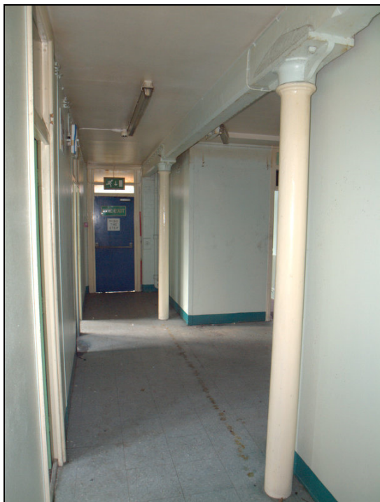
Plate 22: Stanchions supporting beam at southern end
