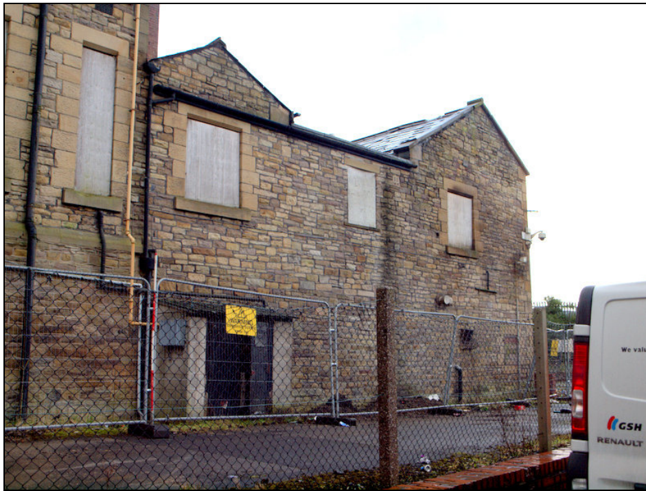
Plate 13: East elevation of the north block
