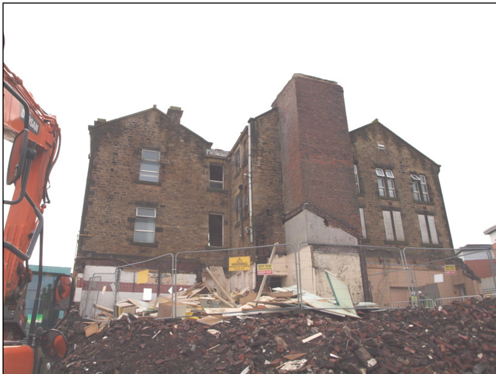
Plate 52: North elevation of building after removal of north block
