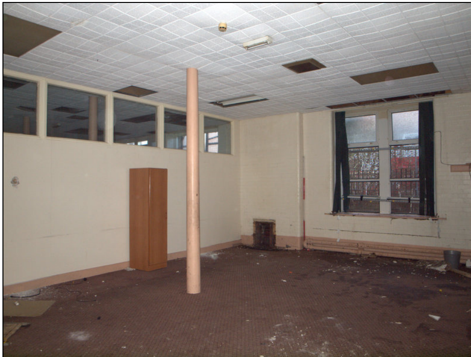
Plate 17: Central room showing fireplace in the west wall.
