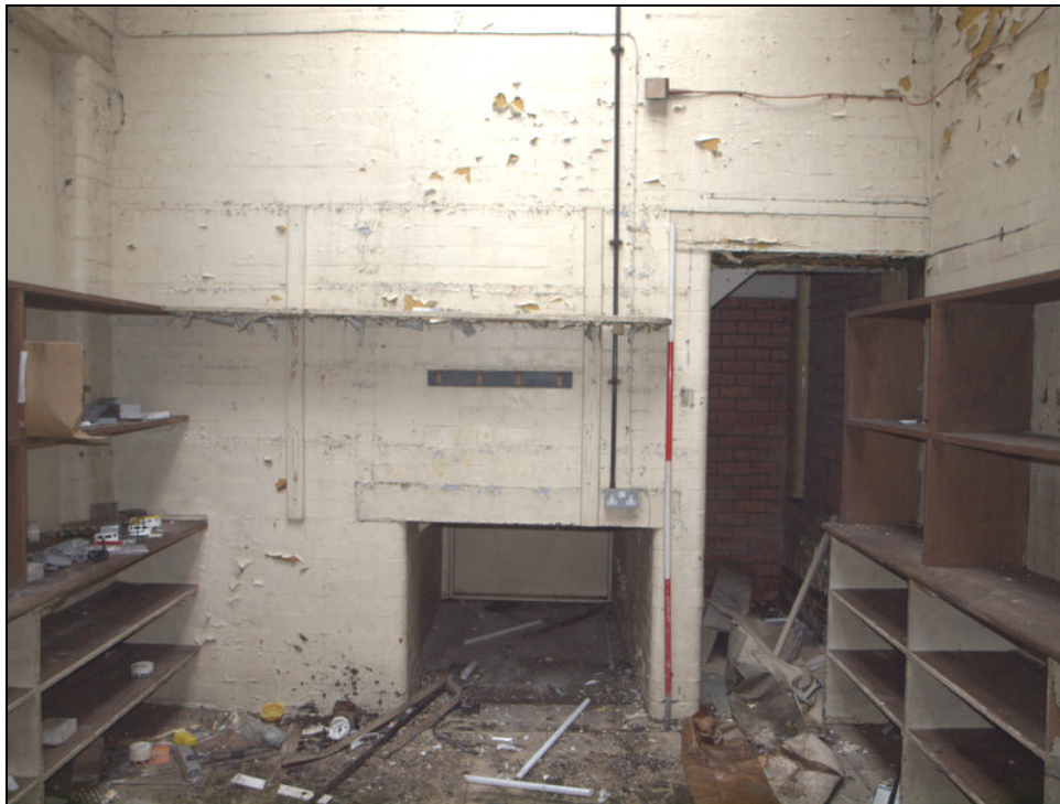
Plate 37: North room of office showing cupboards to the north
