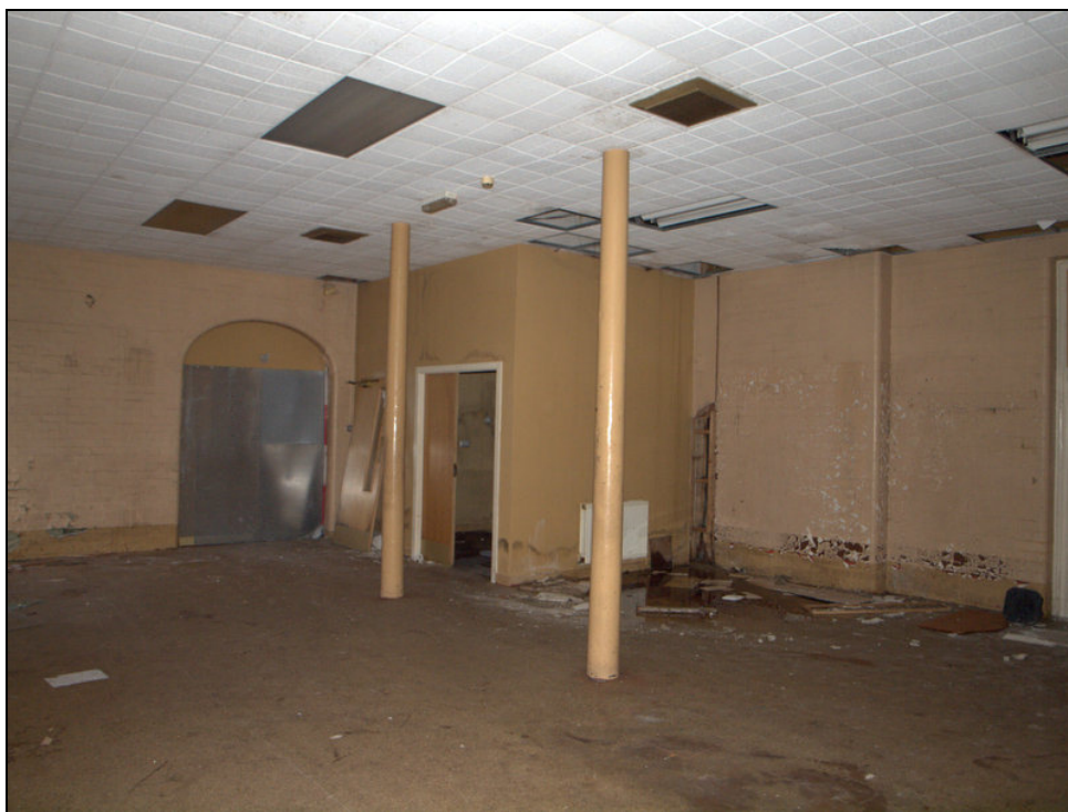
Plate 18: North room showing partition and doorway with arched lintel
