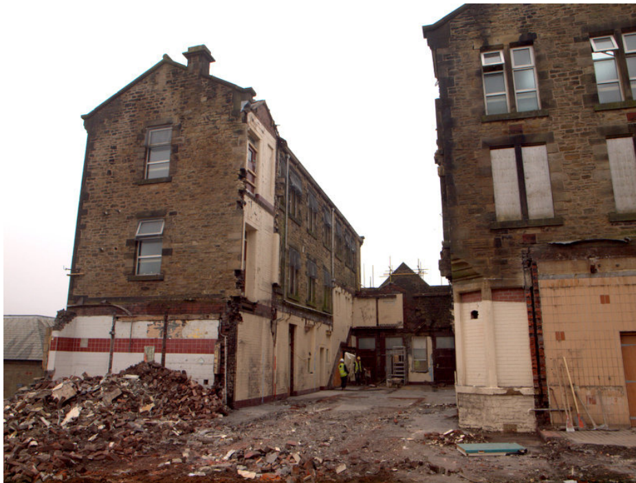
Plate 60: North end of building after removal of central atrium
