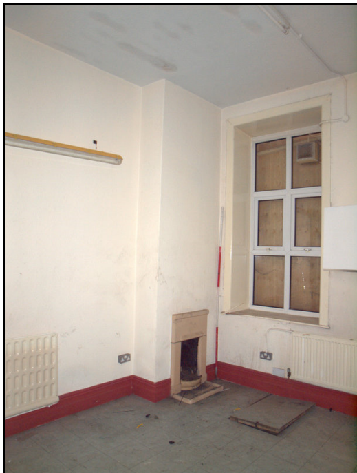
Plate 28: Central room in south side showing fireplace
