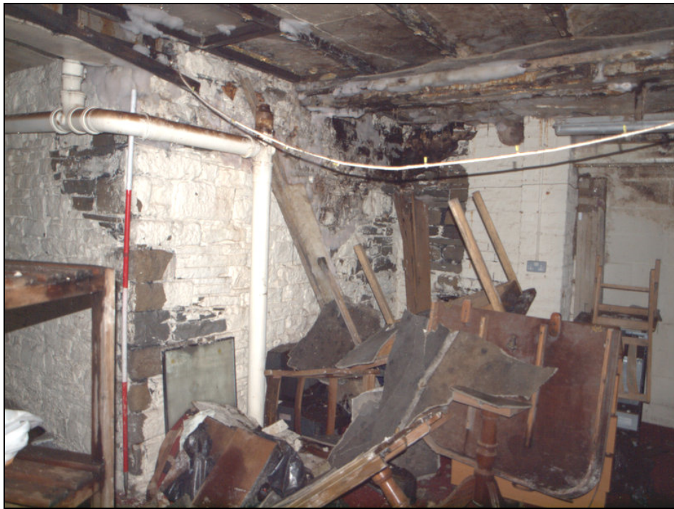
Plate 49: Basement showing stone wall construction
