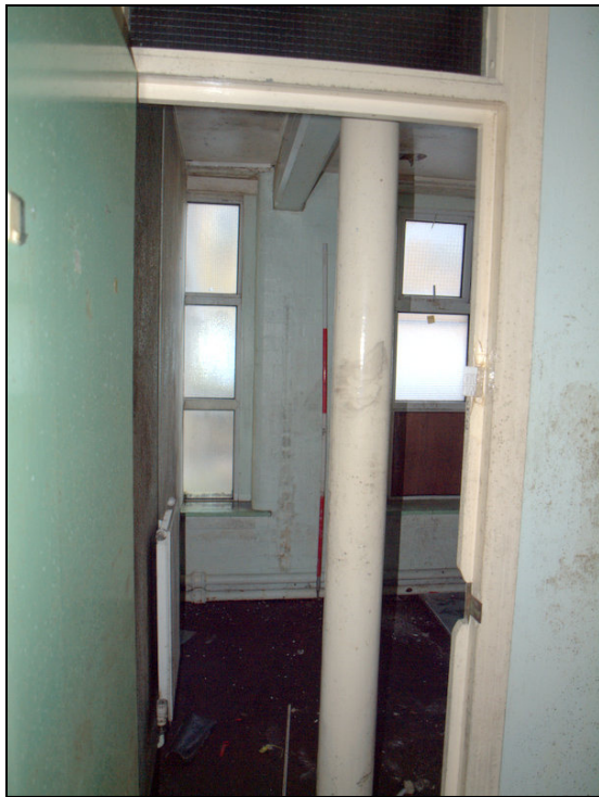
Plate 21: Entrance to room showing partition cutting window and stanchion in doorway
