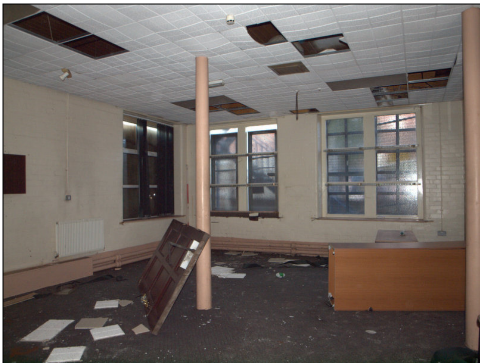
Plate 16: Southern room in ground floor of west block
