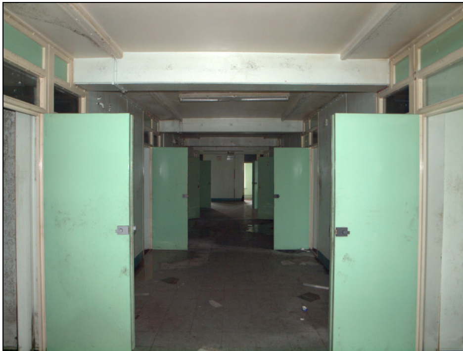
Plate 19: First floor central corridor.
