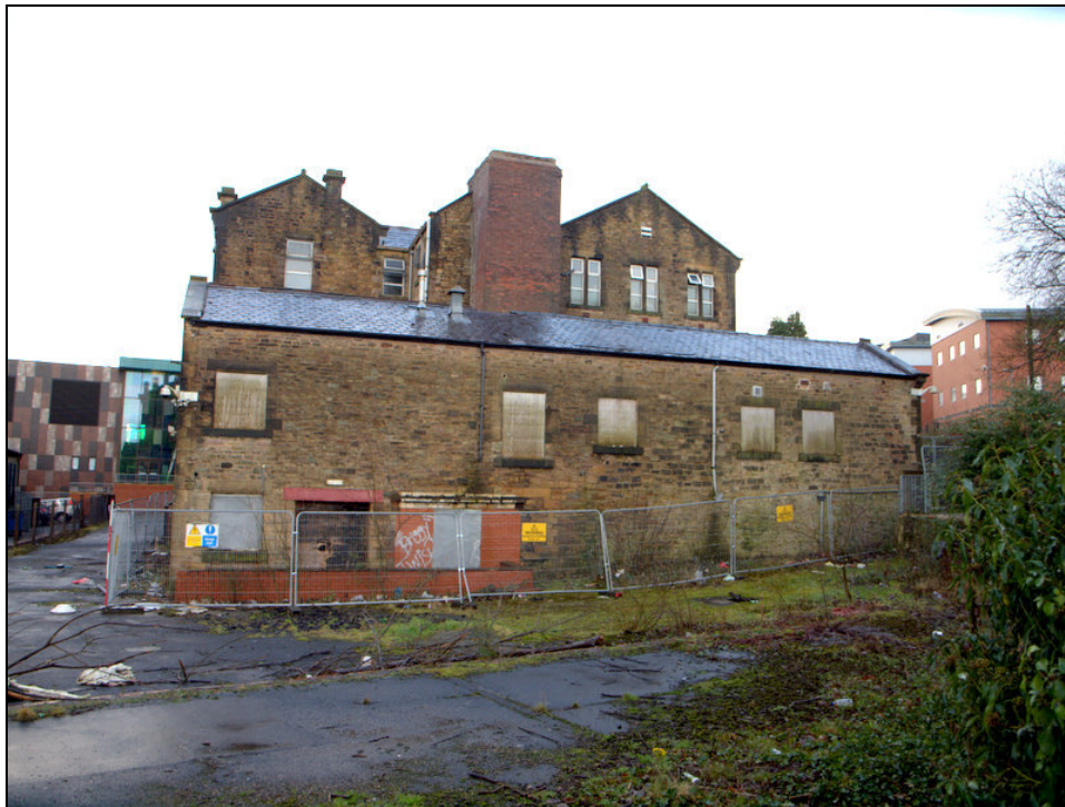
Plate 15: North elevation of the north block
