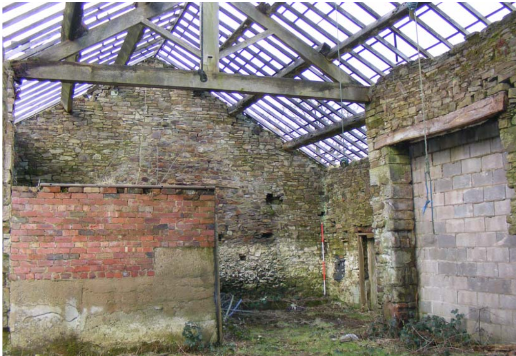
Plate 8. Barn – Internal looking west
