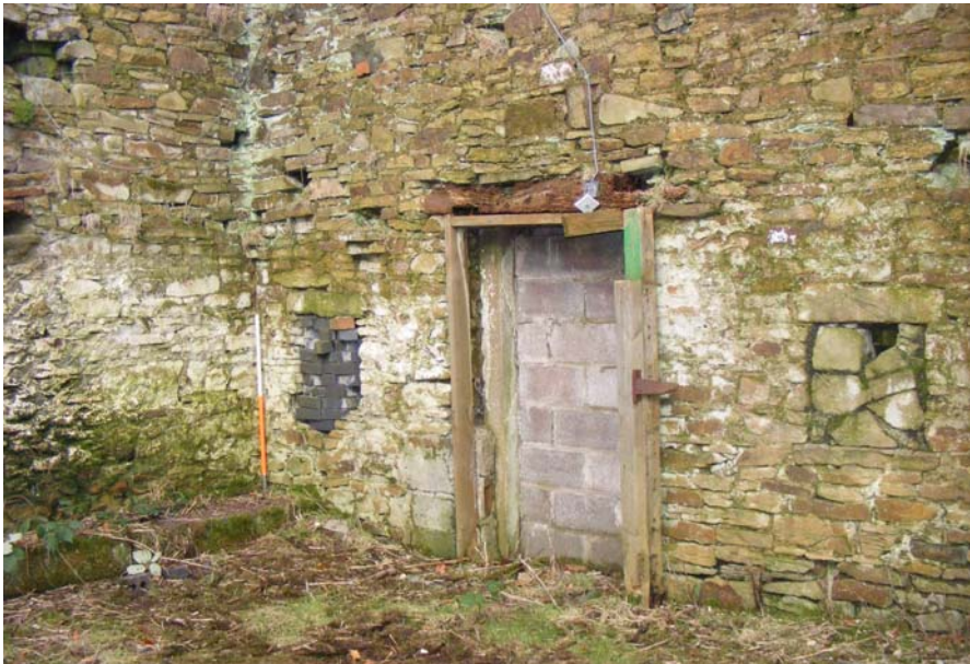
Plate 10. Barn – Internal barn projection looking north-west
