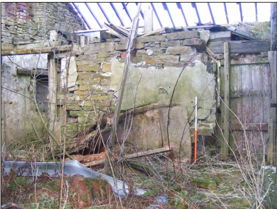
Plate 12. West extension – Internal looking north
