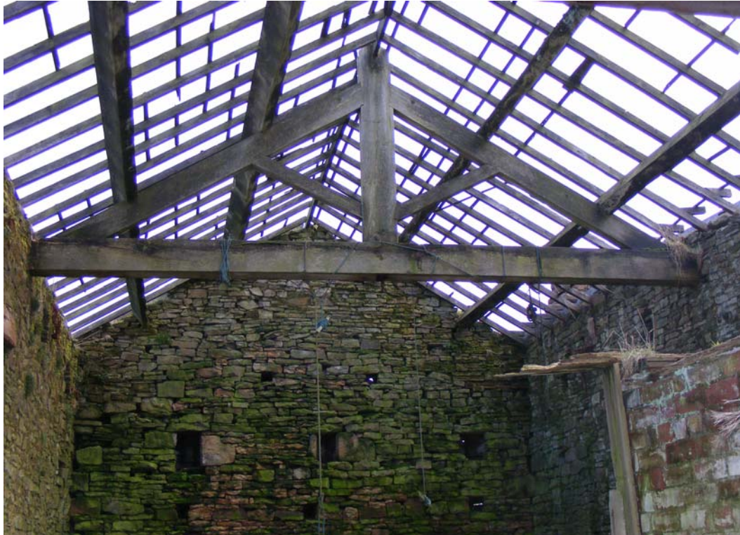
Plate 7. Barn – Internal king post roof truss
