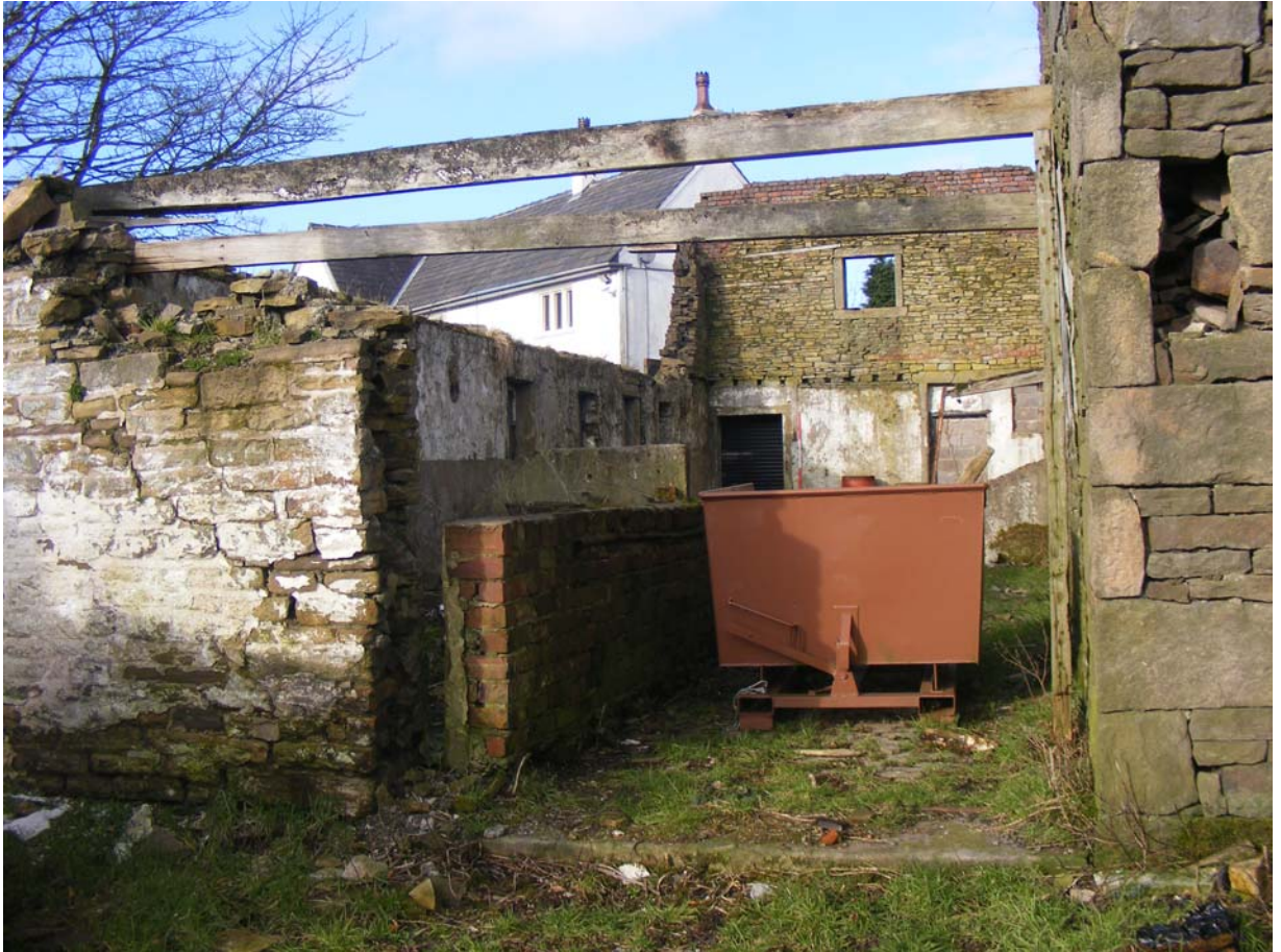
Plate 19. East outshot -internal -with south shippon beyond - looking west
