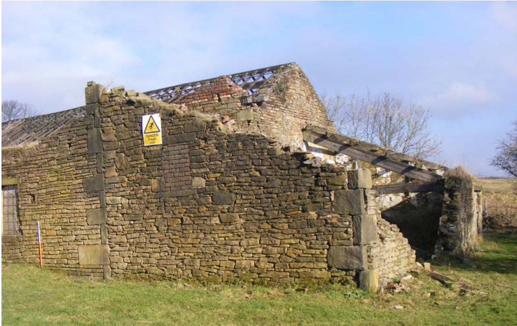
Plate 17. East outshot – looking north-west
