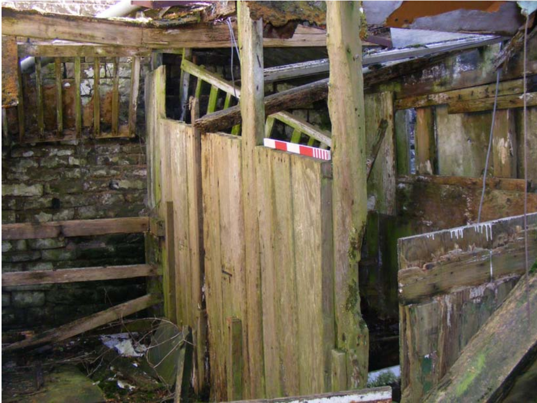
Plate 13. Stables against east wall of west extension
