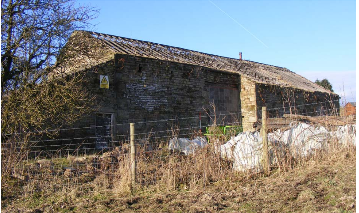
Plate 1. Barn – full view north elevation
