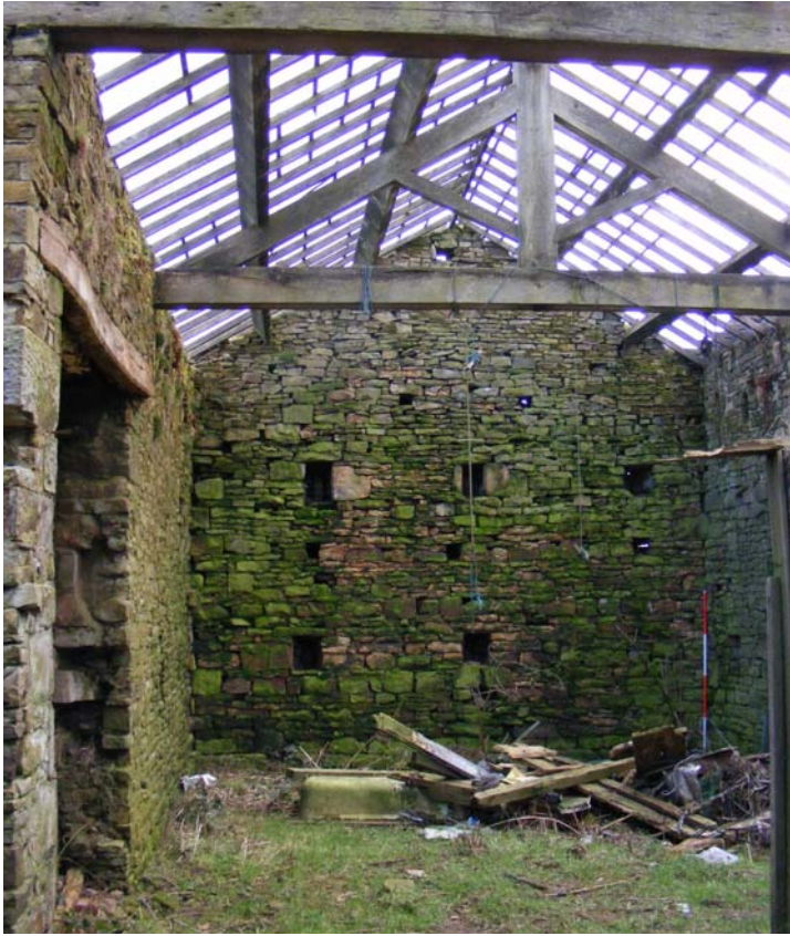
Plate 9. Barn – Internal looking west
