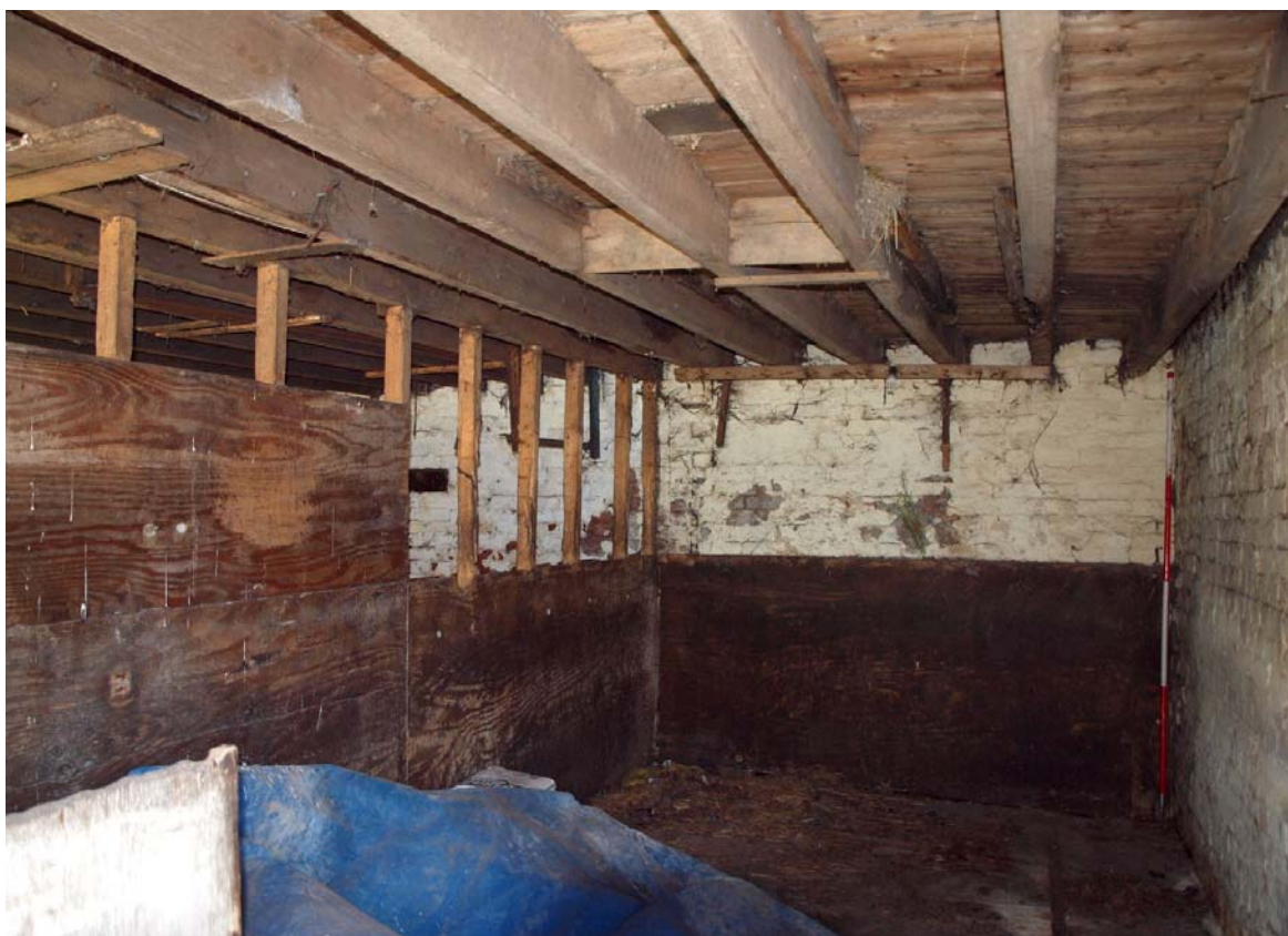
Plate 24: Interior of ground floor of stable, west loose box looking south
