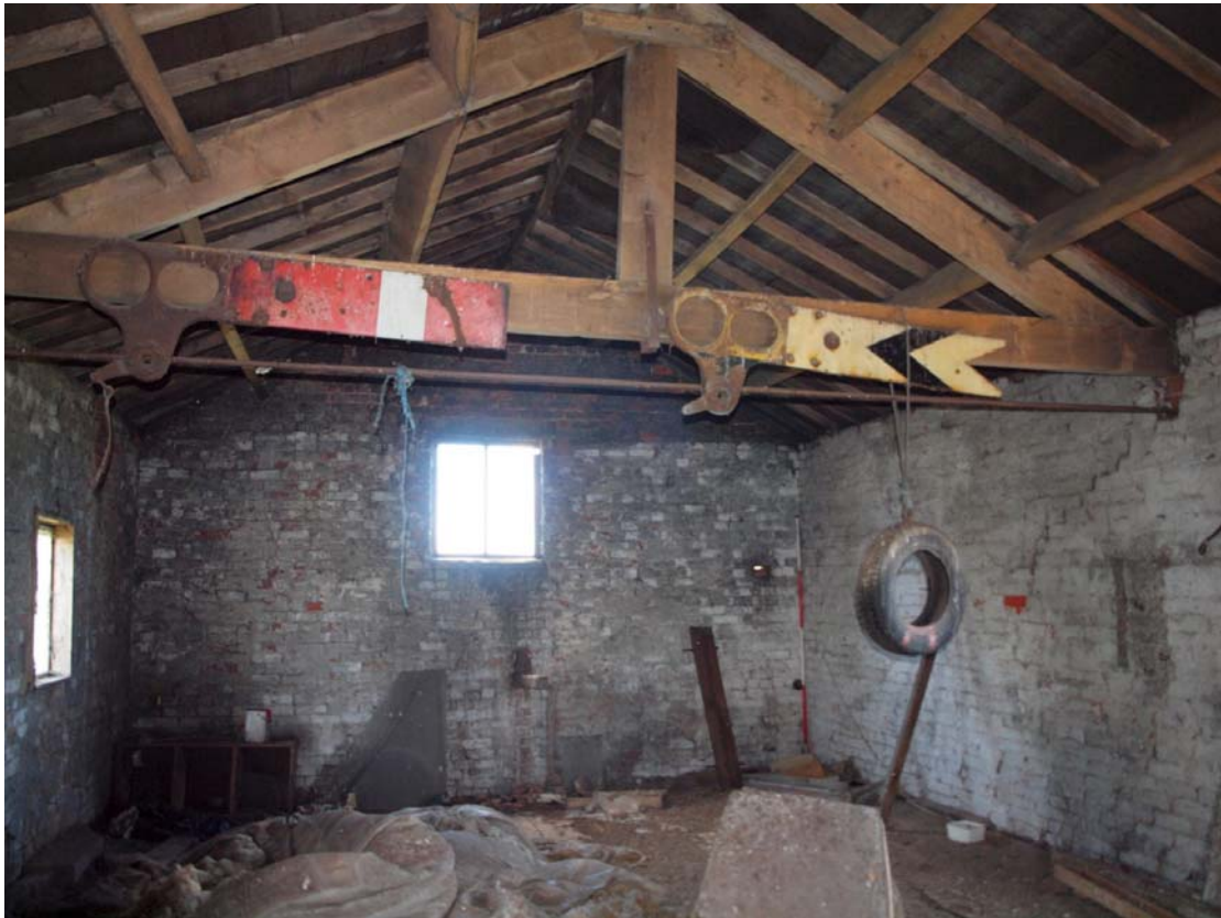
Plate 27: Stable; first floor looking west
