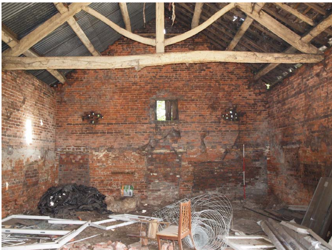
Plate 12: North wall of barn showing blocked doorways
