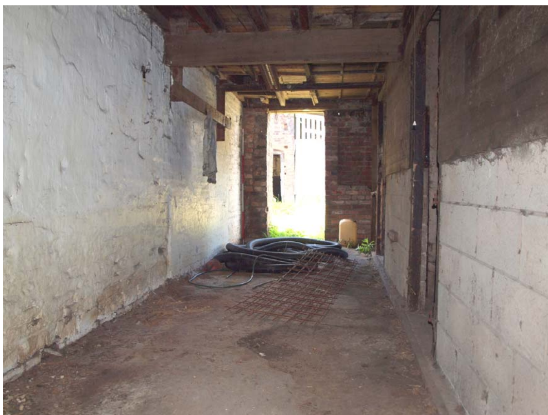
Plate 14: Doorway inserted in cattle door at south end of shippon.
