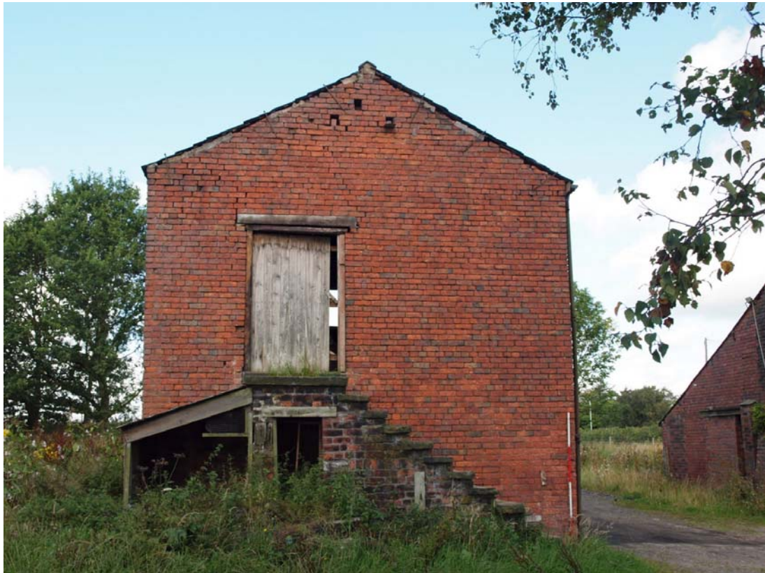
Plate 19: Eastern elevation of stable
