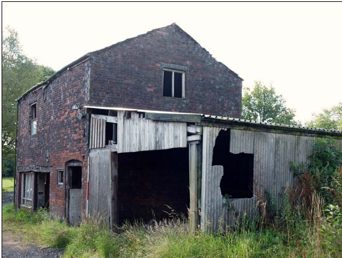
Plate 21: Western elevation of stable
