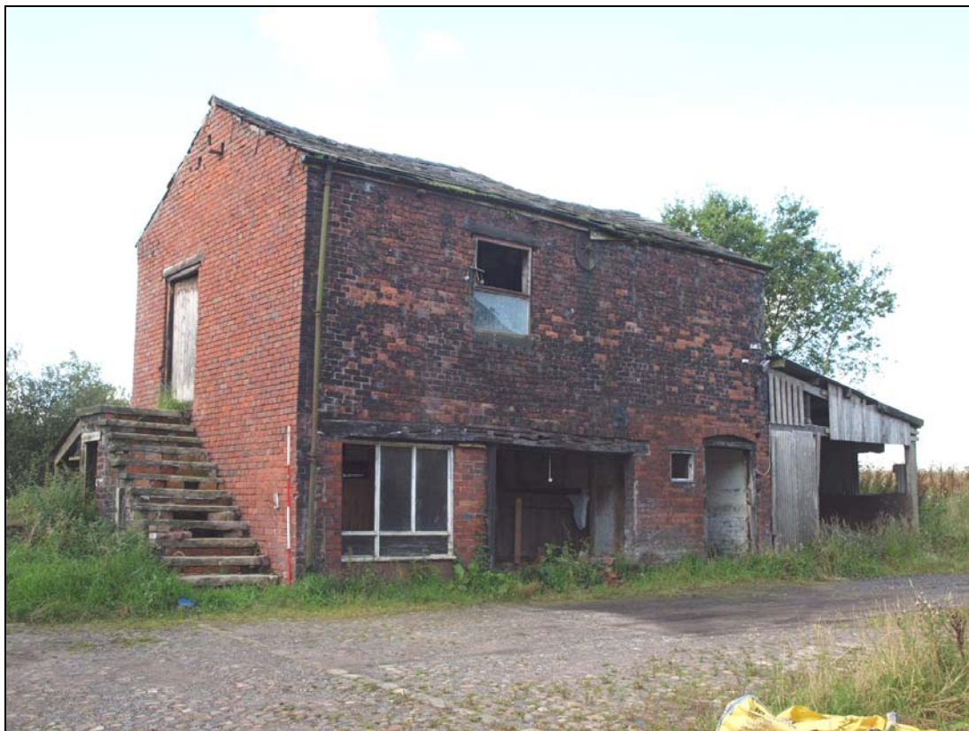
Plate 18: Northern elevation of stable
