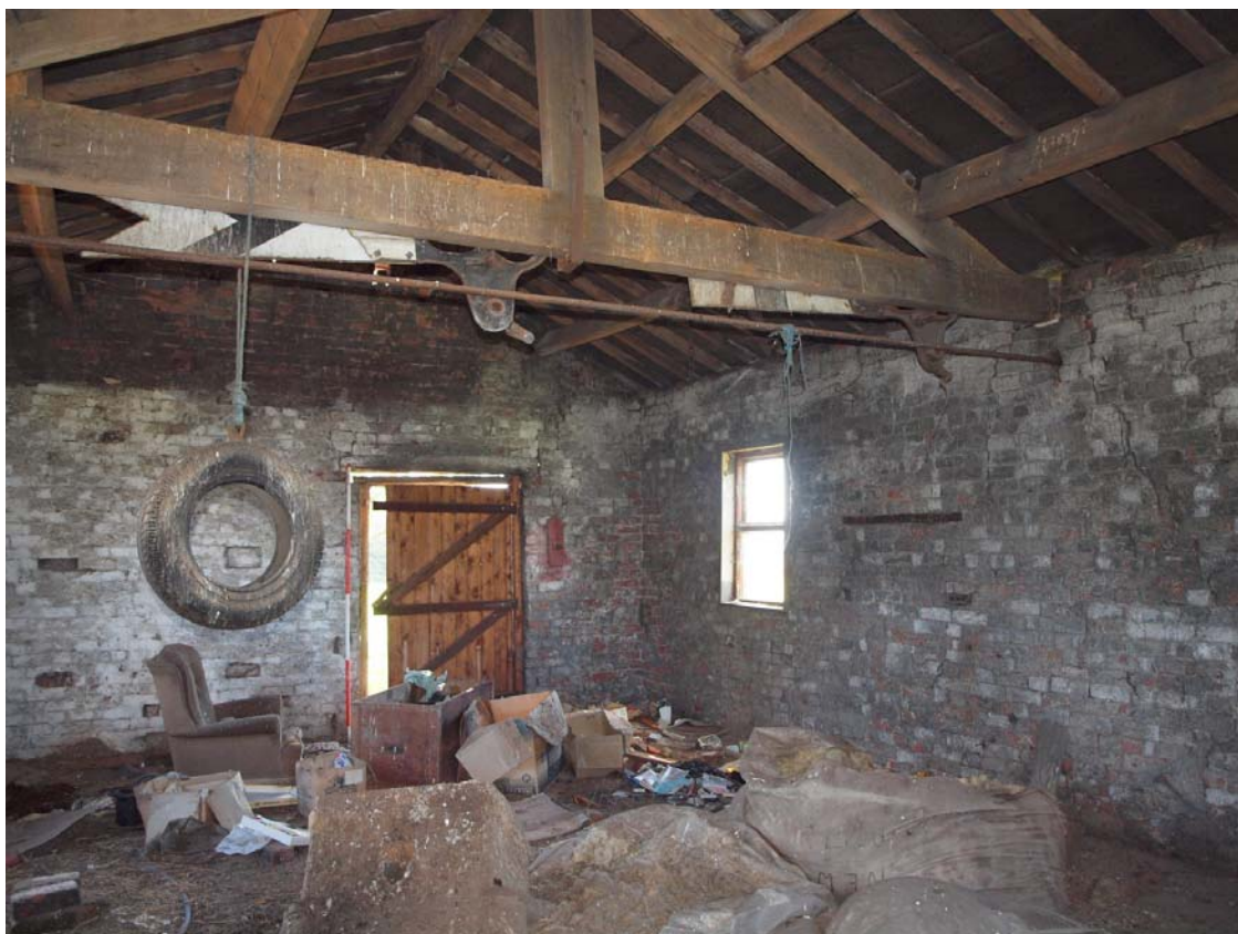
Plate 26: Stable; first floor looking east
