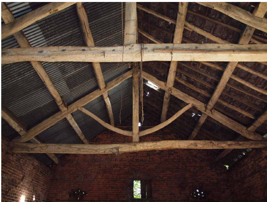
Plate 13: Hand cut timber truss in barn
