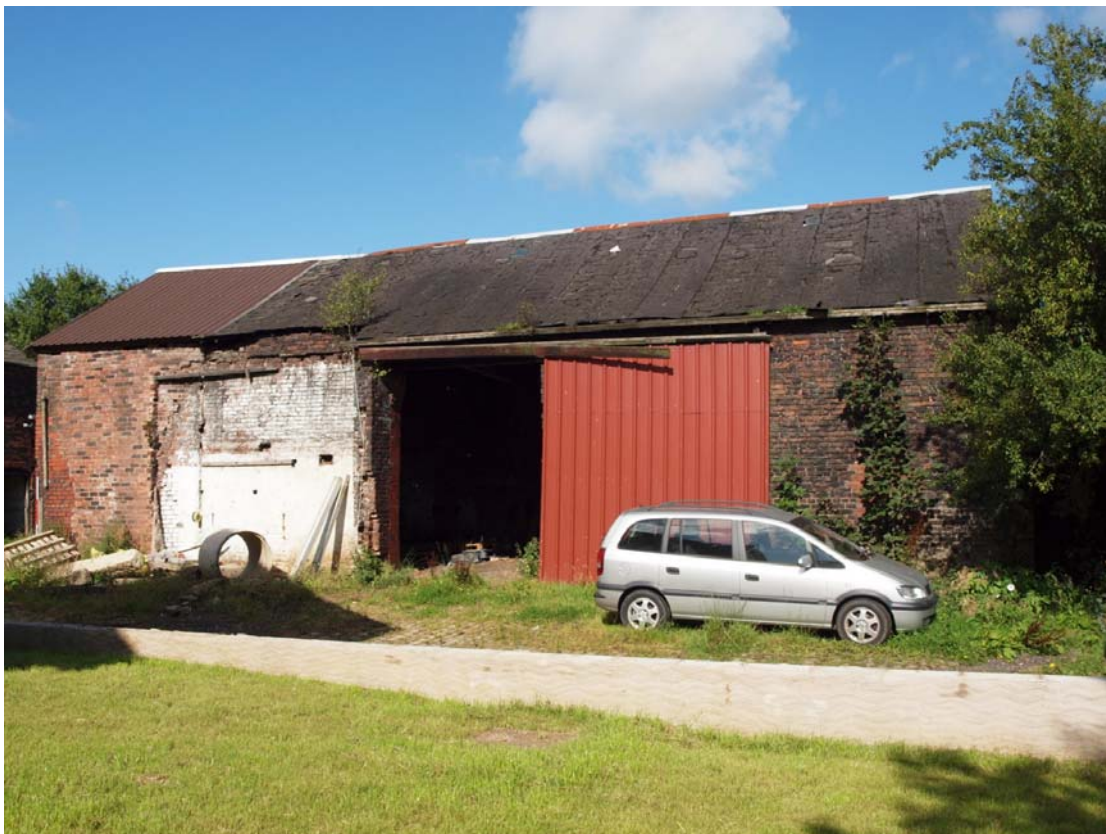
Plate 2: Eastern elevation (front) of barn
