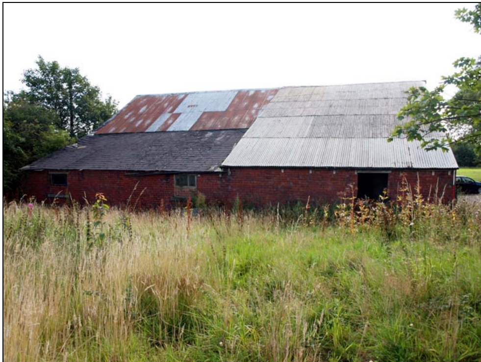
Plate 4: Western elevation of barn
