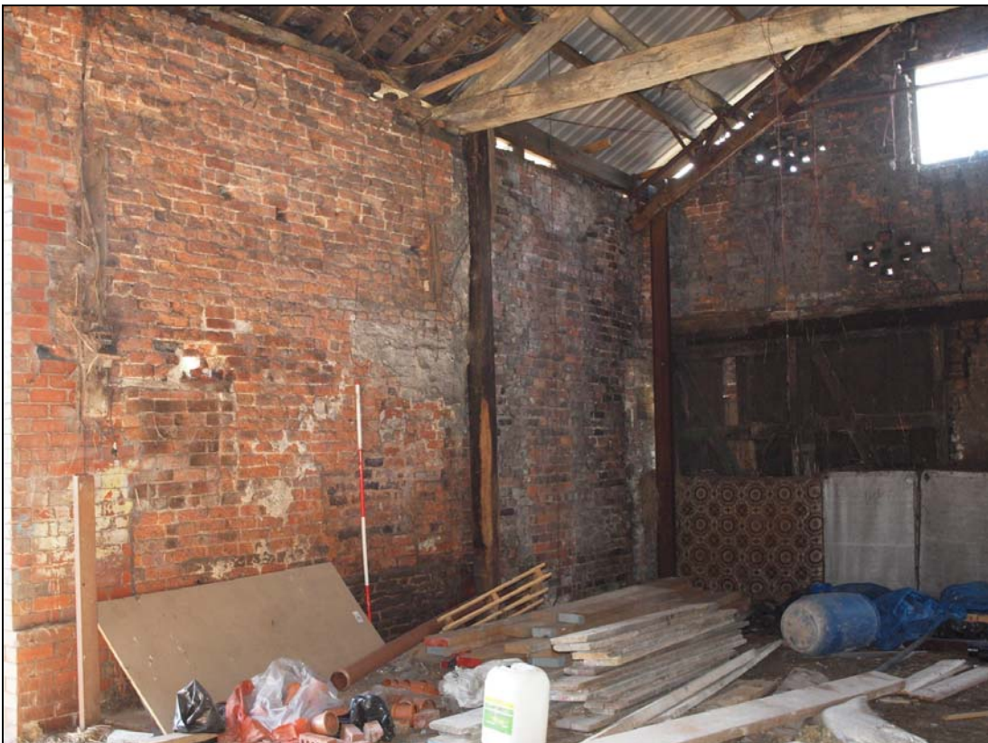
Plate 10: Southern end of east wall of barn showing timber posts.
