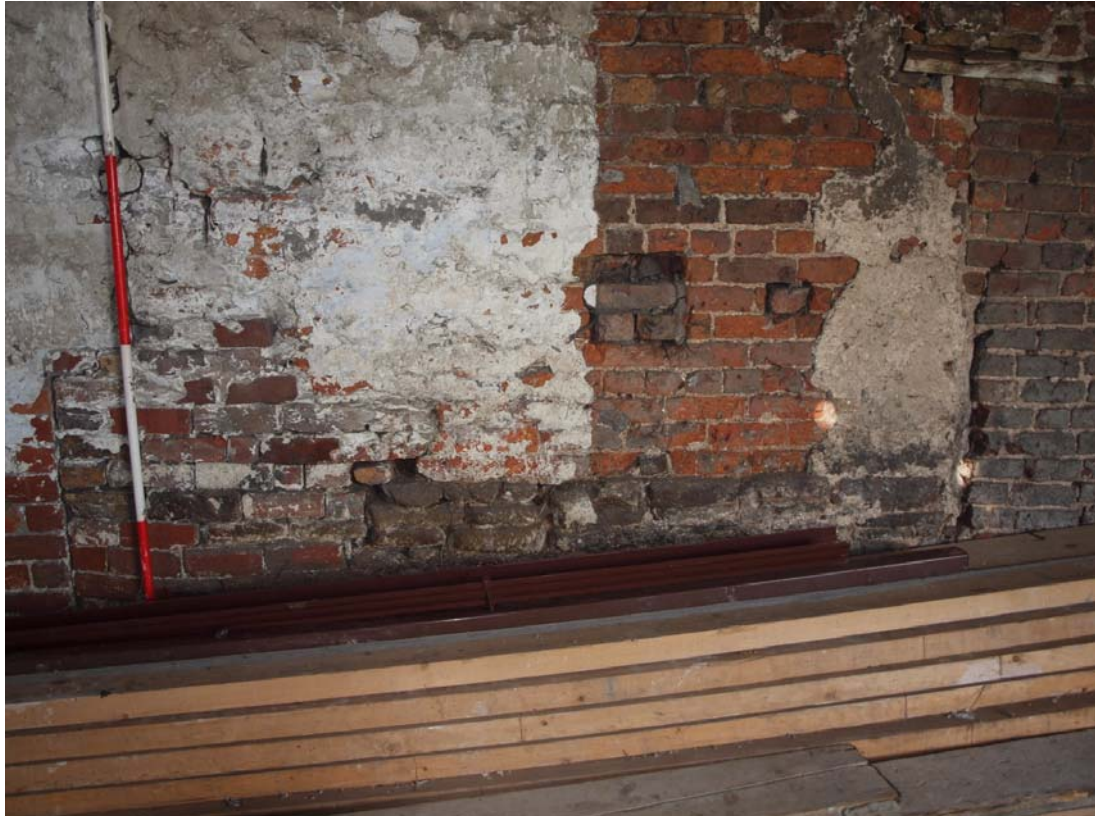
Plate 8: Area of sandstone walling in west wall of barn
