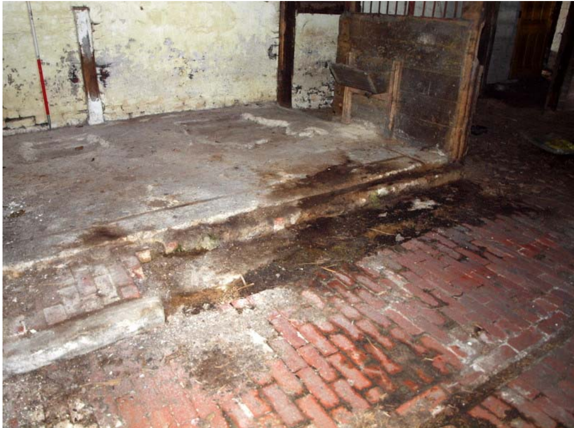
Plate 17: Brick and concrete flooring.
