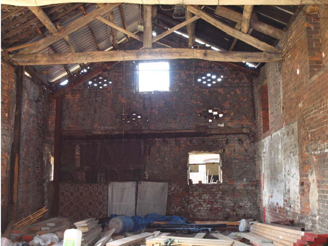
Plate 9: Southern wall of the barn showing window inserted into doorway
