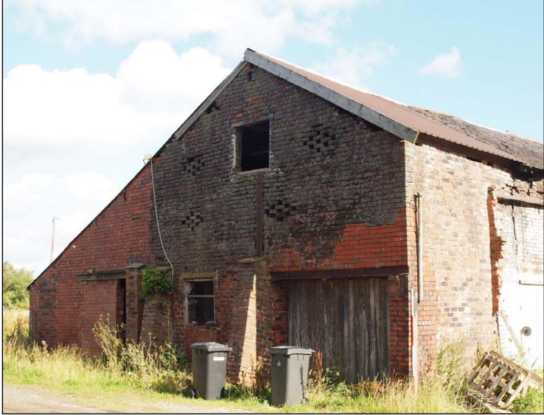
Plate 3: Southern elevation of barn
