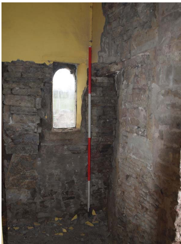
Plate 50: Arched window and recess at junction of east and south walls of west wing
