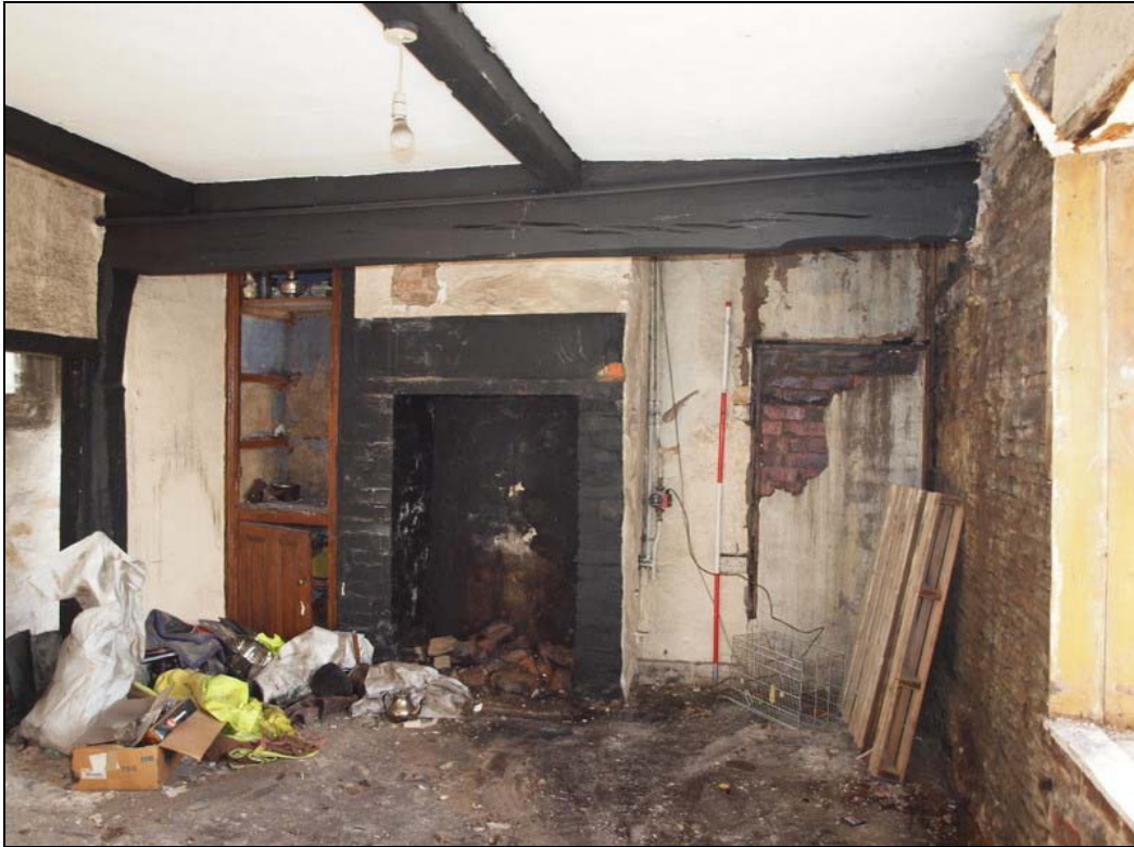
Plate 27: Inglenook fireplace in east wall of west bay of central dwelling. Heck separating house room from mell passage is to left of fireplace
