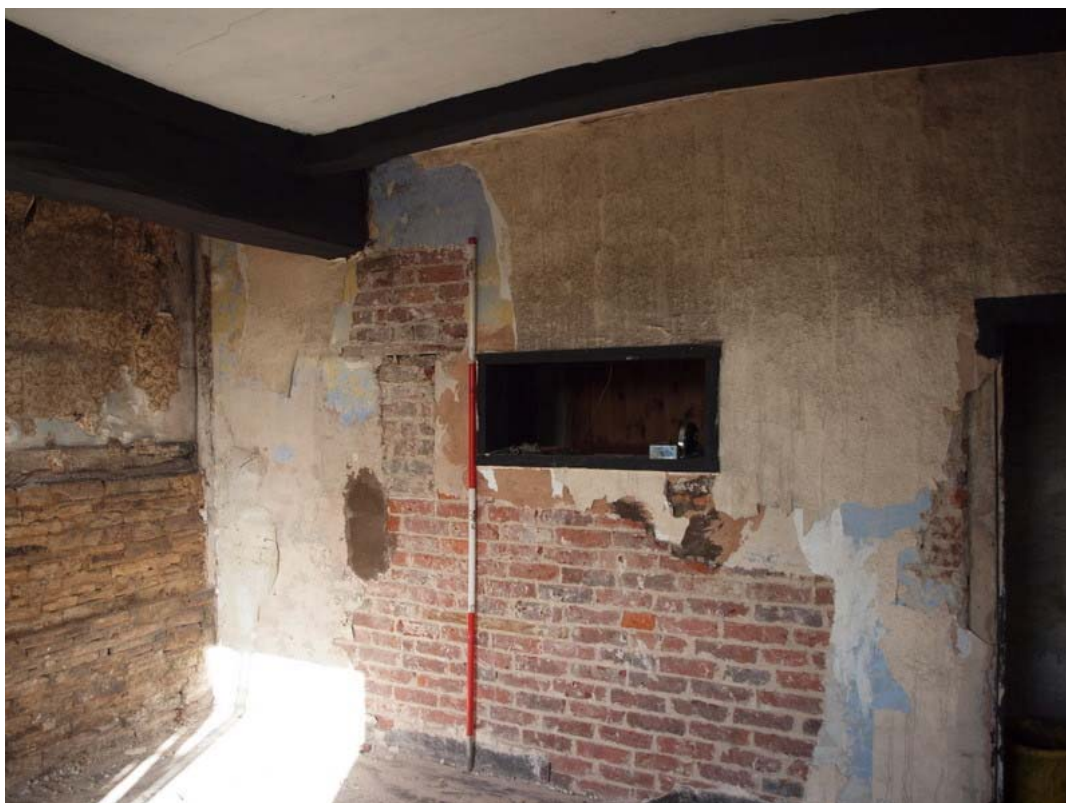
Plate 29: Modern partition extending to south of mell passage beyond
