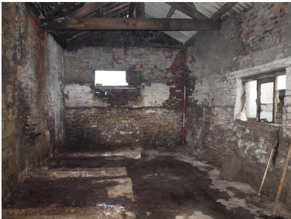
Plate 53: Interior of western extension showing remains of concrete boskins
