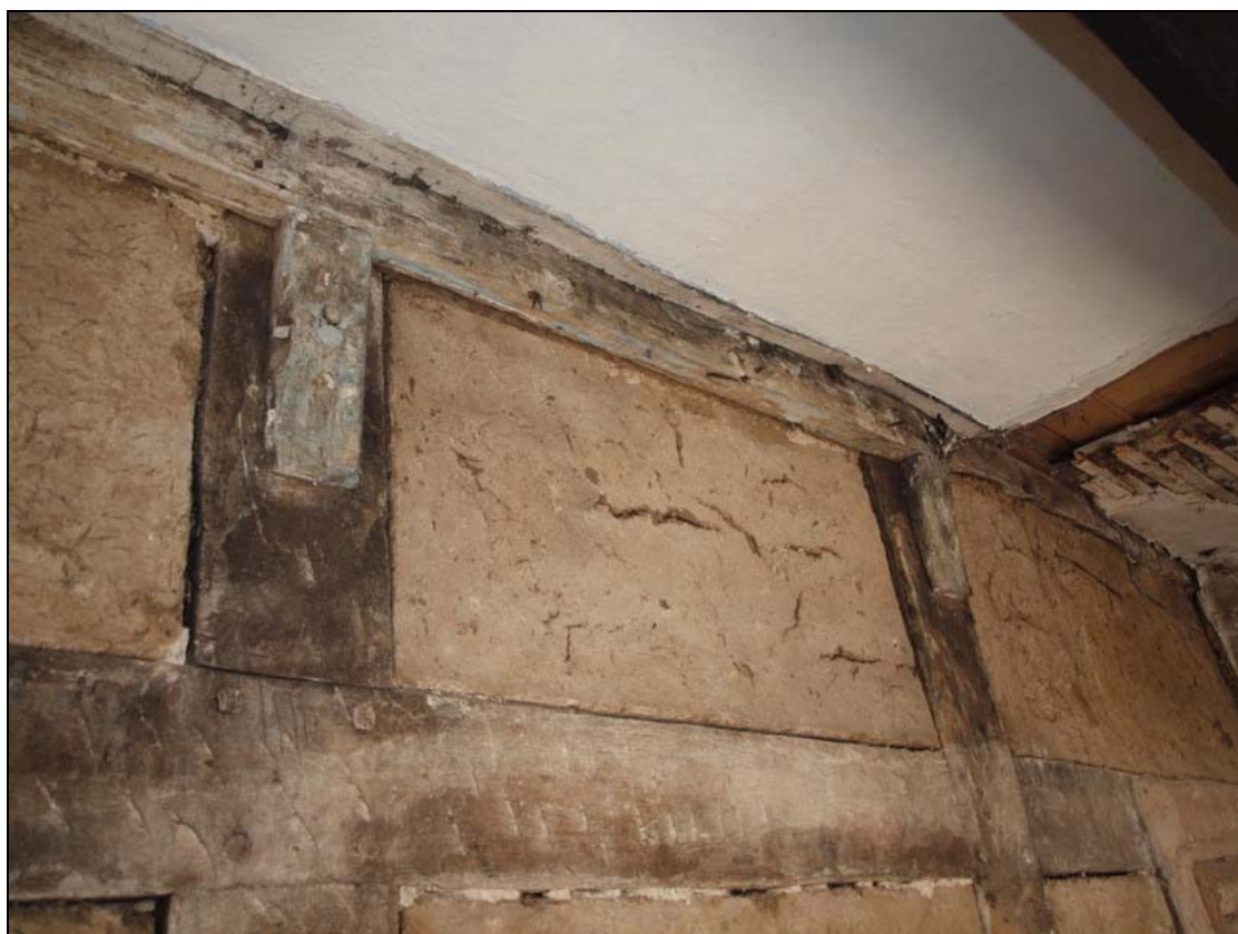
Plate 33: Detail of timber frame showing timber brackets, pegs, carpenter's marks and adze marks
