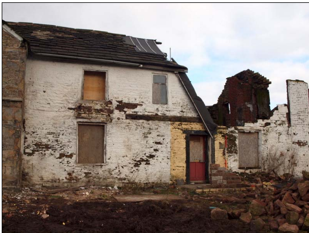
Plate 9: South elevation of the dwelling
