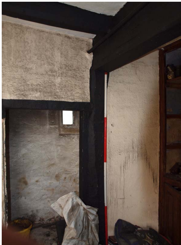
Plate 28: Heck post supporting bressummer with mell passage beyond
