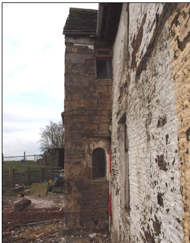
Plate 14: South end of east elevation of west wing.
