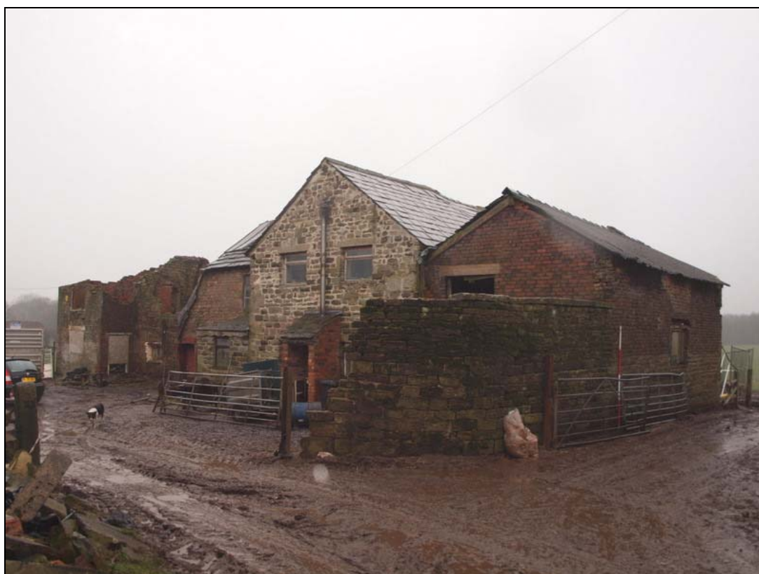
Plate 2: Buildings to be redeveloped looking south-east
