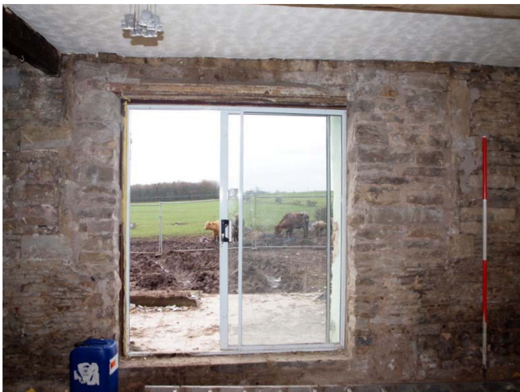
Plate 47: Mullioned window pierced by French window in south wall of wing
