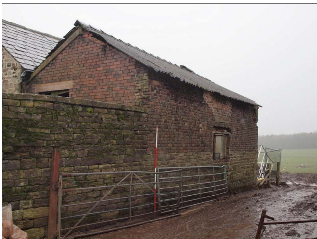
Plate 18: West elevation of western extension
