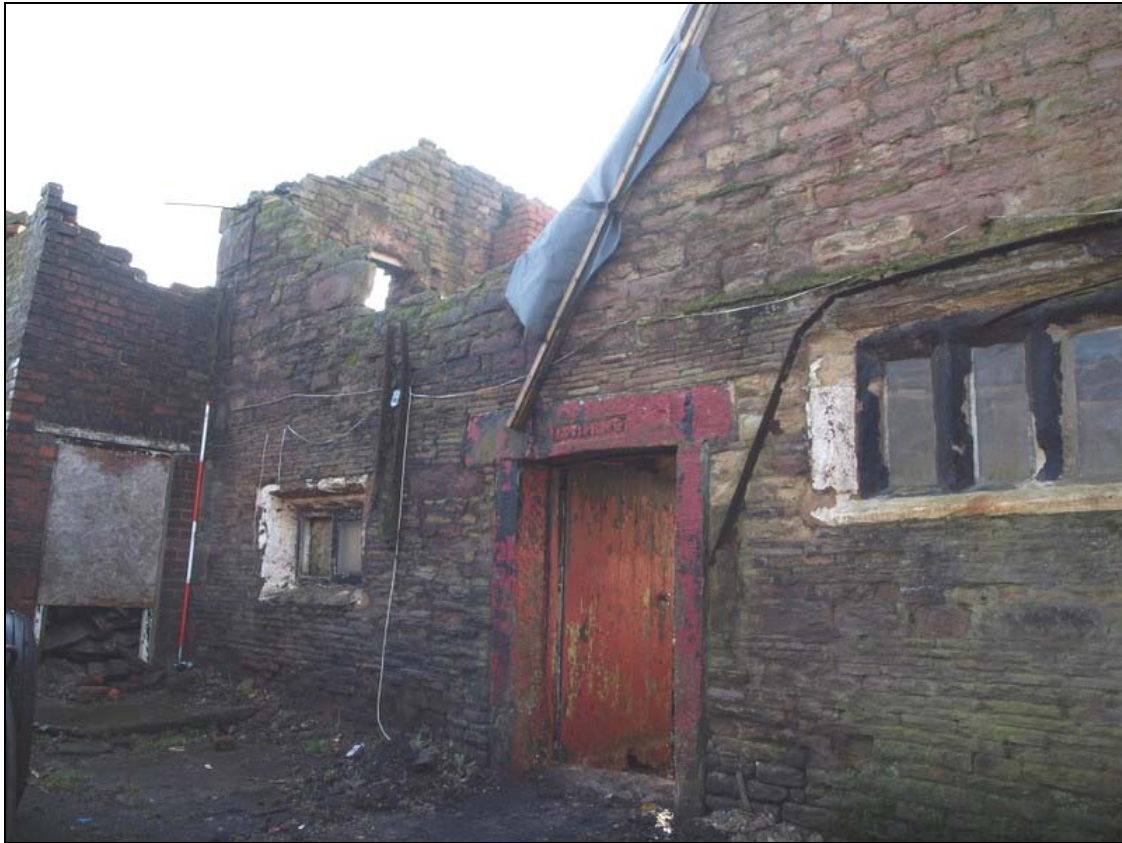
Plate 5: Mullioned window with chamfered frame to east (left) of doorway
