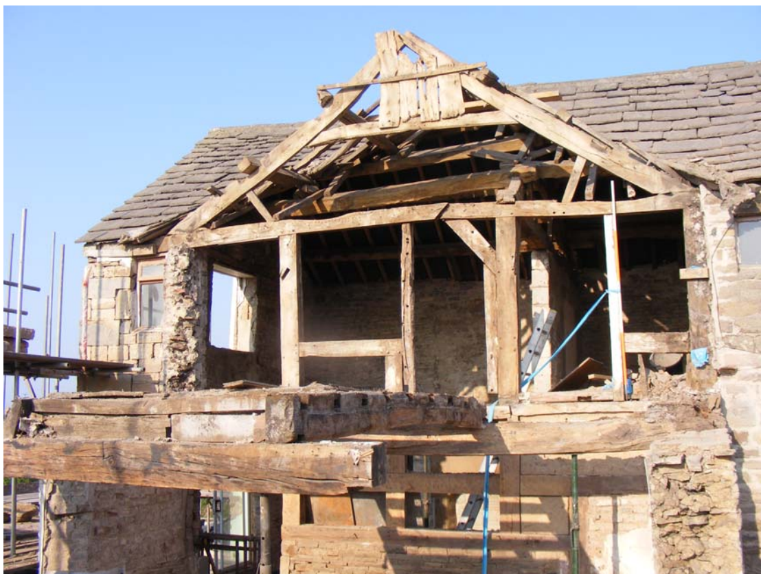
Plate 38: Exposed timber frame at ground and first floor levels
