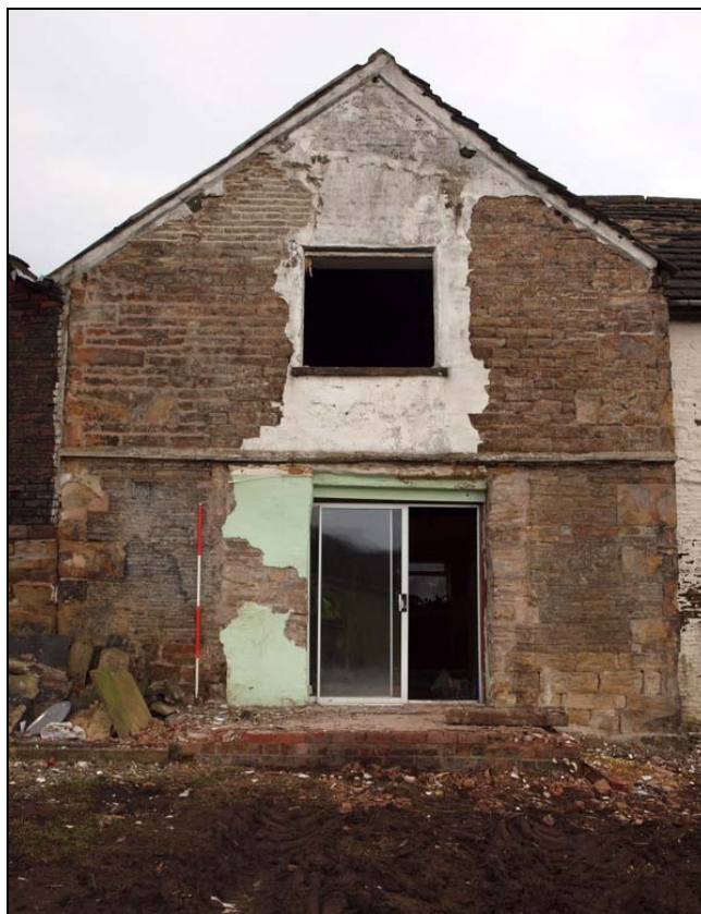
Plate 13: South elevation of west wing
