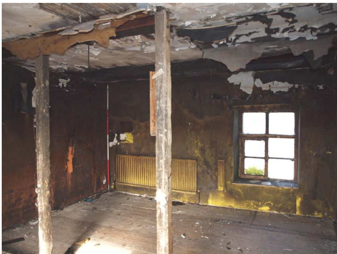
Plate 36: First floor of west bay of central dwelling looking north-west
