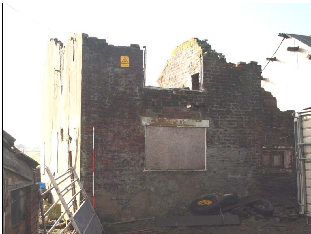
Plate 20: North elevation of eastern extension
