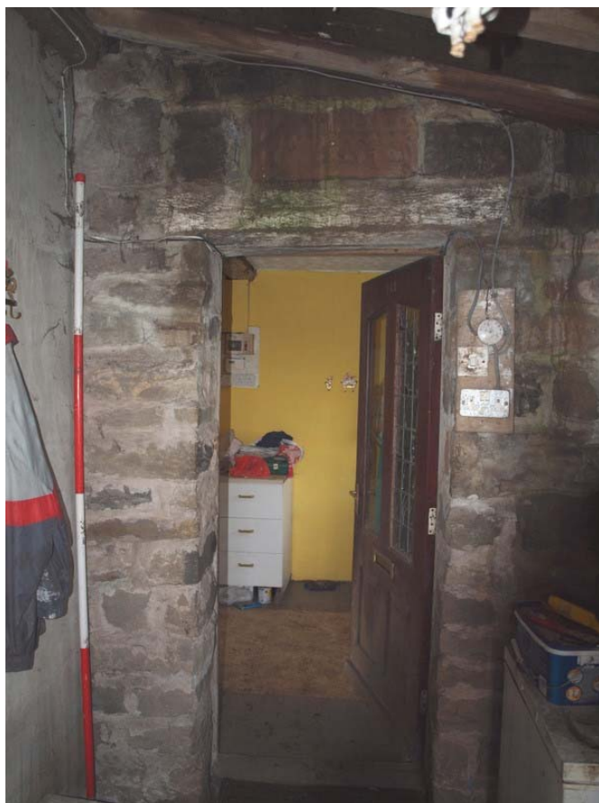
Plate 15: North end of east elevation of west wing showing doorway
