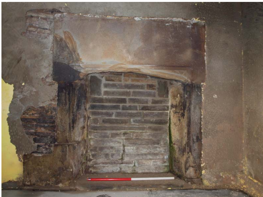
Plate 45: Detail of fireplace in south bay of west wing
