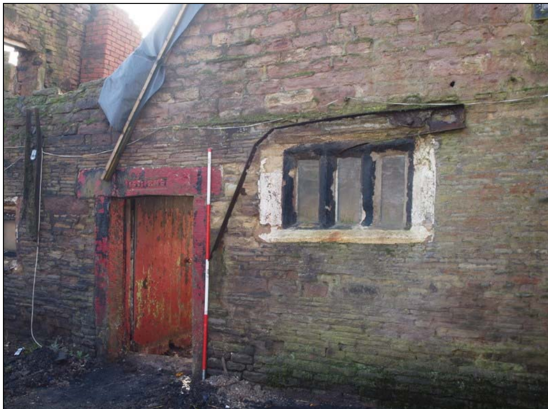
Plate 6: Window with chamfered frame and splayed mullions to west (right) of doorway
