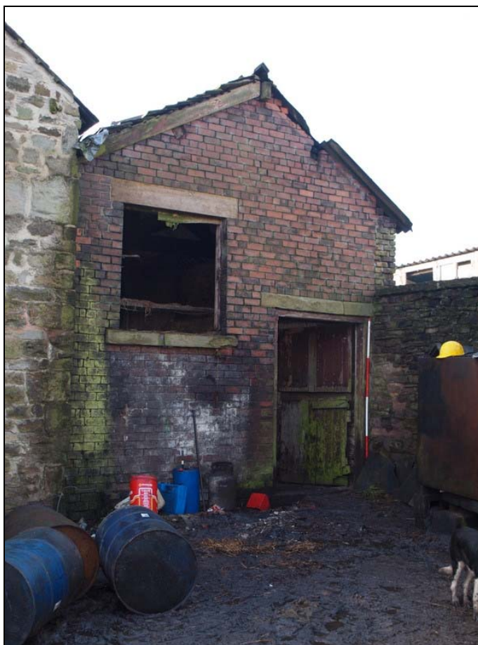
Plate 17: North elevation of western extension
