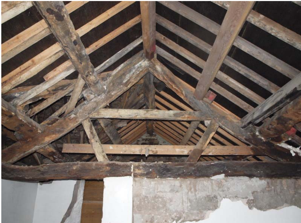
Plate 52: Exposed hand cut timber truss in west wing
