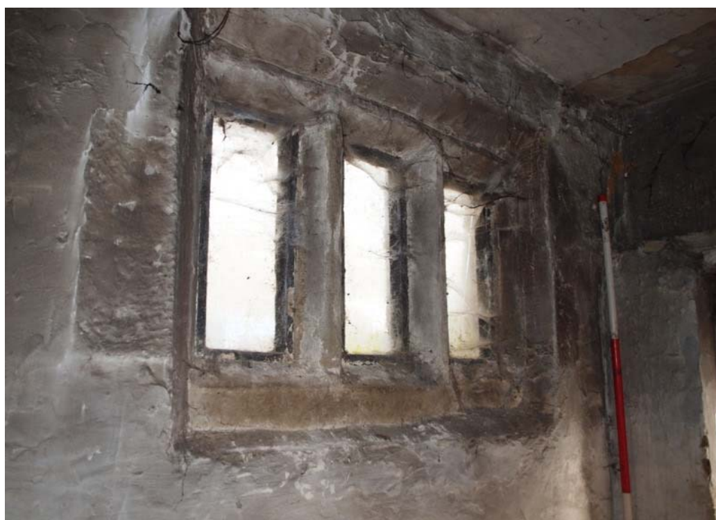
Plate 26: Mullion window in north wall of mell passage
