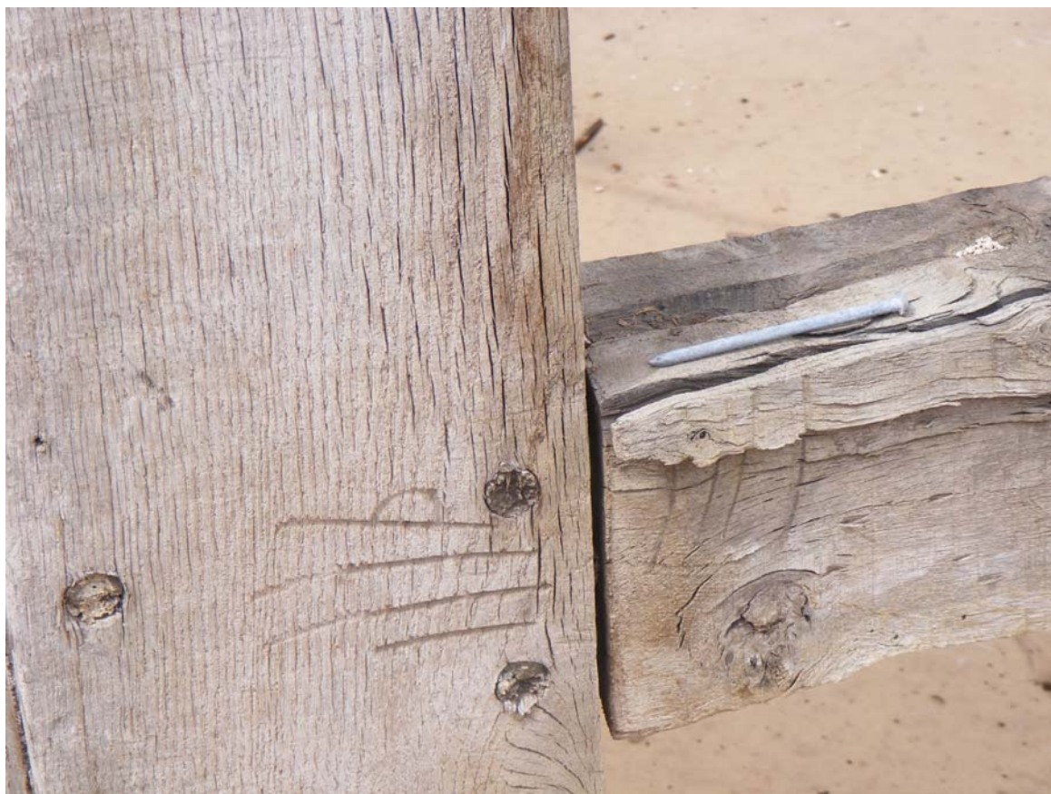
Plate 39: Carpenter's mark at first floor level matching those on ground floor (cf Plate 34)
