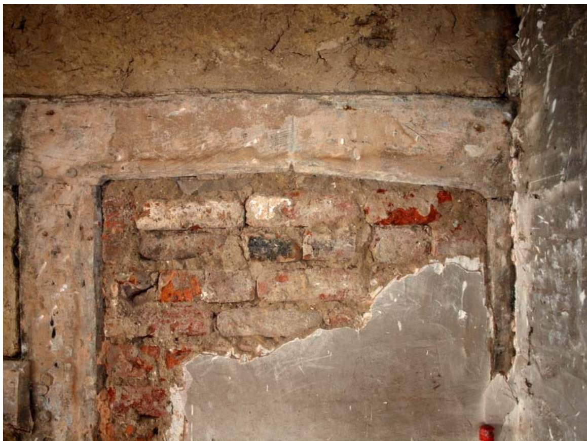
Plate 35: Detail of lintel of north doorway in timber-framed wall
