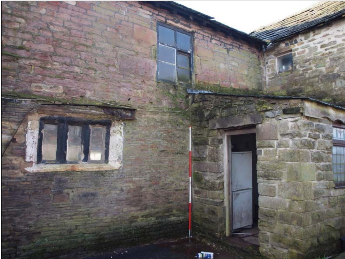
Plate 7: Variation in stonework above and below west window lintel
