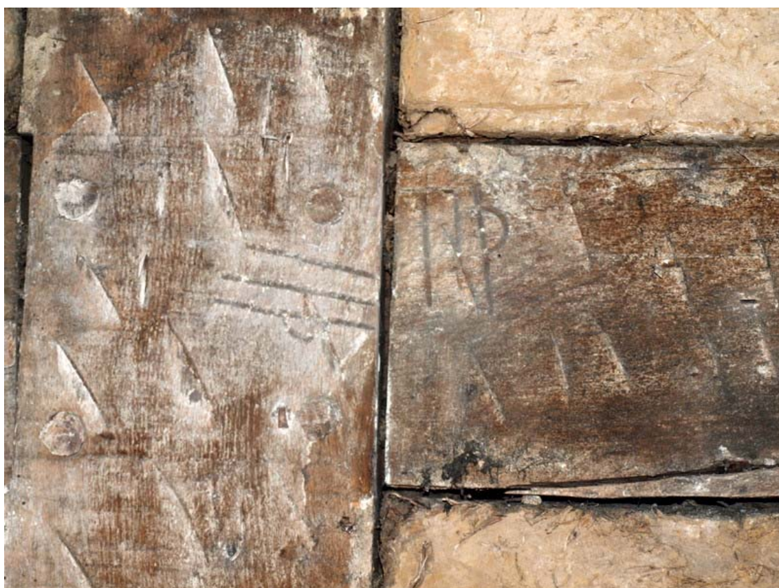
Plate 34: Detail of carpenter's marks on timber frame
