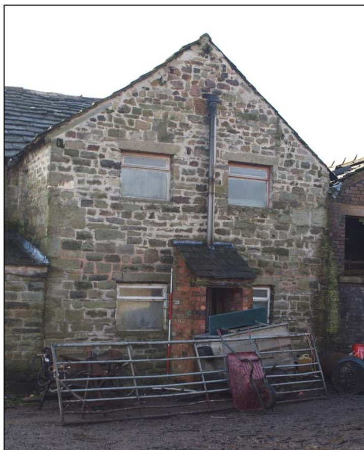
Plate 10: North elevation of west wing
