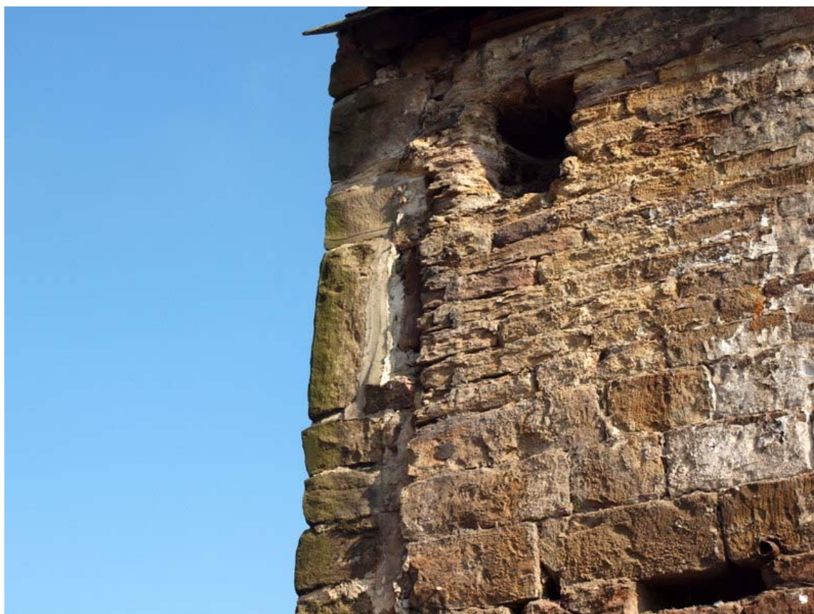
Plate 12: Remains of timber framing in north end of west wall of west wing
