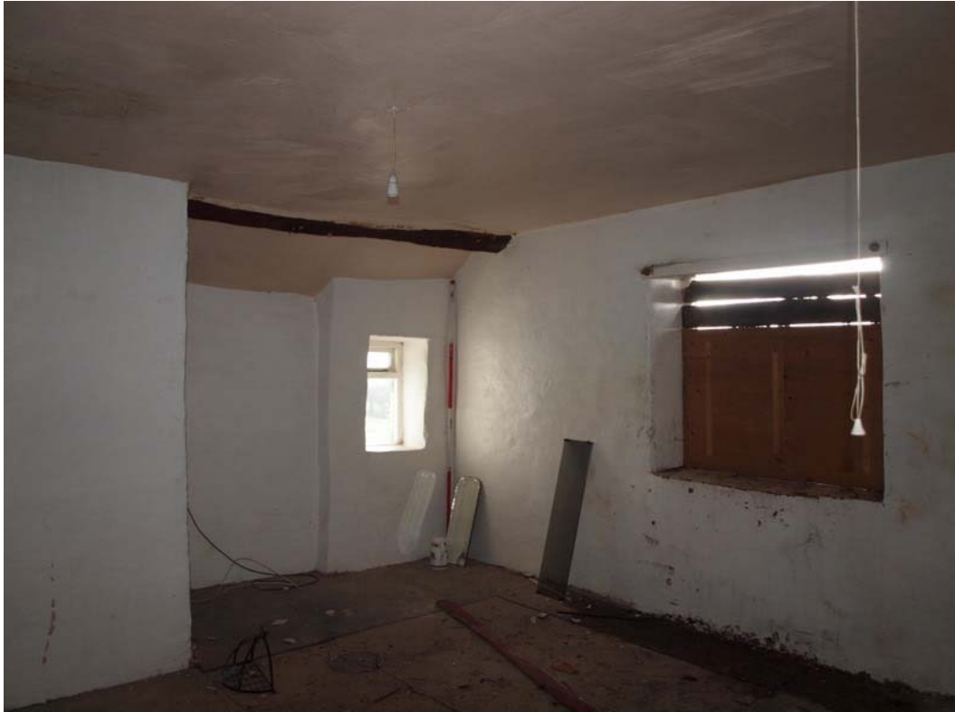
Plate 51: First floor of west wing; south end looking west
