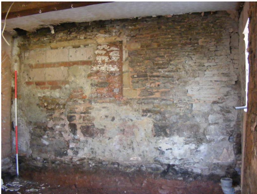
Plate 43: Frame of mullion window in west wall of west cell in north bay of west wing
