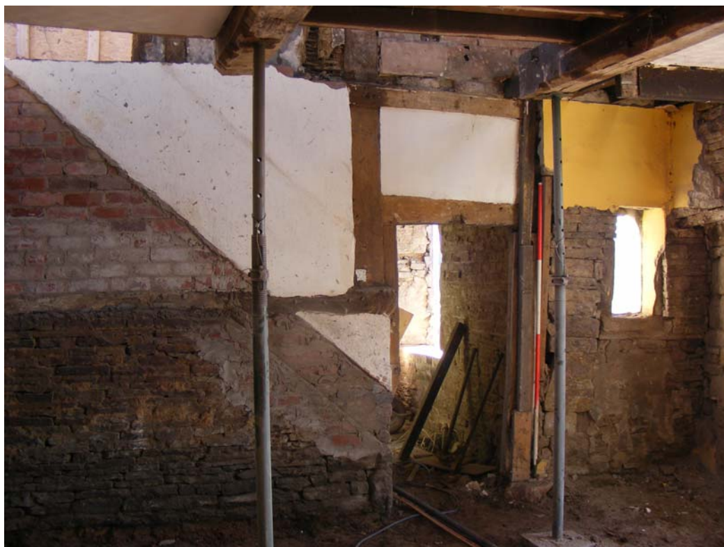
Plate 49: East wall of west wing with staircase removed
