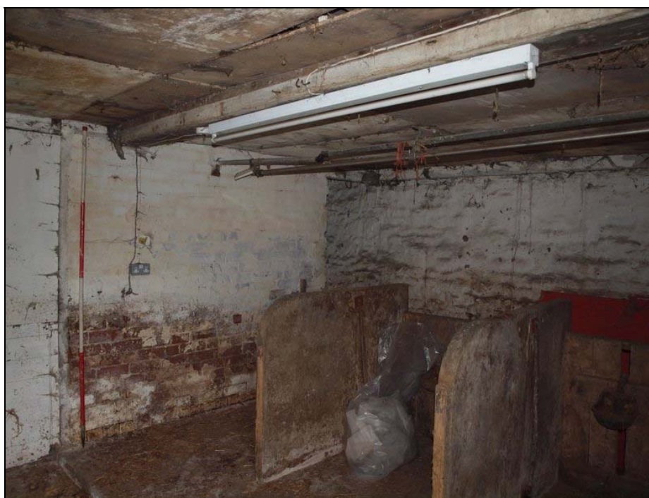
Plate 33: Interior of east side of lean-to shippon showing concrete boskins
