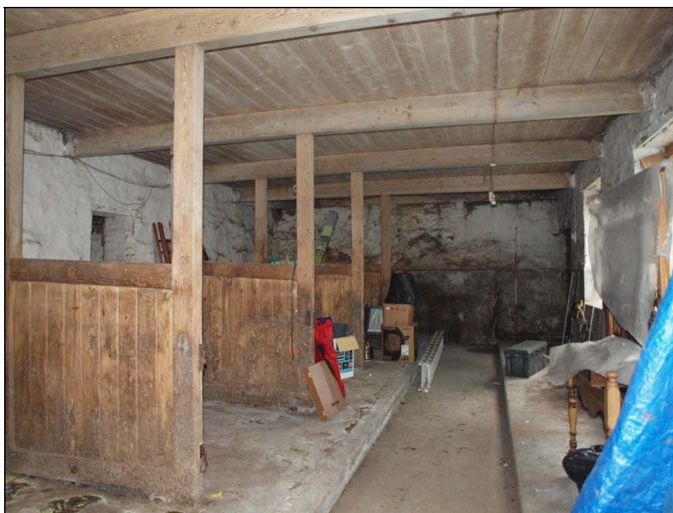
Plate 11: Interior of barn looking west
