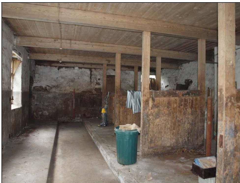
Plate 12: Interior of barn looking east
