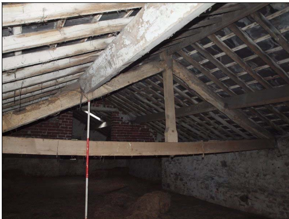
Plate 21: Detail of modern roof structure
