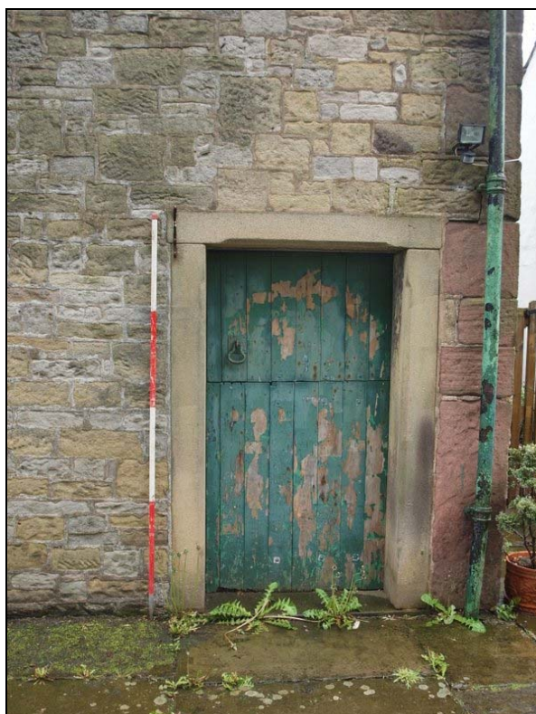
Plate 2: Detail of yellow sandstone snecked rubble stonework, red sandstone quoins and cattle doorway at west end of north elevation
