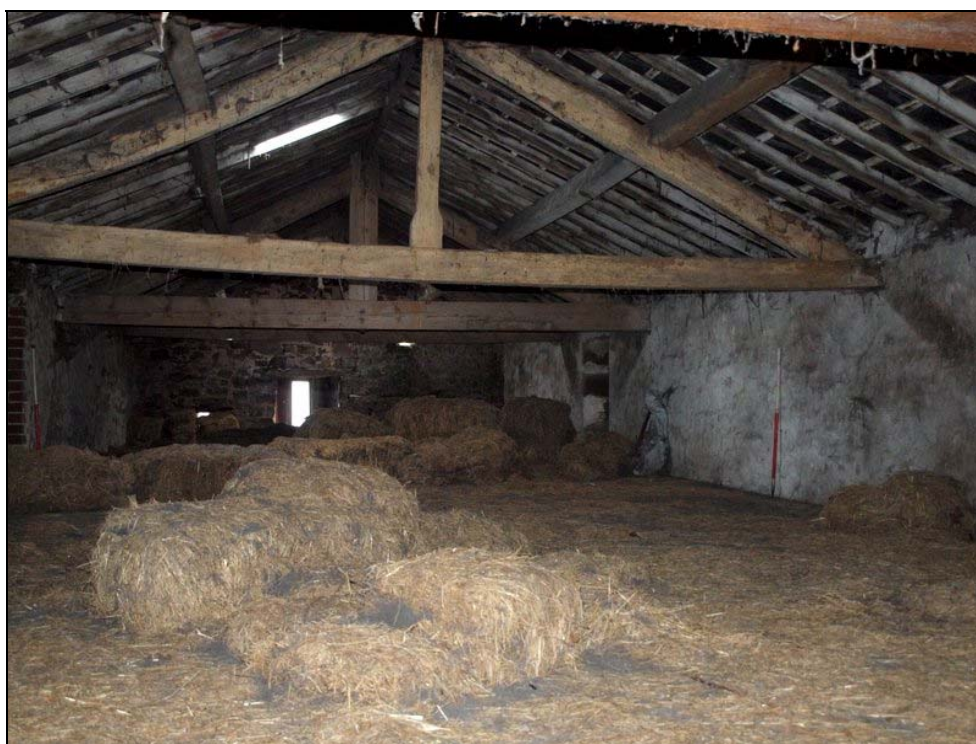
Plate 23: General shot of first floor
