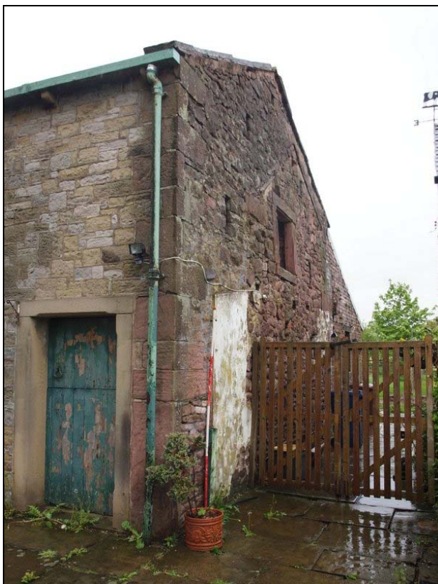
Plate 6: Detail of west gable
