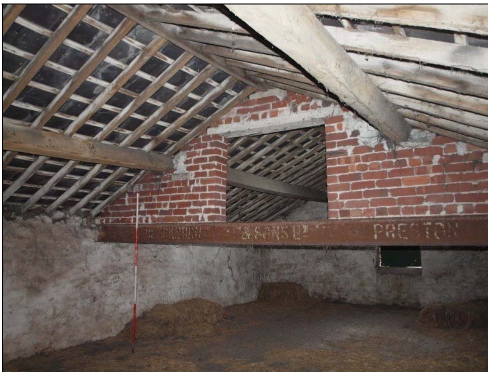
Plate 20: RSJ beam with brick over at east end
