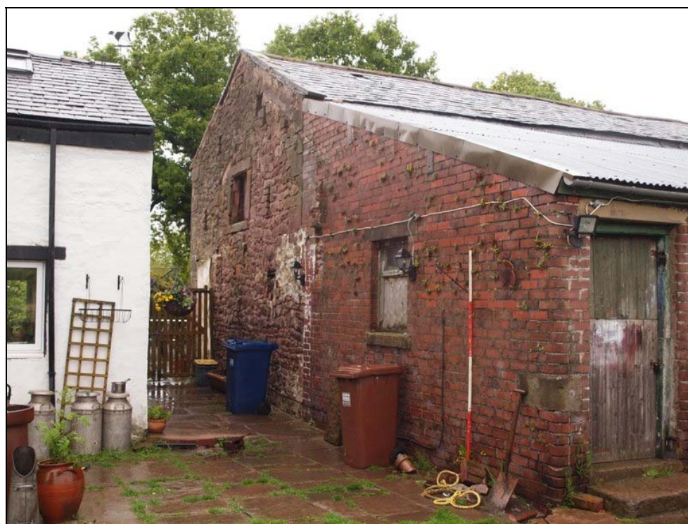
Plate 8: West gable and brick lean-to
