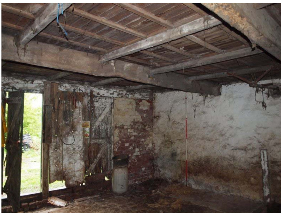
Plate 28: Interior of lean-to access area to shippon
