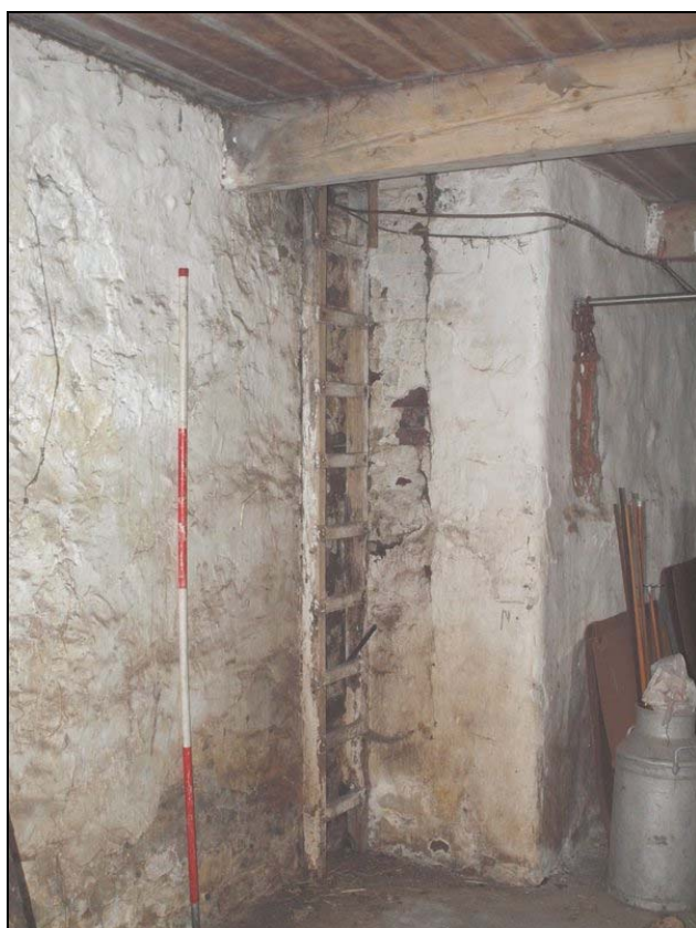
Plate 15: Jacob's ladder with brick infill between former barn and shippon behind
