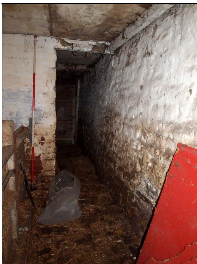
Plate 34: Feeding passage of lean-to shippon
