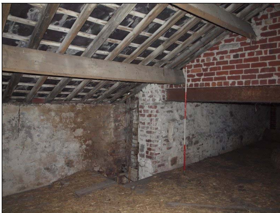
Plate 25: Brick infilling at first floor level on south wall at junction of former barn and shippon
