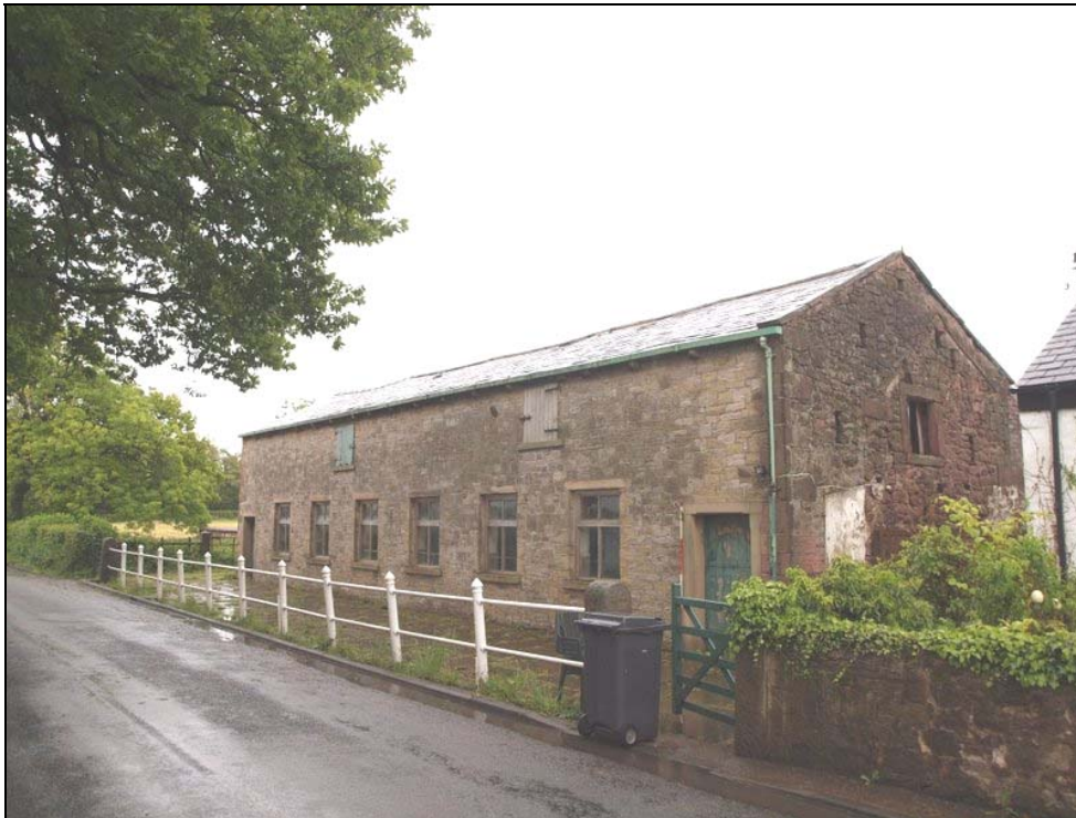
Plate 5: North elevation of yellow sandstone and western gable of red sandstone
