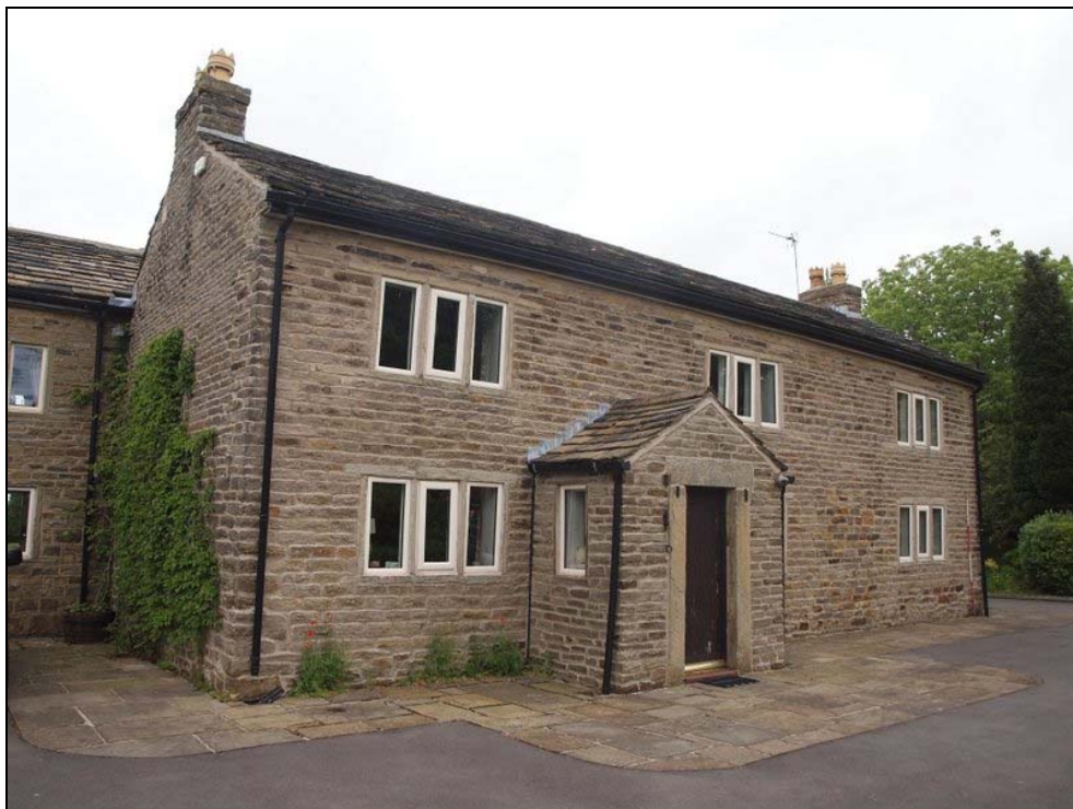
Plate 16/2: Front (south) side of the building, east end
