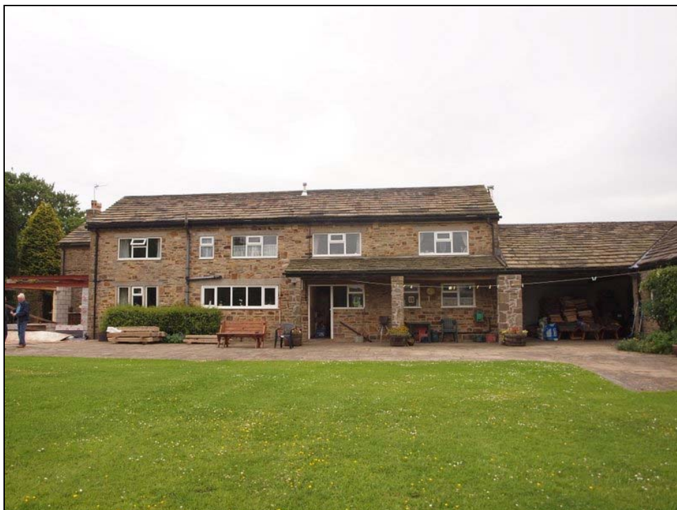
Plate 12/5: Rear (north) side of the building
