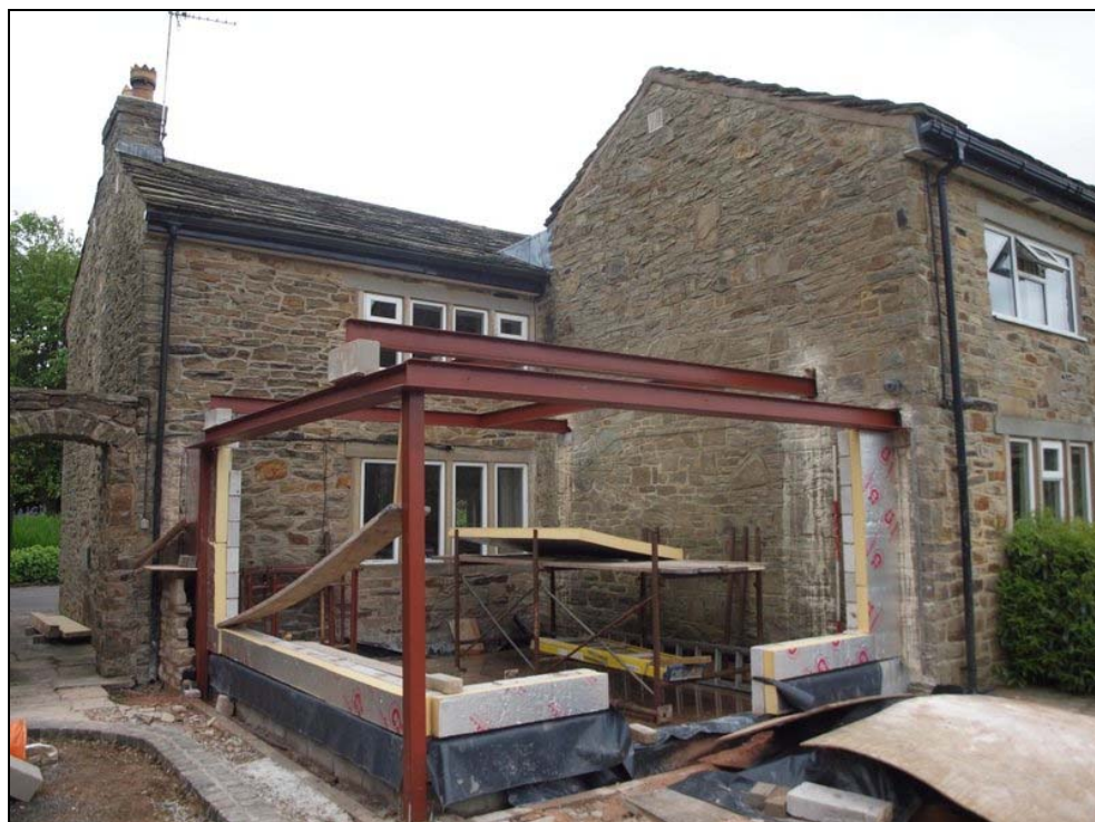
Plate 1/8: Corner of building where openings were to be inserted
