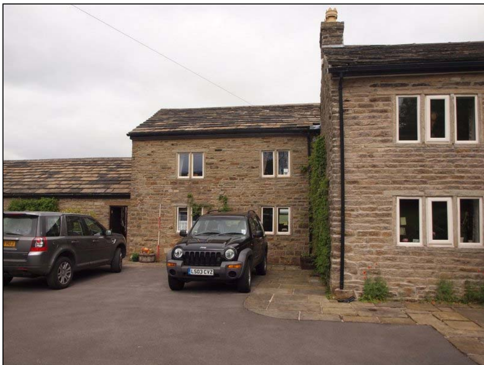
Plate 17/3: Front (south) side of the building, centre
