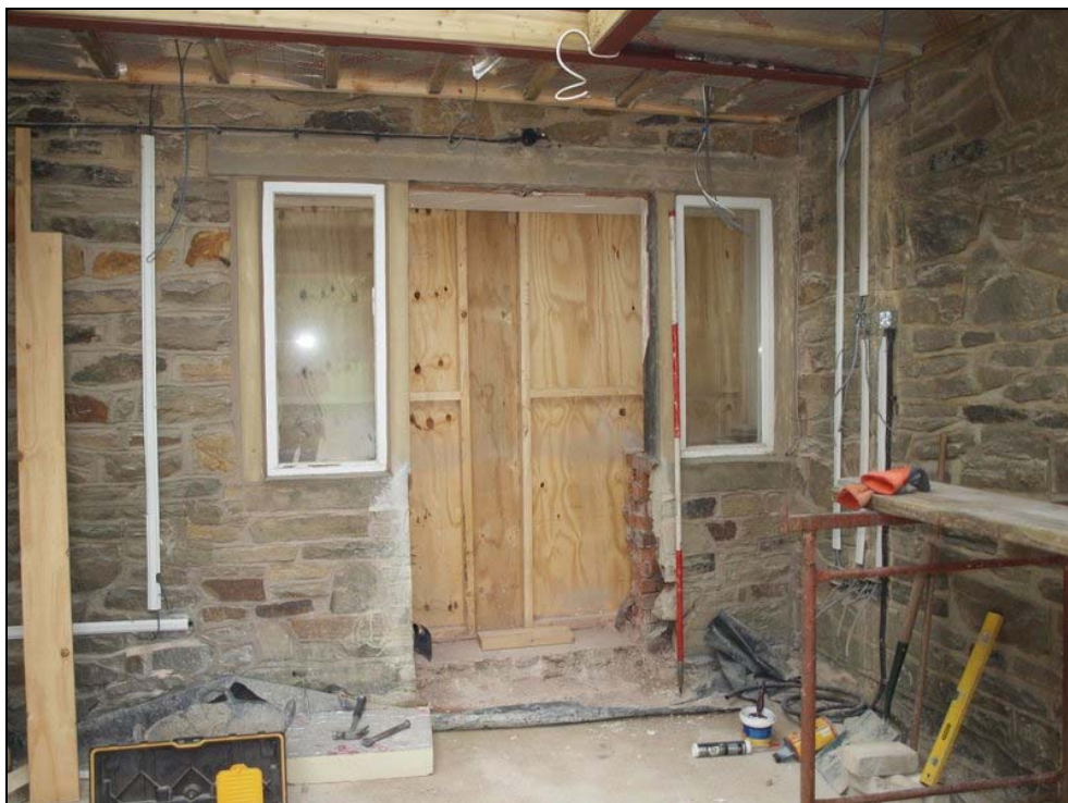
Plate 6/9: Opening inserted in window
