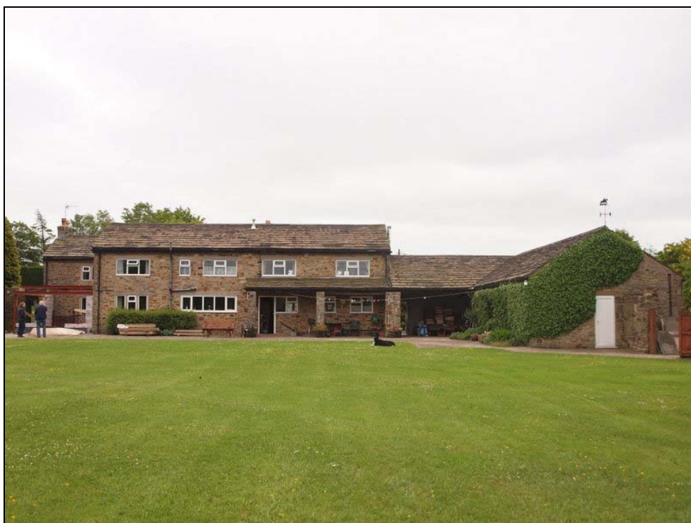
Plate 13/4: Whole north side of the building
