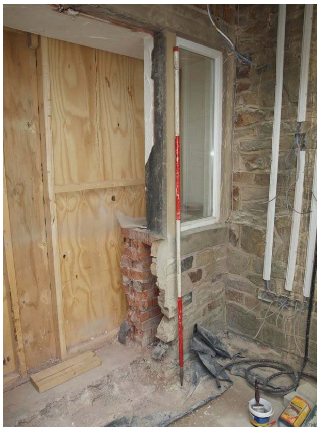
Plate 7/10: Opening in window showing cavity wall with stone & brick skins
