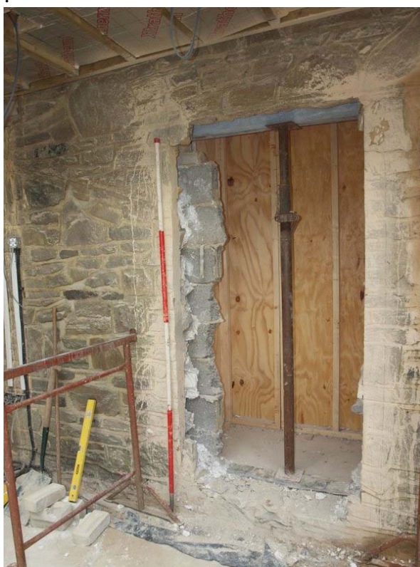
Plate 8/12: Opening inserted in gable wall
