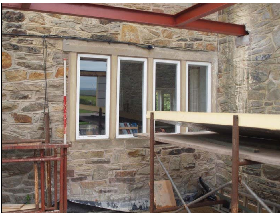
Plate 2/6: Detail of window to have doorway inserted
