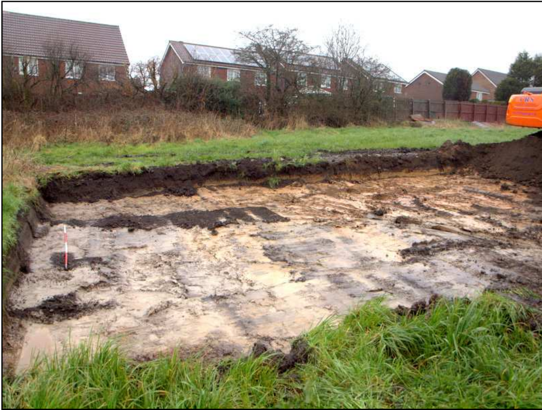
Plate B9: Open area excavation viewed from the south
