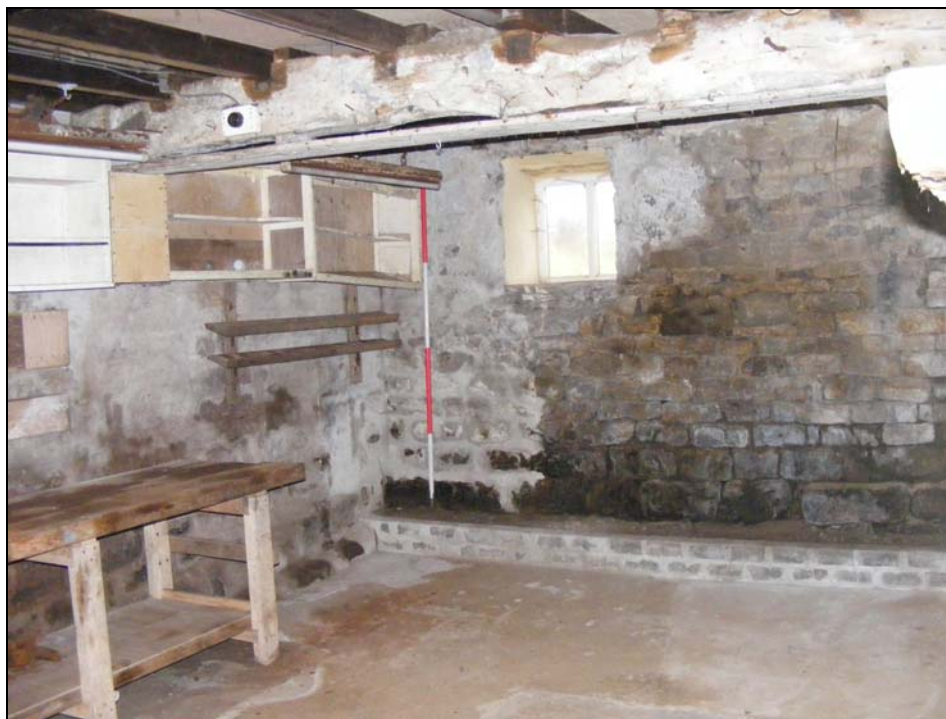
Plate 7: Ground floor of cottage
