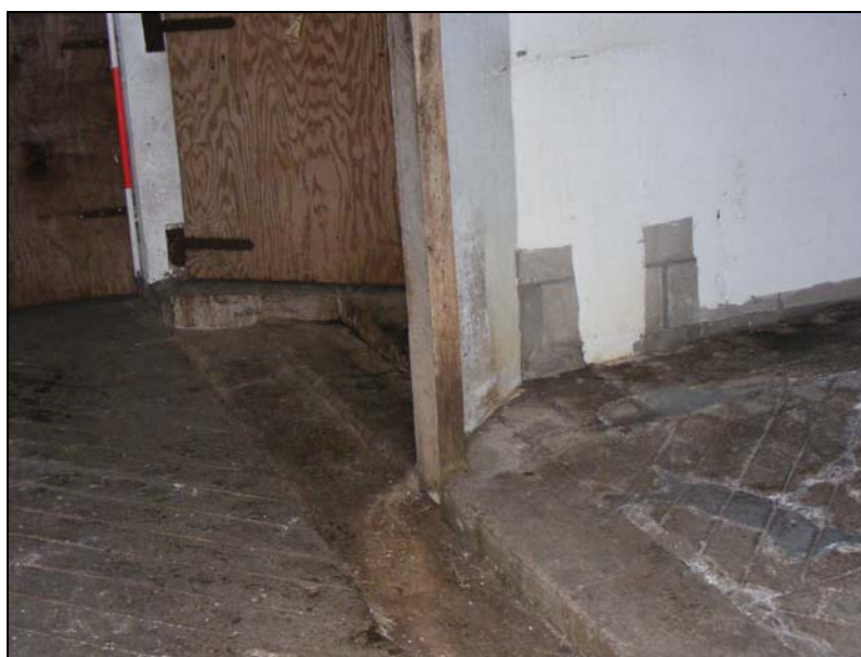
Plate 20: Floor of former shippon in ground floor of barn
