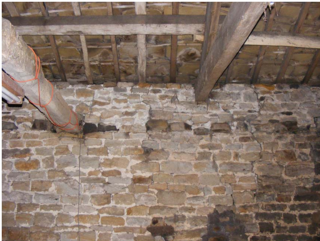
Plate 23: Raised south elevation of barn
