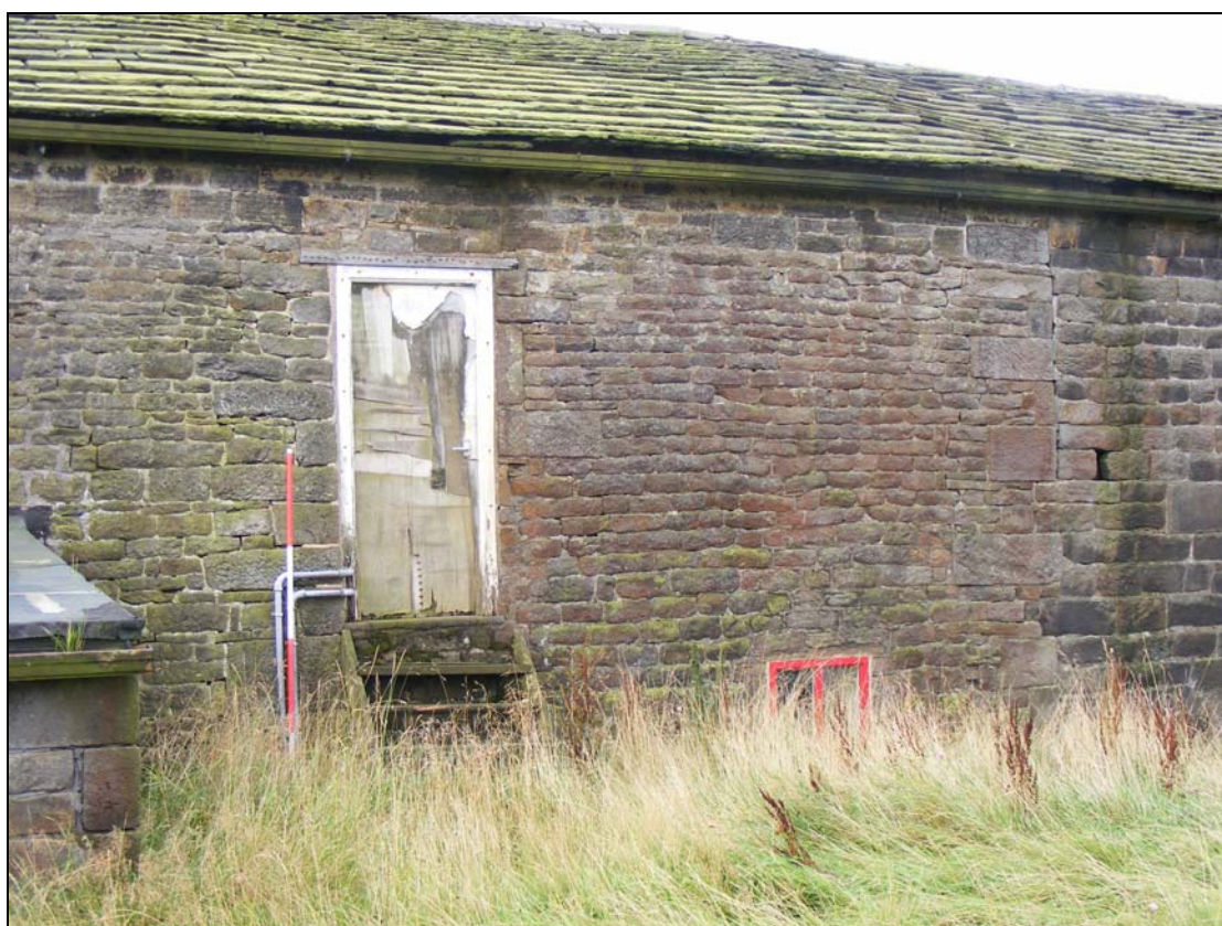
Plate 6: North elevation of cottage
