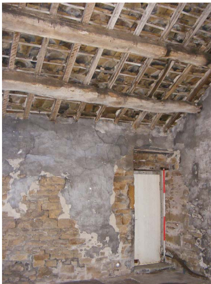
Plate 11: Doorway in northeast corner of first floor of cottage
