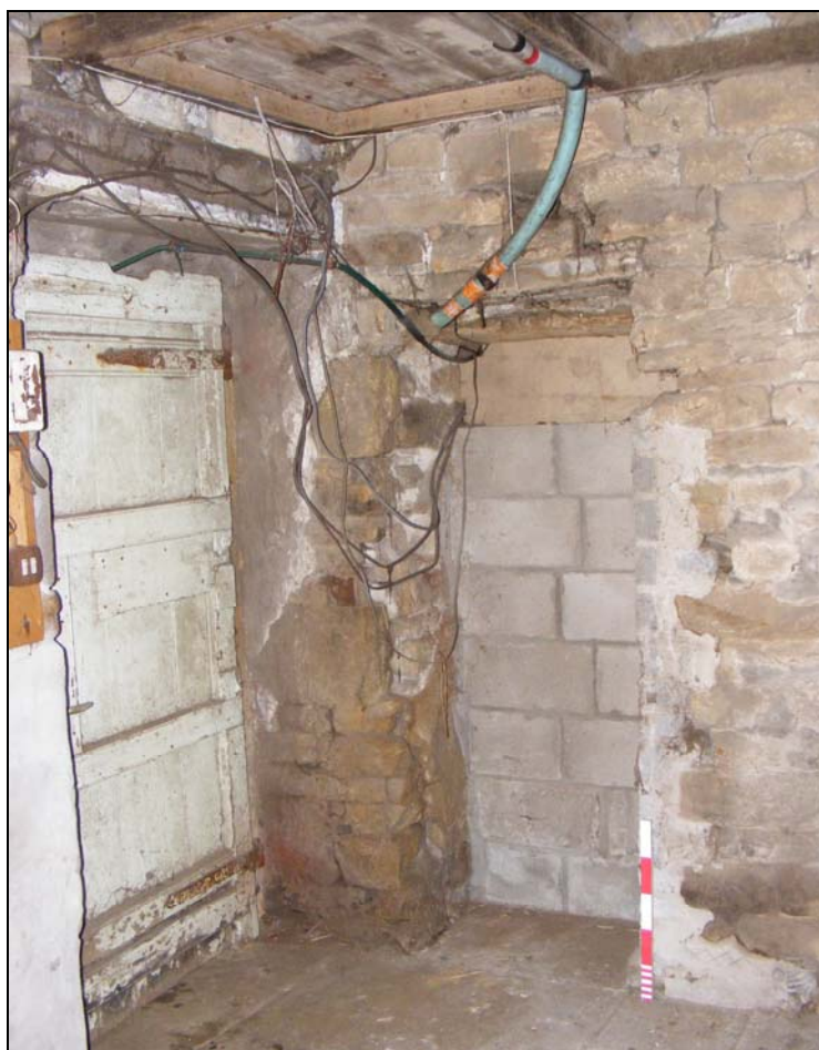
Plate 8: Doorway in northeast corner of first floor of cottage
