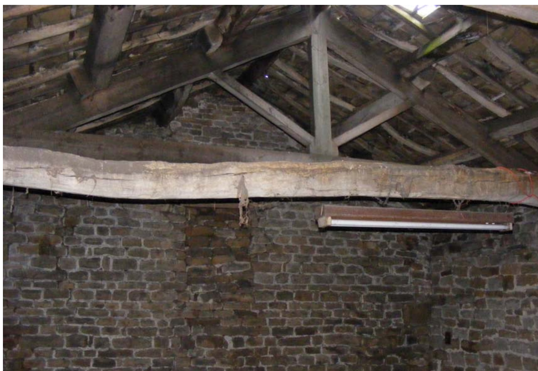
Plate 22: Queen-post roof truss and hand-cut roof-tie
