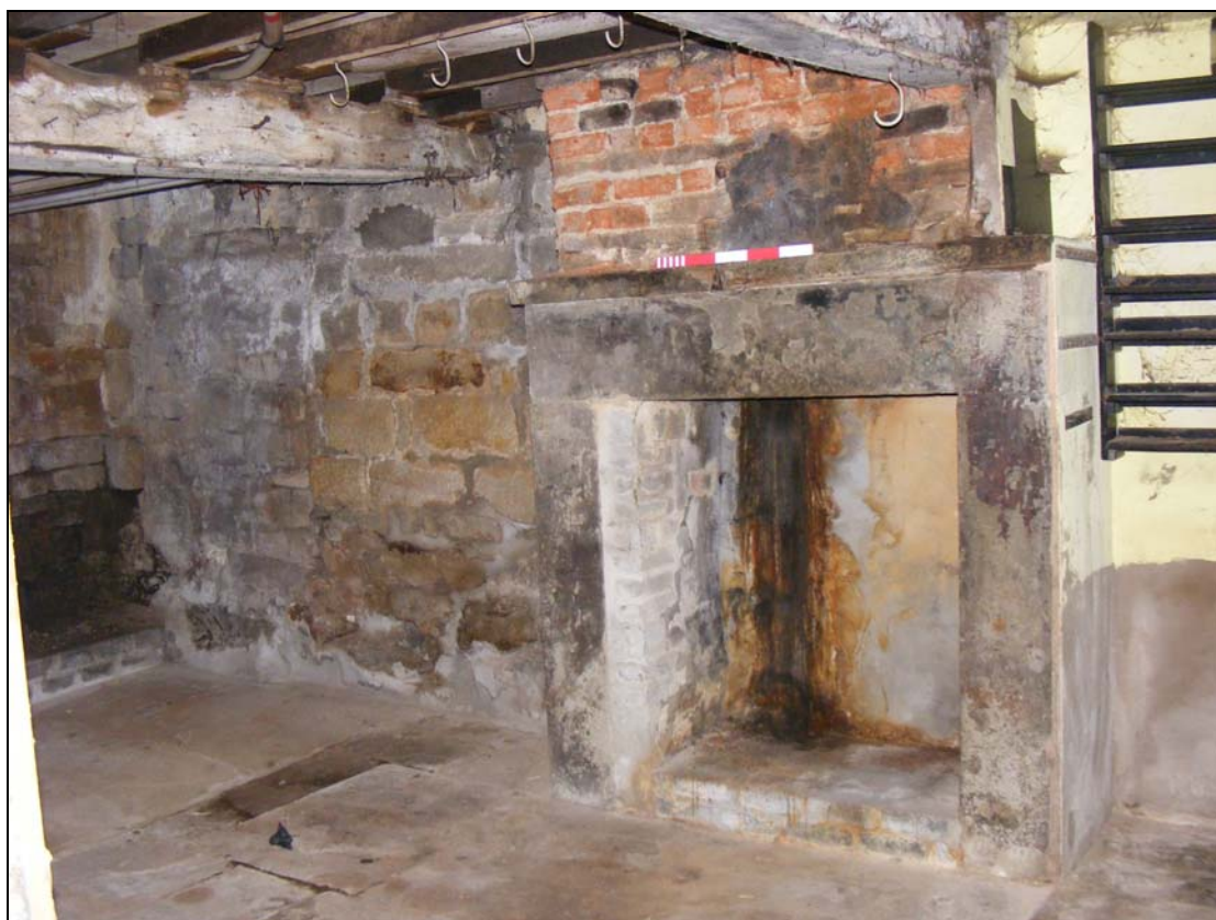
Plate 10: Ground floor of cottage
