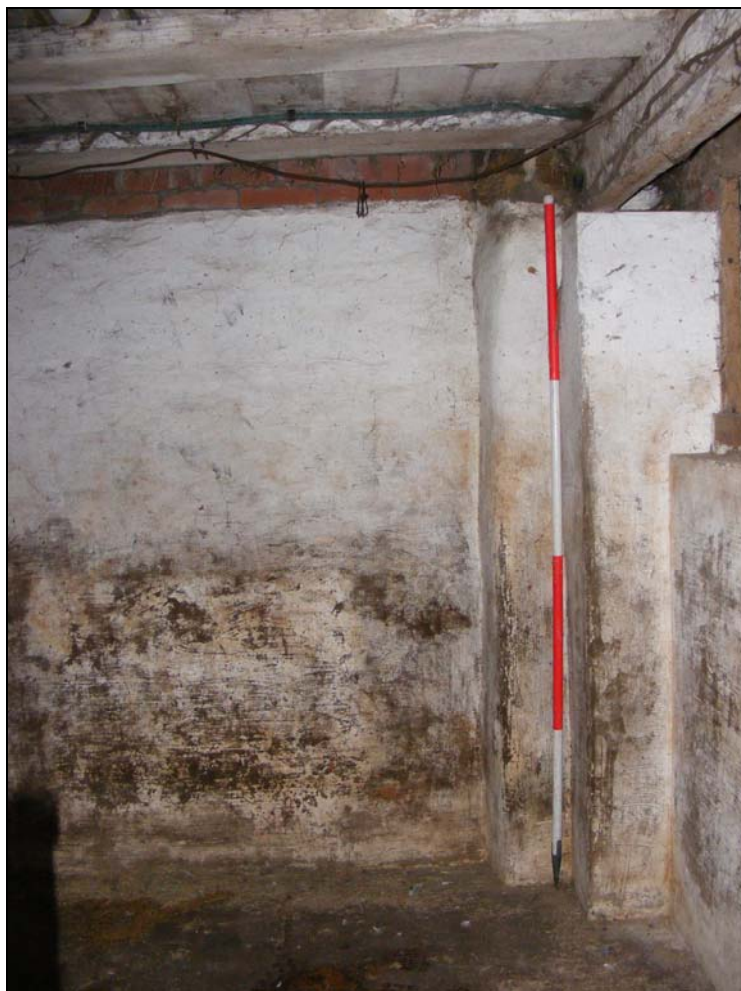
Plate 19: Stub of former wall in ground floor of barn
