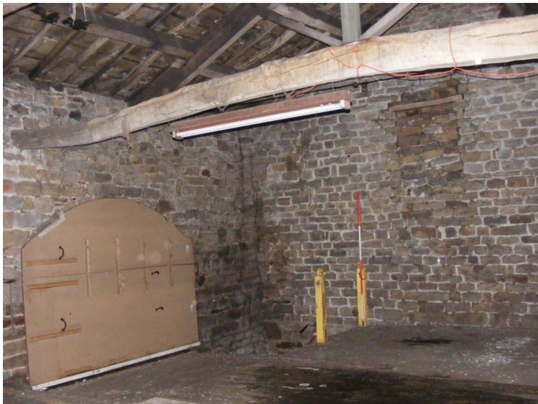
Plate 21: First floor of barn showing stairwell and north barn door
