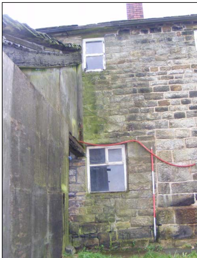
Plate 3: South elevation of cottage
