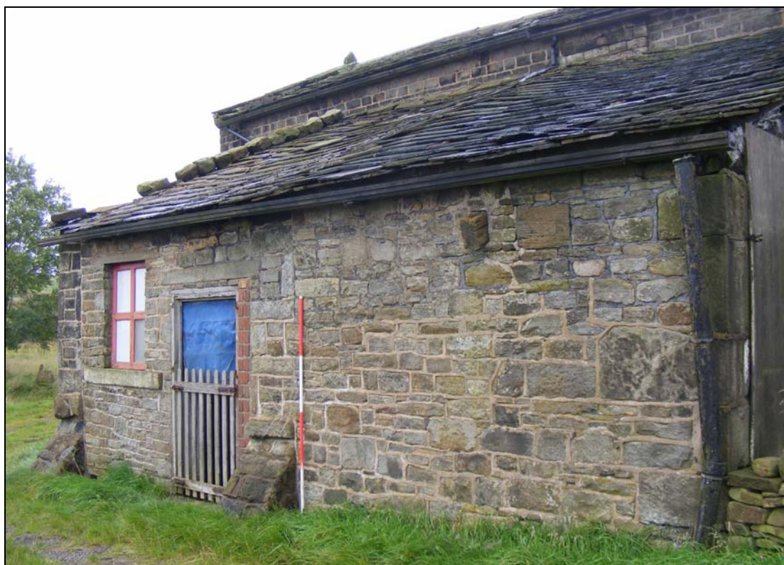
Plate 25: South elevation of southern outrigger
