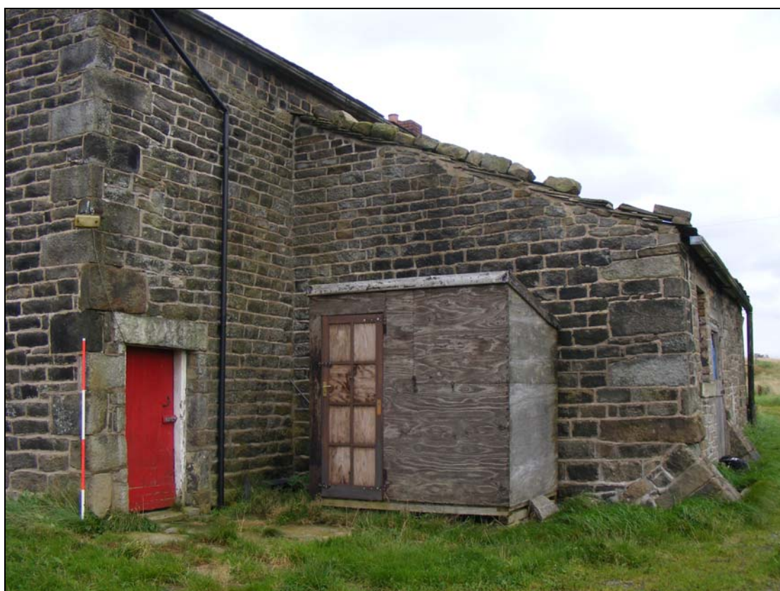
Plate 14: South elevation of barn and west elevation of southern outrigger
