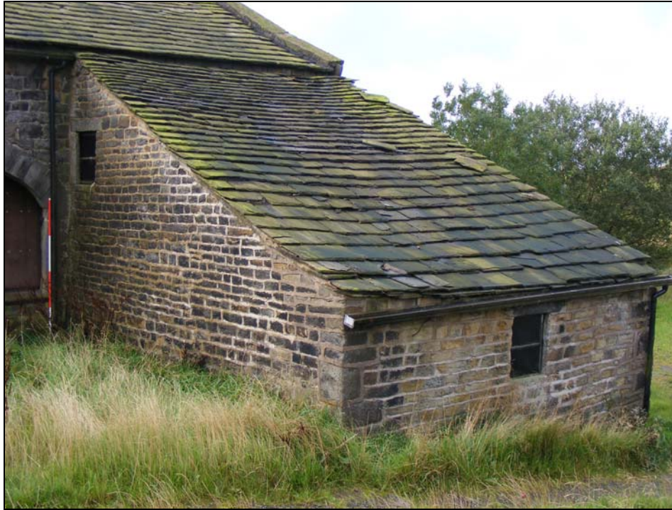
Plate 27: North and east elevations of northern outrigger
