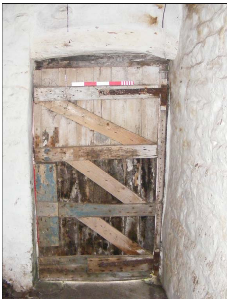
Plate 18: Door in south elevation of barn
