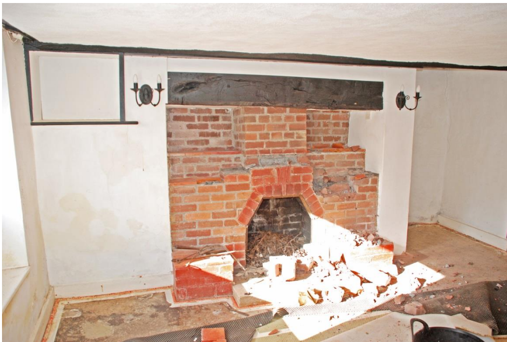
Fig. 9 The kitchen fireplace with modern brick infilling beneath old timber lintel.
