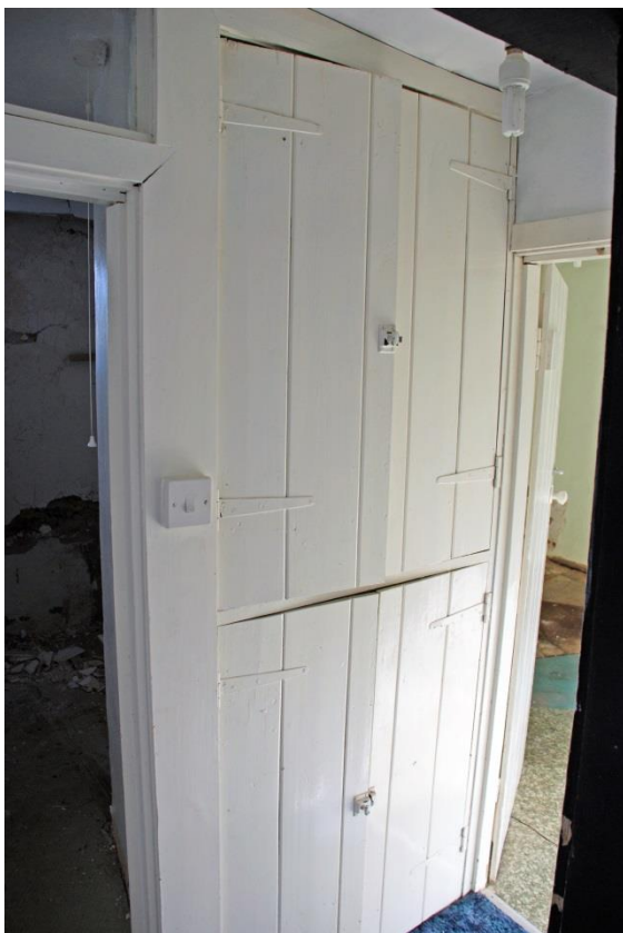
Fig. 15 The airing cupboard doors.
