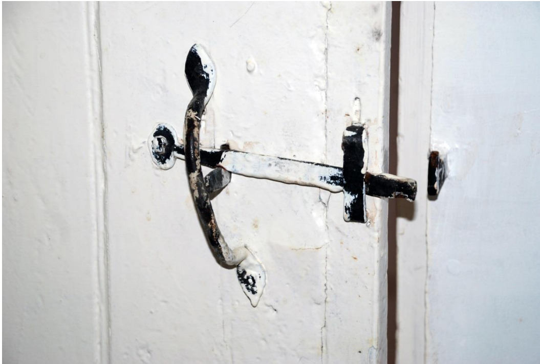
Fig. 4 18th-century handle and lifting bar latch on inside of door into central service room.
