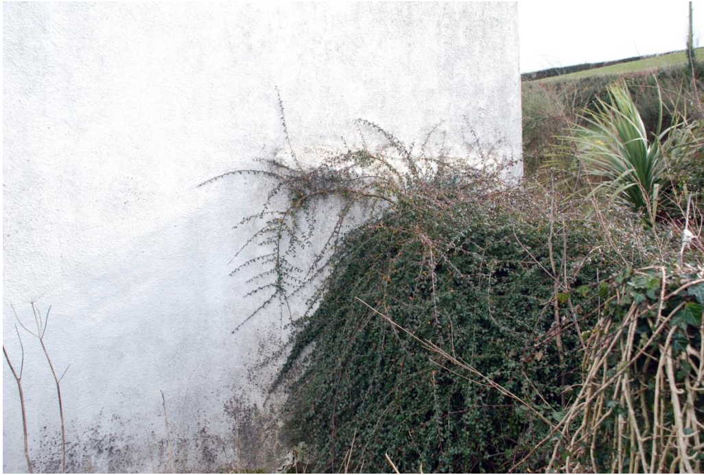
Fig. 11 The external ground-floor round projection for an oven next to the kitchen fireplace.
