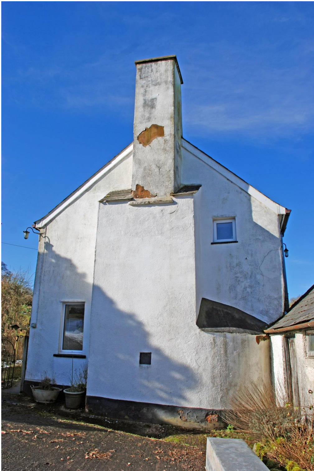
Fig. 10 The east gable end of the house showing round ground-floor projection for oven next to the parlour fireplace.
