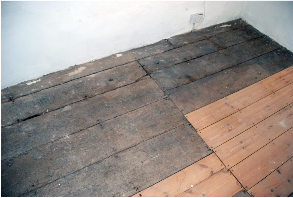
Fig. 14 Old floor boards in the middle bedroom.
